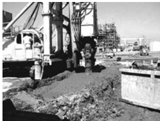
Photo 3.13 TRD operation at Alamitos Gap, California.
