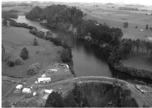
Photo 4.22 Arapuni Dam, New Zealand. (From Amos, P. D., D. A. Bruce, M. Lucchi, N. Watkins, and N. Wharmby, “Design and Construction of Deep Secant Pile Seepage Cutoff Walls Under the Arapuni Dam in New Zealand,” USSD 2008 Conference , Portland, OR, 2008. With permission.)
