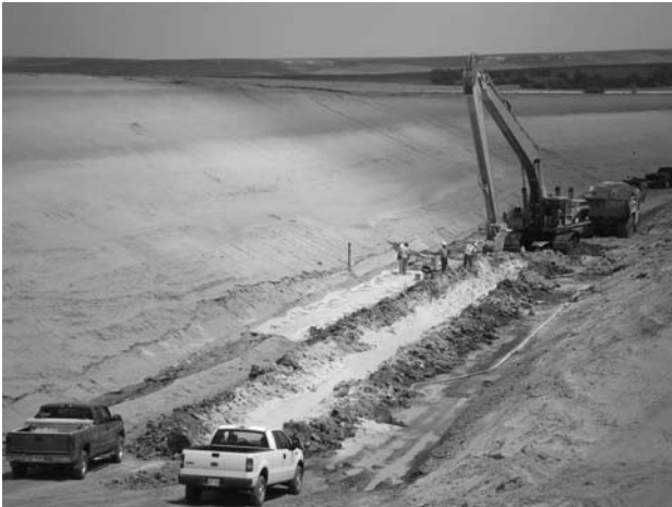
Photo 4.3 Excavation for CB cutoff, Horsethief Dam, Kansas.
