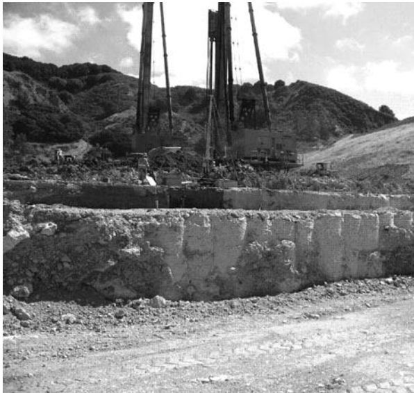
Photo 3.10 Exposed soil-cement shear wall at San Pablo Dam, California.
