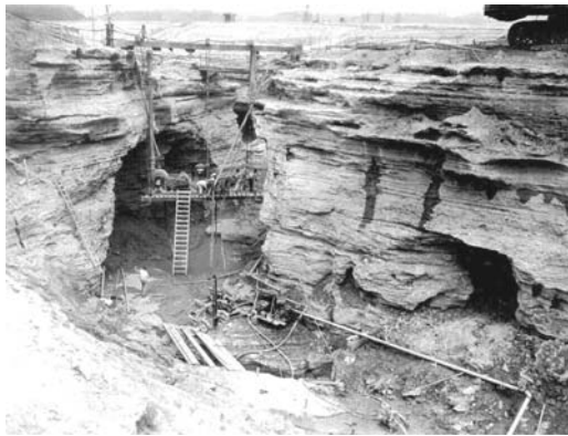
Photo 2.7 Photo of the system of caves uncovered during excavation of the dam foundation, Wolf Creek Dam, Kentucky. (Courtesy of U.S. Army Corps of Engineers.)
