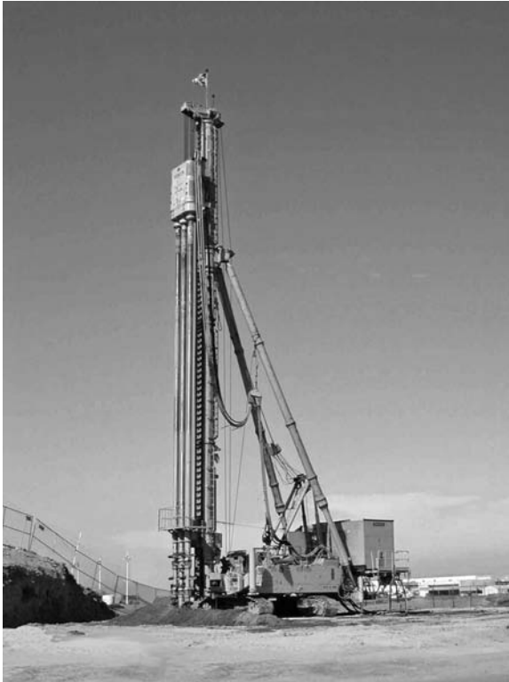
Photo 3.4 DMM triple axis rig (WRE). (Courtesy of Raito, Inc.)
