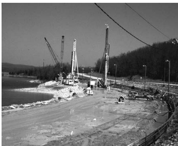
Photo 4.16 Secant pile operations at Beaver Dam, Arkansas. (Courtesy of Rodio-Nicholson JV.)
