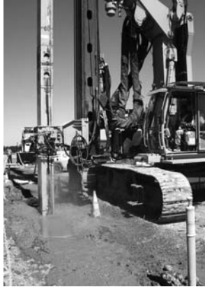
Photo 3.16 Kelly (square) guided CSM unit for depths up to 140 feet.
