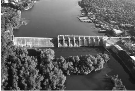
Photo 6.2 Aerial view of Tom Miller Dam, Texas. (Courtesy of Lower Colorado River Authority archives.)
