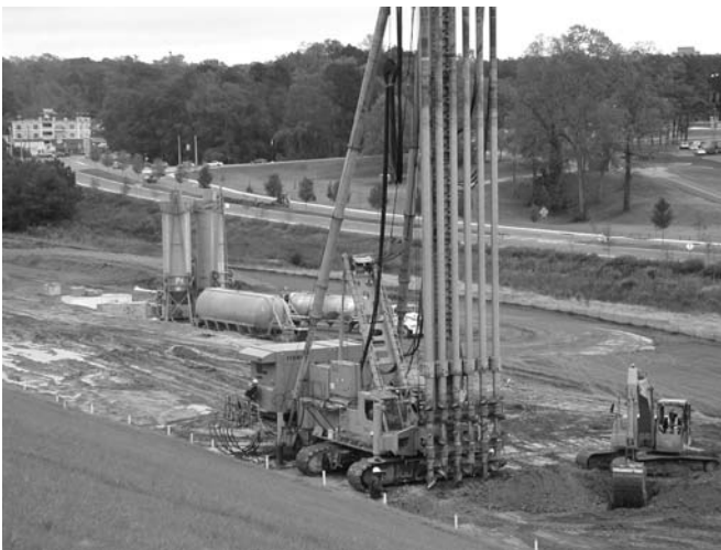
Photo 3.7 Six-axis DMM Rig at Clemson Dam, South Carolina. (Courtesy of Ratio, Inc.)
