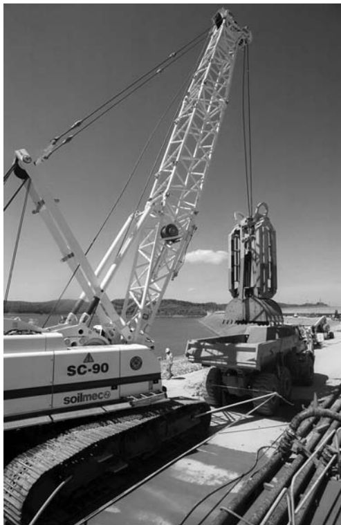
Photo 4.4 Cable-suspended and activated clamshell. (Courtesy of TREVIICOS Corp.)
