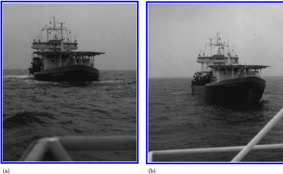
Figure 3.10 Hydraulic deposition of sand into berm (see Figure 1.20). About 5000 m 3 sand was deposited by bottom-valve discharge through water in 10 min between photo on left and photo on right. (a) With hoppers full and (b) after discharging load.
