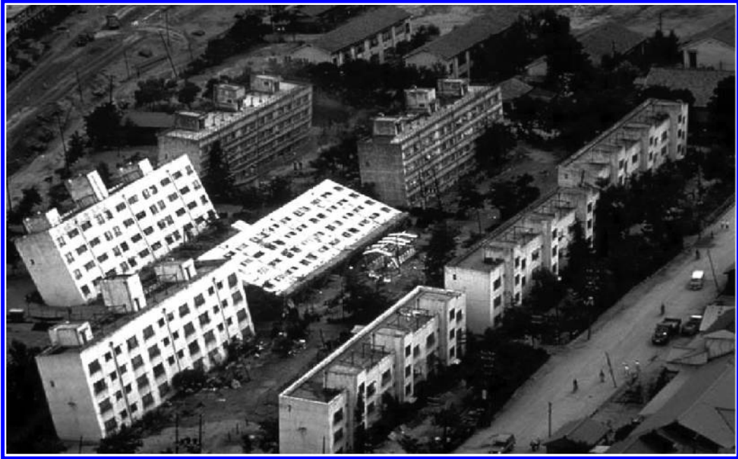
Figure 1.8 Apartment building at Kawagishi-cho that rotated and settled because of foundation liquefaction in 1964 Niigata earthquake. (From Karl V. Steinbrugge Collection, Earthquake Engineering Research Center, University of California, Berkeley, CA.)
