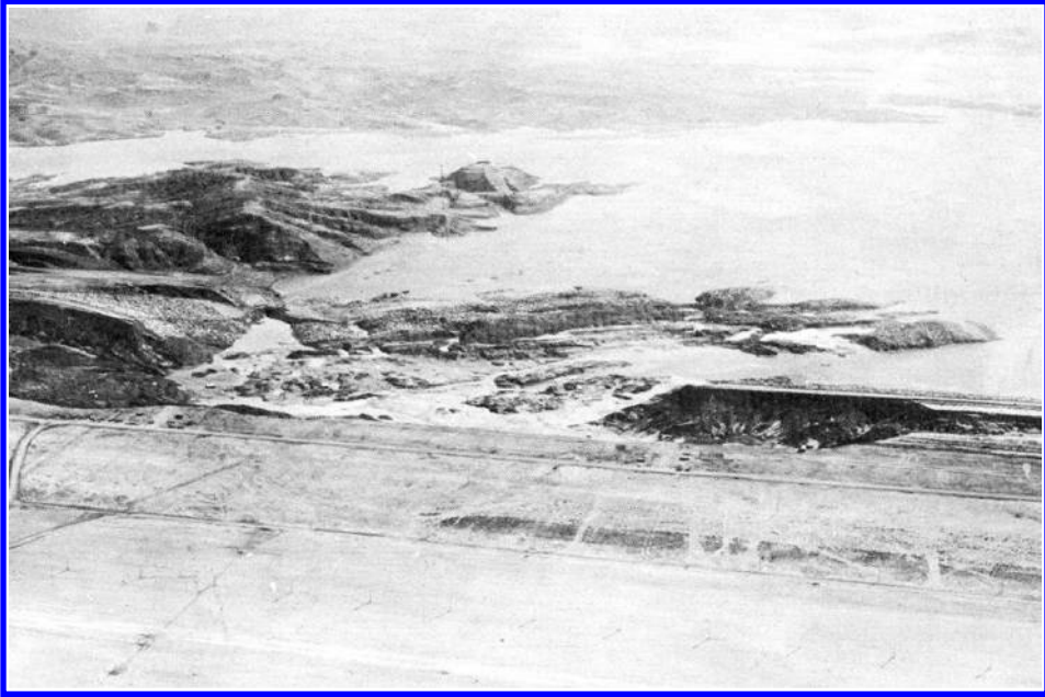
Figure 1.2 Aerial view of Fort Peck failure. (From U.S. Army Corp of Engineers, Report on the slide of a portion of the upstream face at Fort Dam. US Government Printing Office, Washington, DC, 1939.)
