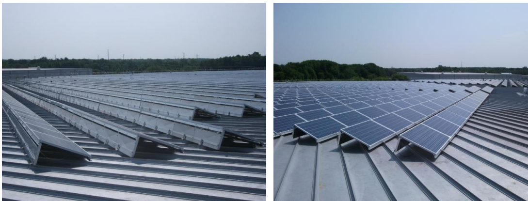
Fig. 1-2. Typical Tilted-Closed Solar Panels (Photos courtesy of MBMA)
