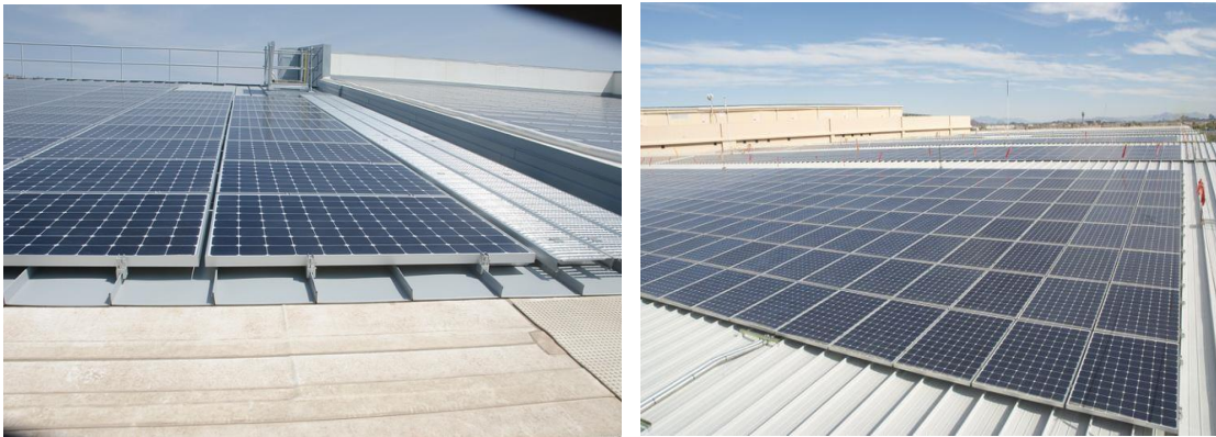
Fig. 1-1. Typical Flush Solar Panels (Photos courtesy of MBMA)
