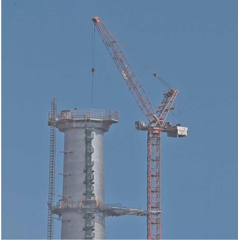
Figure 7.16 One of the pylons of Stonecutters Bridge during construction
