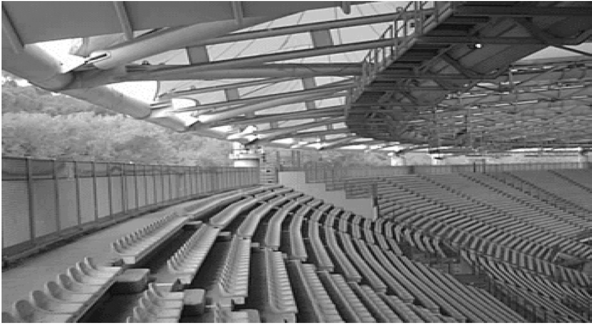
Figure 8.6 Roof structure of the Rome Stadium
