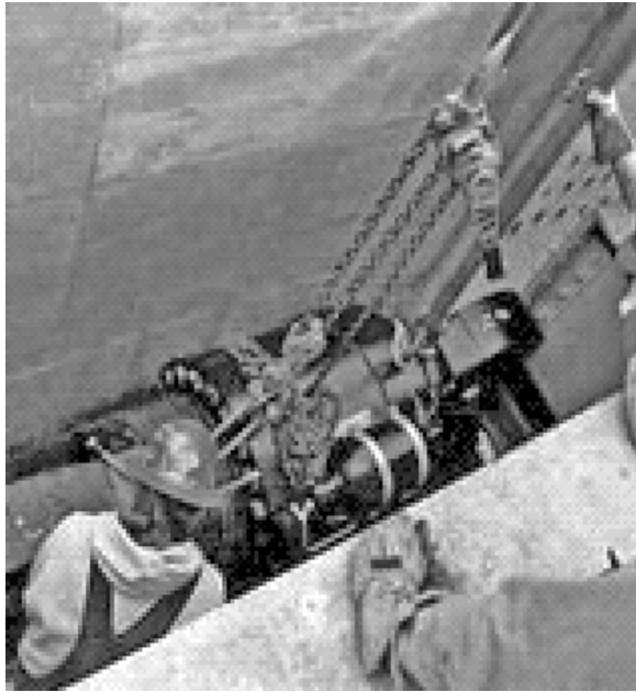
Figure 11.11 The STU is positioned to align with the brackets for connection
