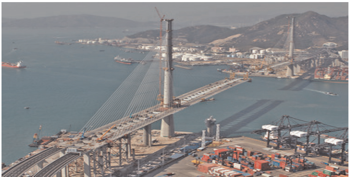
Figure 7.15 Stonecutters Bridge spanning the Rambler Channel, Hong Kong
