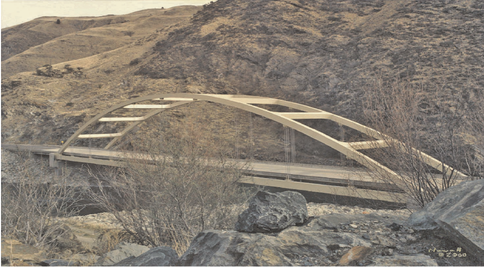
Figure 4.7 Goff Bridge, Riggins, Idaho, USA
