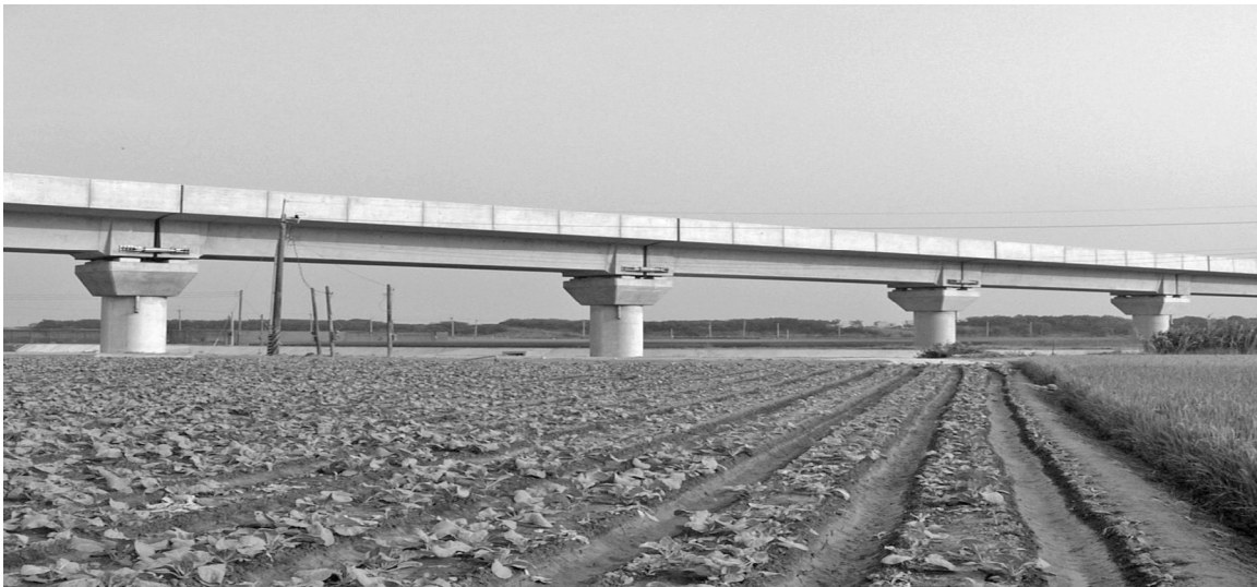
Figure 6.2 Taiwan High Speed Rail viaduct with STUs at the expansion joints
