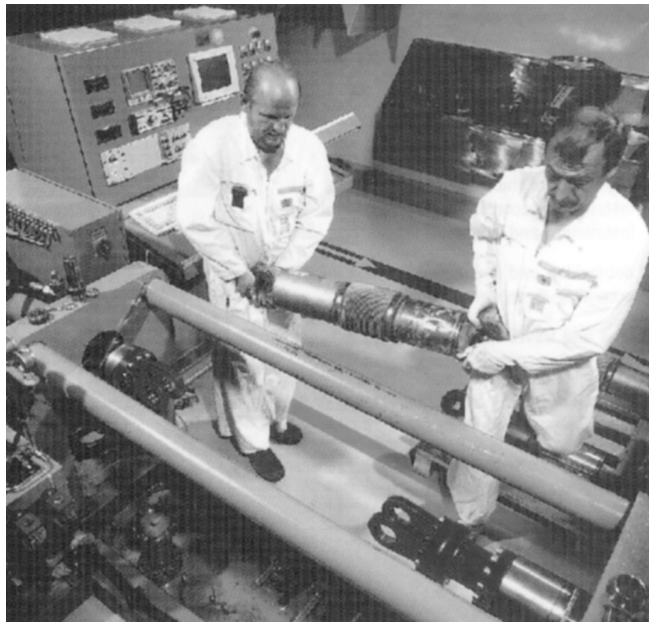
Figure 9.10 In-service testing of installed snubbers
