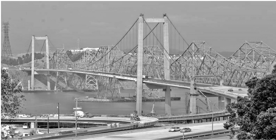
Figure 5.3 The new suspension bridge and the two older Carquinez crossings
