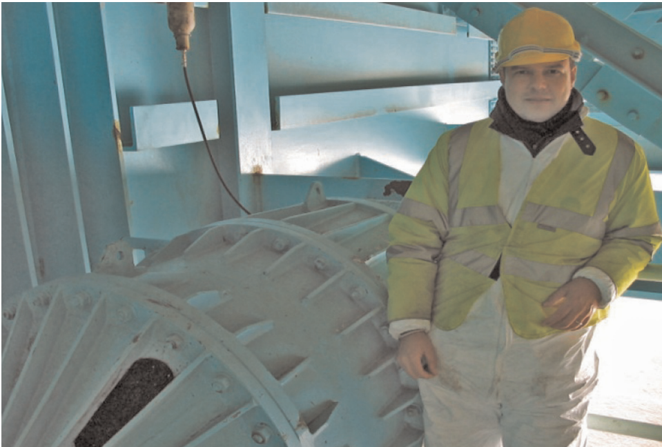
Figure 7.9 STUs in place on the Second Severn Bridge
