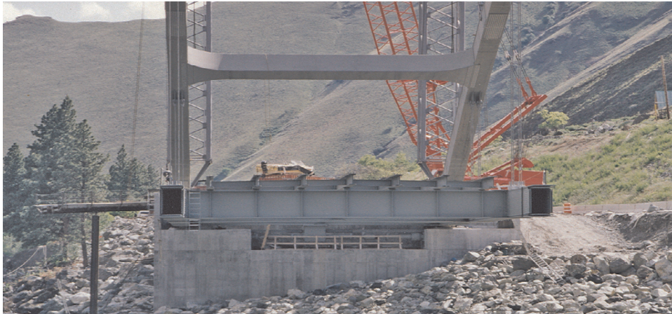
Figure 4.9 The extra-wide abutment of the Goff Bridge
