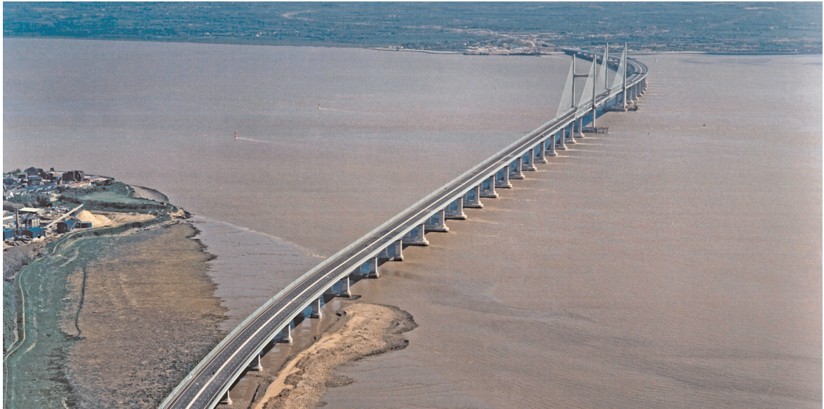
Figure 7.6 The Second Severn Bridge. Reproduced courtesy of FIP Industriale SpA
