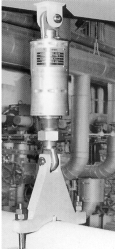
Figure 9.15 Snubber connection to a pipe in a nuclear power plant to control movement of the pipe in the vertical direction
