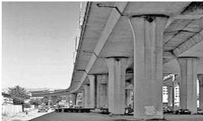
Figure 5.9 Structural elements of the Arthur Laing Bridge
