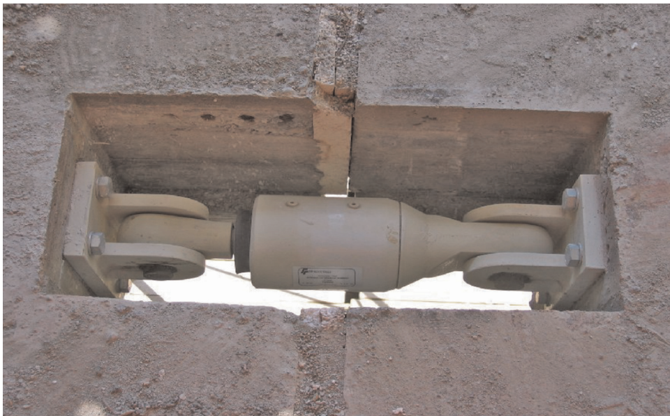
Figure 8.2 An STU installed in the multi-bay building at Udine shown in Figure 8.1
