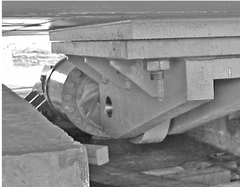
Figure 11.5 Installation of STUs on the Second Bassein Creek Bridge
