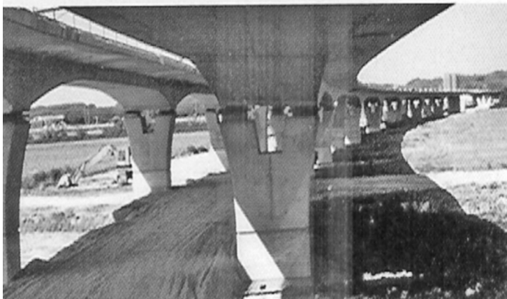
Figure 17.4 The Mortaiolo Viaduct. Courtesy of Agostino Marioni, Alga
