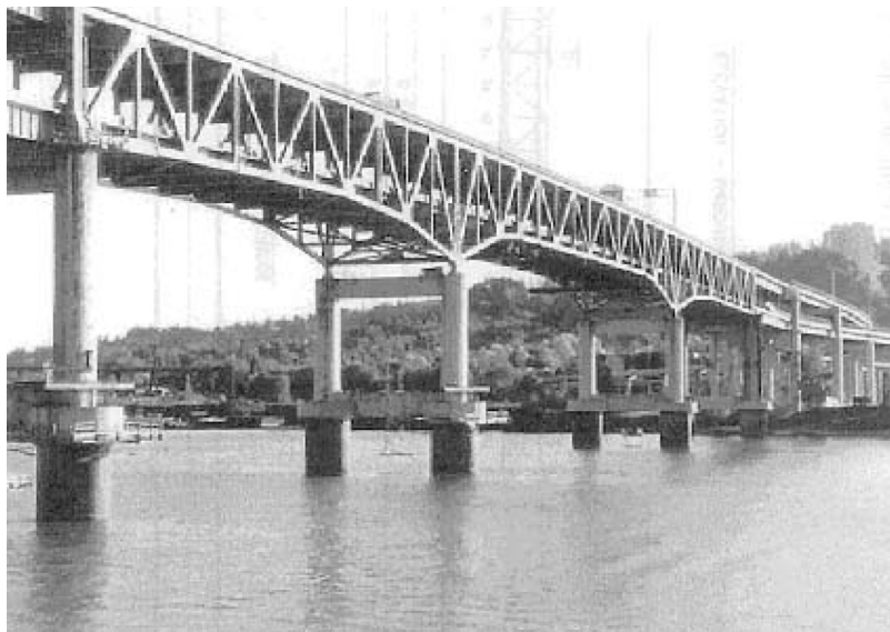
Figure 17.15 The Marquam Bridge. Image courtesy of the Oregon Department of Transportation
