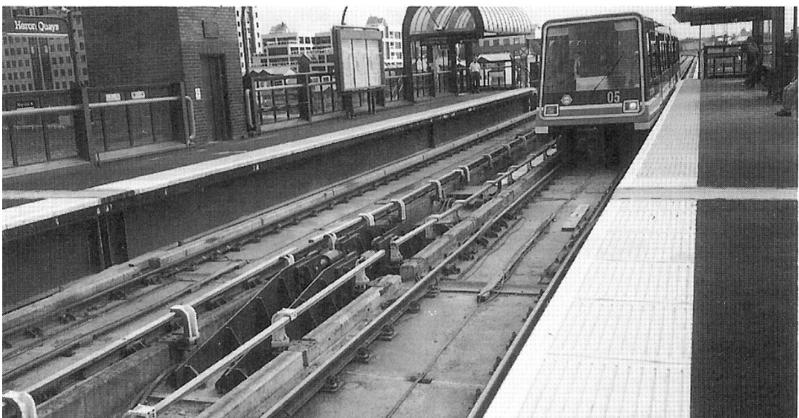
Figure 6.11 The DLR in operation with added trains after installation of STUs
