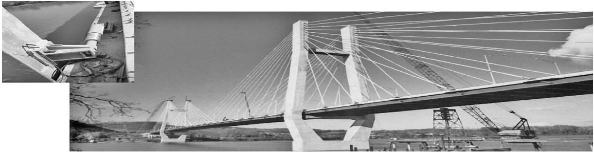
Figure 12.2 The Maysville cable-stayed bridge
