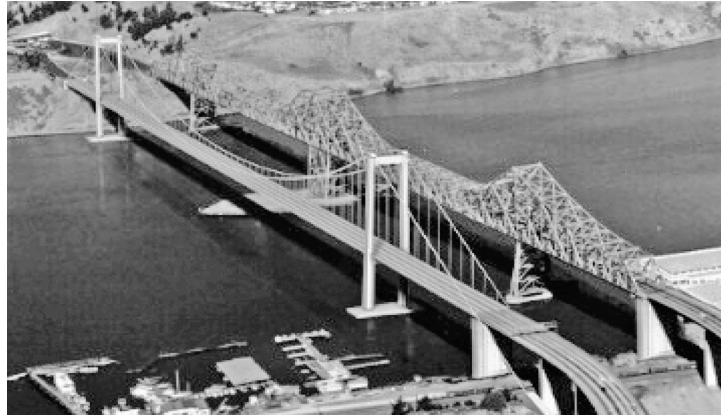
Figure 5.4 The new suspension bridge and retrofitted 1958 steel truss bridge after demolition of the 1927 bridge at Carquinez
