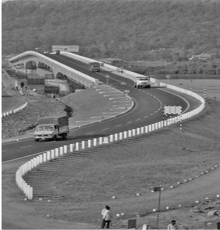
Figure 4.4 The completed Second Bassein Creek Bridge
