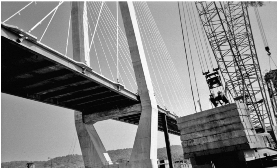
Figure 7.10 The Maysville Bridge
