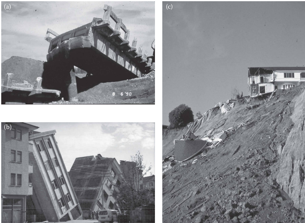
Figure 4.2 Examples of poorly sited structures. (a) Fault Rupture – Luzon, Philippines 1990. (b) Liquefaction – Adapazari, Turkey 1999. (c) Slope Instability – Pacific Palisades, Los Angeles, 1994.
