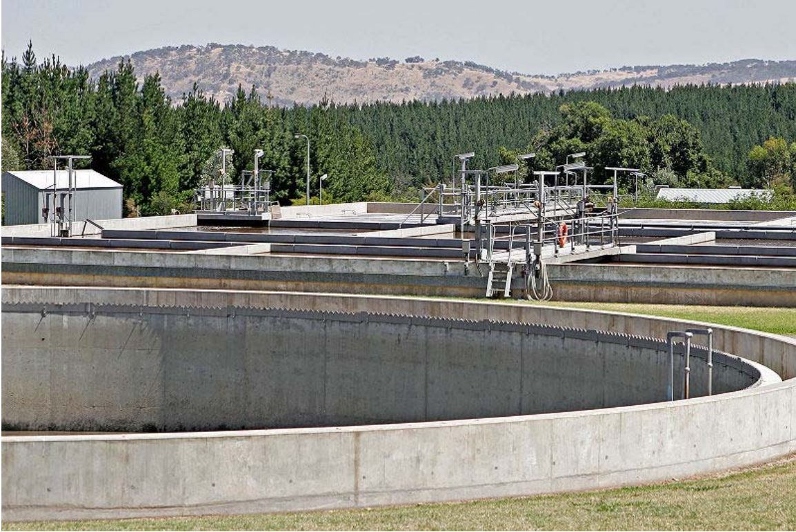
Sewage treatment plant, Australia.
