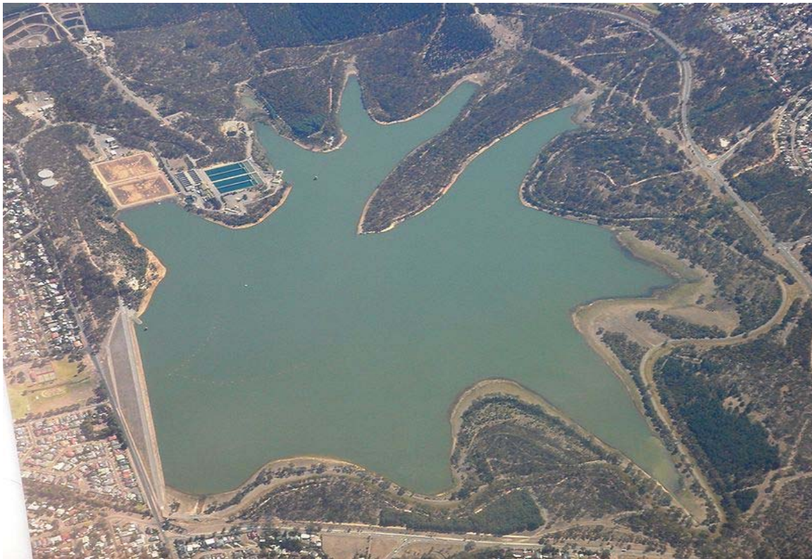
The Happy Valley Reservoir stores water for supply to Adelaide.
