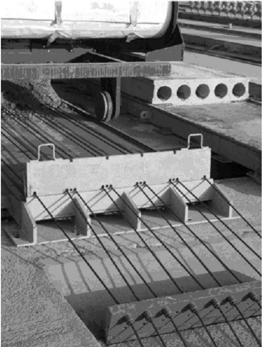
Fig. 2.2b Placing concrete after pre-tensioning the cables
