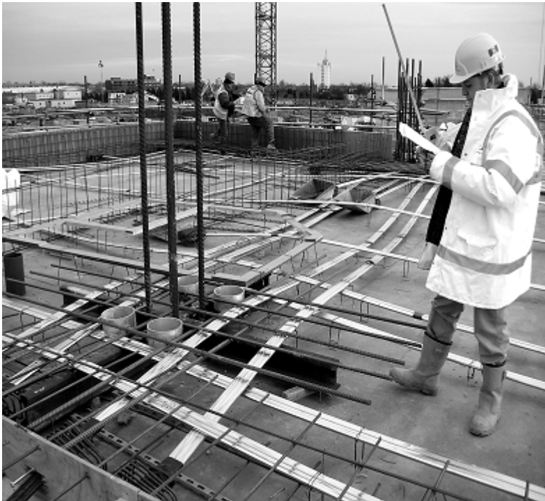
Fig. 12.89 Fully banded layout of tendons Photo Courtesy VSL
