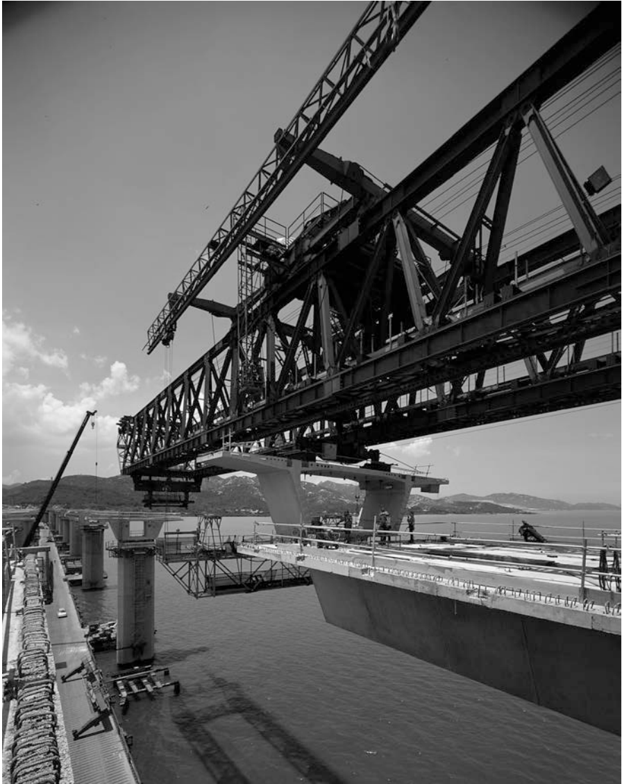
Fig. 16.6 Erection of an additional unit (Photo: Courtesy of CCL)
