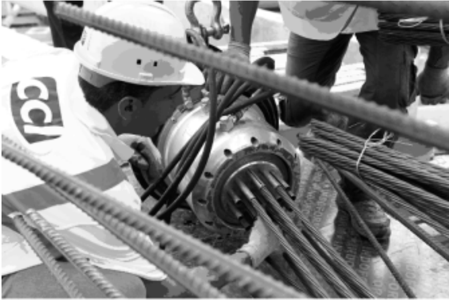
Fig. 2.19 Stressing the cable Photo Courtesy CCL
