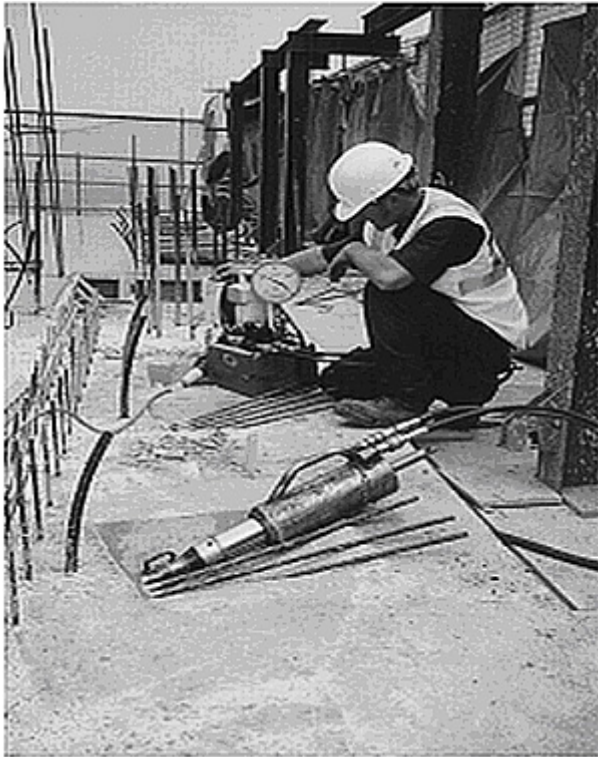
Fig. 12.91 Stressing the cables Photo Courtesy VSL
