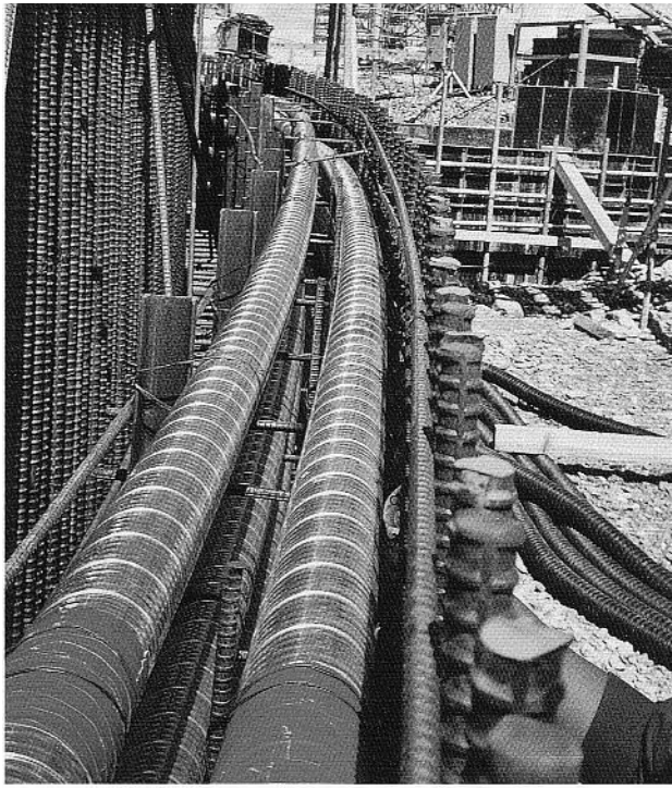
Fig. 2.13 Ducts fixed to reinforcement Photo courtesy DYWIDAG Systems International
