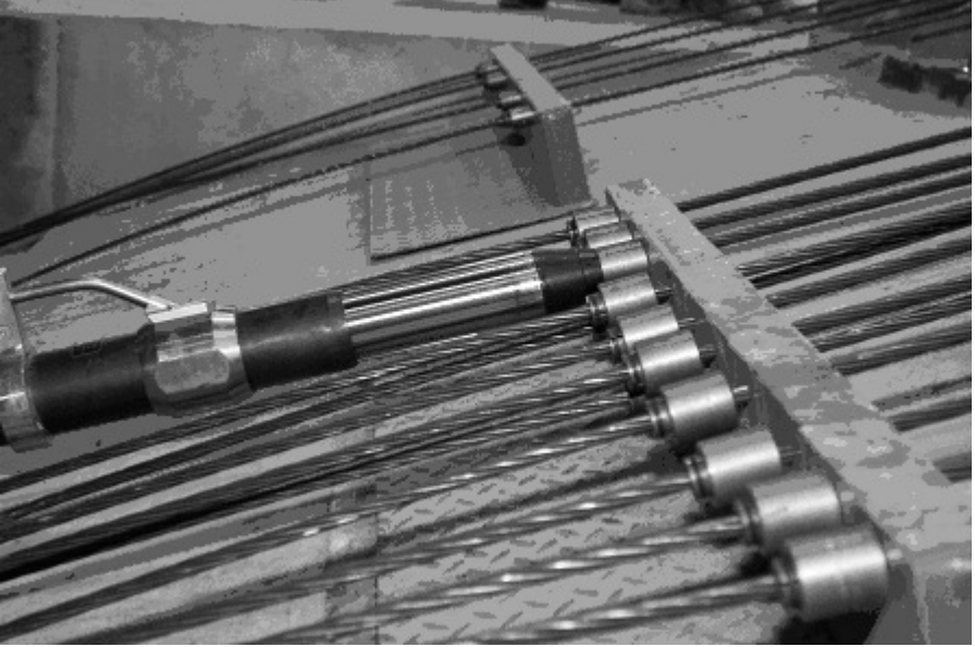
Fig. 2.2c Close-up of anchors and stressing of a cable
