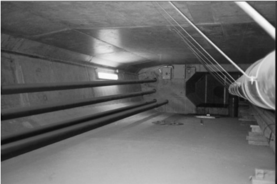
Fig. 2.22b 'External' tendons in a box girder
