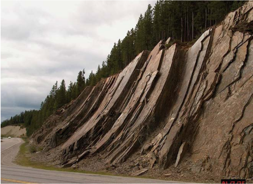
Figure 1.4 Cut face coincident with continuous, low-friction bedding planes in shale (Trans Canada Highway near Lake Louise, Alberta). (Image by A. J. Morris.)
