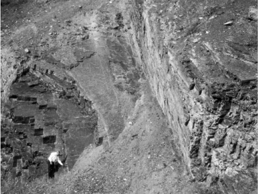
Figure 8.2 Wedge formed by bedding (left) and a conjugate joint set (right); sliding occurred on bedding with joints acting as a release surface (bedded shale, near Helena, Montana).
