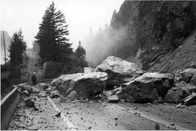
Figure 14.1 Highway closure caused by rock fall in very strong, blocky granite from a height of about 300 m.
