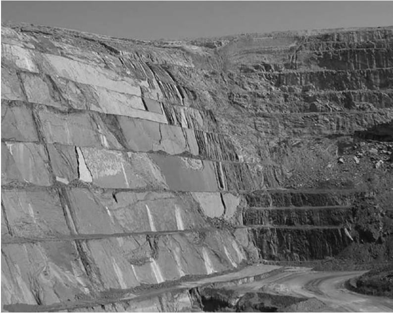
Figure 12.4 Anisotropic rock mass – shale (from Sainsbury et al., 2008).
