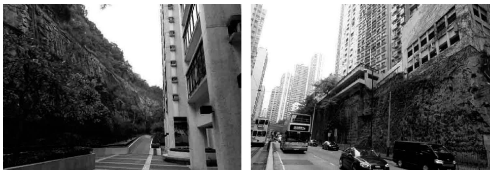
Figure 2 Typical rock cut slopes in the urban setting of Hong Kong.
