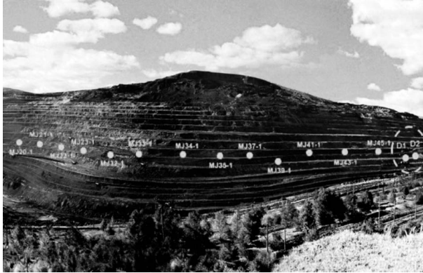
Figure 15 Monitored area in Pingzhuang open pit coal mine: A photograph showing the monitored points on the slope.
