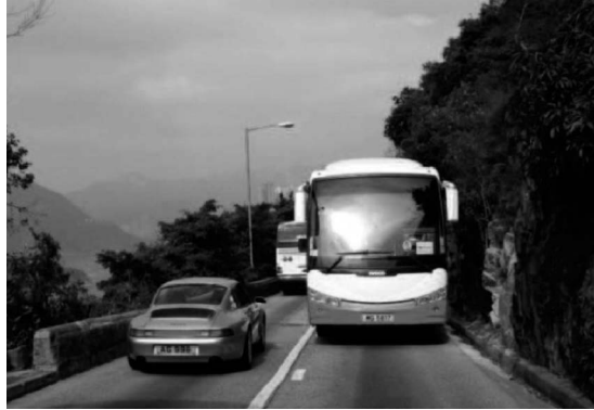
Figure 13 Typical rock cut slope abutting narrow and busy road (Ho & Wright, 2011).
