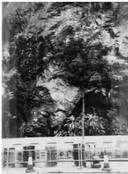
Figure 18 The 1998 A Kung Ngam Road rockfall.
