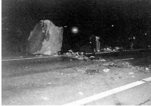
Figure 23 The 1995 Tuen Mun Highway rockfall.
