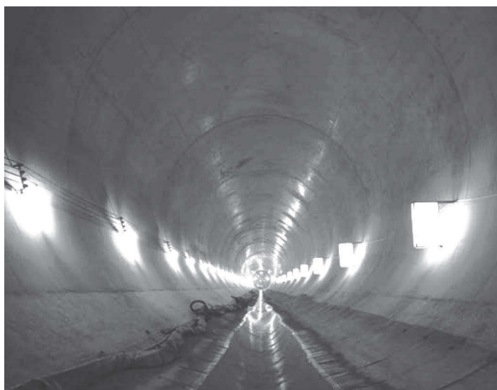
Figure 16 Diversion tunnel face before operation.
