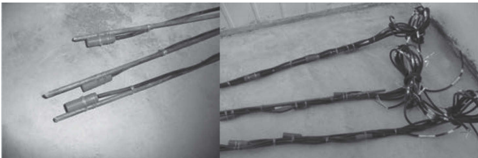
Figure 21 The field installation of temperature sensors assemblies.
