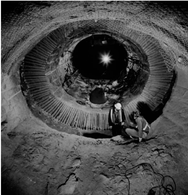
Figure 18 Test chamber for the Tunnel Sealing Experiment, showing the clay-bulkhead key (rectangular cross-section).
