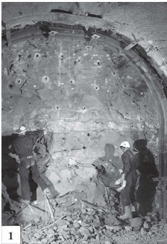
Figure 10 View of the front face during drift excavation at -445 m (b) resin injected borehole showing no fracture at the side wall and fracture near the wall at the floor.
