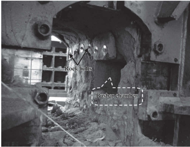
Figure 27 Failure pattern of the main power house under an overburden depth of 1800 m.
