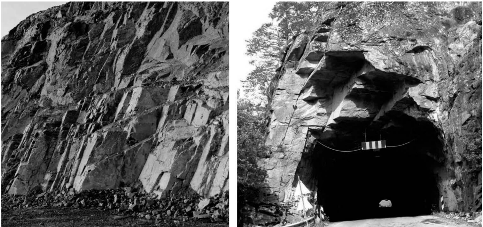
Figure 1 Characteristics of joint sets as observed in a Finnish open pit and at the portal of an old unsupported road tunnel in Norway (100 years prior to Q-system tunnel support guidance). We see variable orientation (dip and dip direction), variable spacing within each set, variable numbers of joint sets (two to three), variable block shape and size, and variable joint continuity (e.g. 1–10m and discontinuous).
