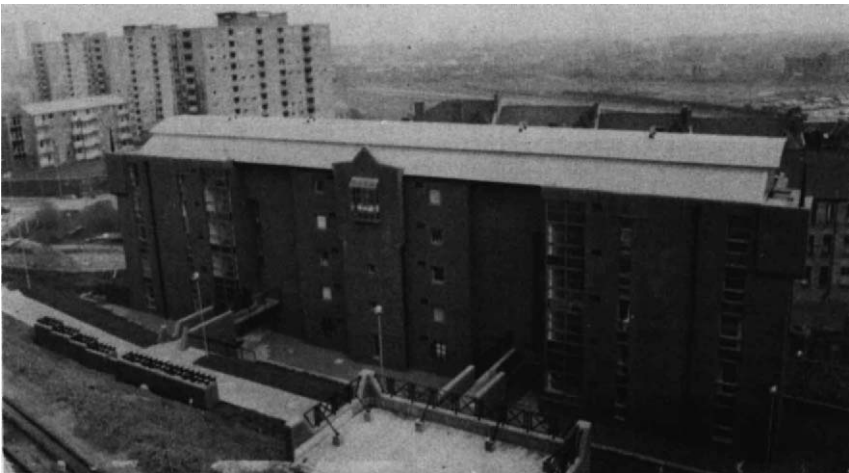
Figure 2: Rear view, low glazing area and open aspects
