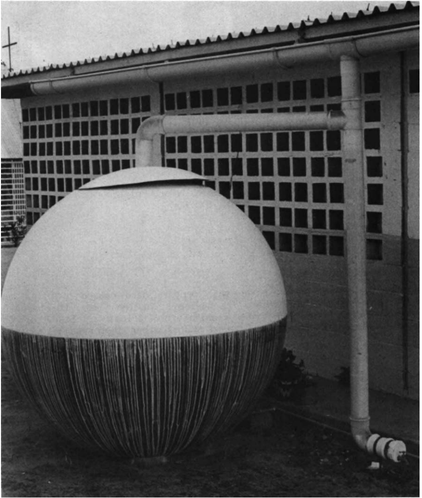
Fig. 2 Details of the first-flush system for keeping debris from the roof out of the tank.
