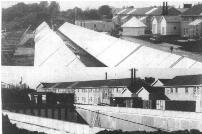
Fig. 1. Photo of the building project Tubberupvænge in Herlev where a low energy design and 400 m 2 of local solar collectors are used together with a central solar heating plant with 1050 m 2 of high temperature solar collectors and a 3000 m 3 seasonal storage under the wide part of the solar collector field. This total energy system is expected to save 80% of the "normal" gas consumption for heating.
