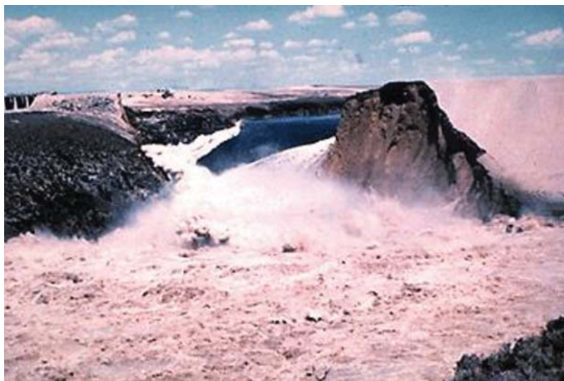
Figure 1.2 Teton Dam collapse on 5 June 1976. (Reproduced with permission of U.S. Department of the Interior)
