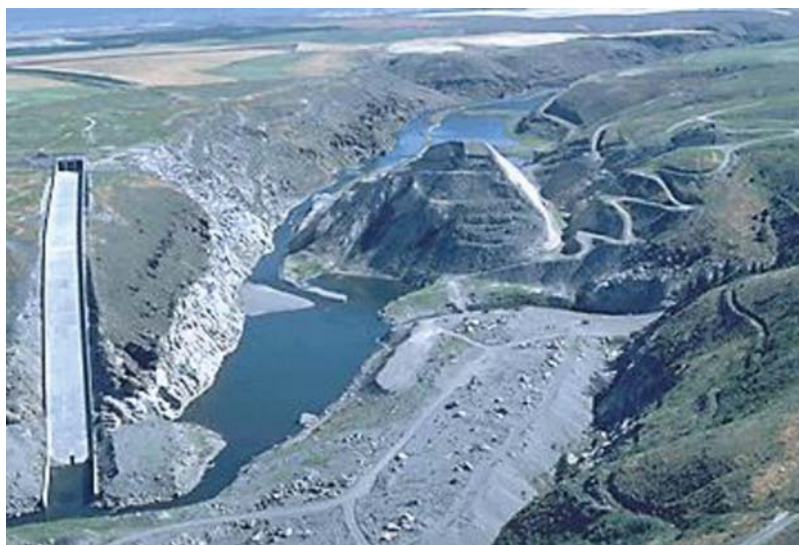
Figure 1.3 View of the Teton Dam after collapse. (Reproduced with permission of U.S. Department of the Interior)
