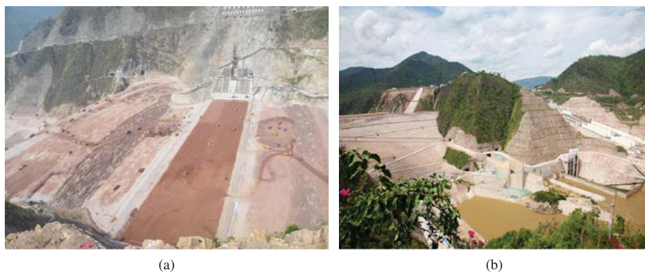
Figure 10.4 Nuozhadu Dam in construction. (a) Overhead view and (b) full view
