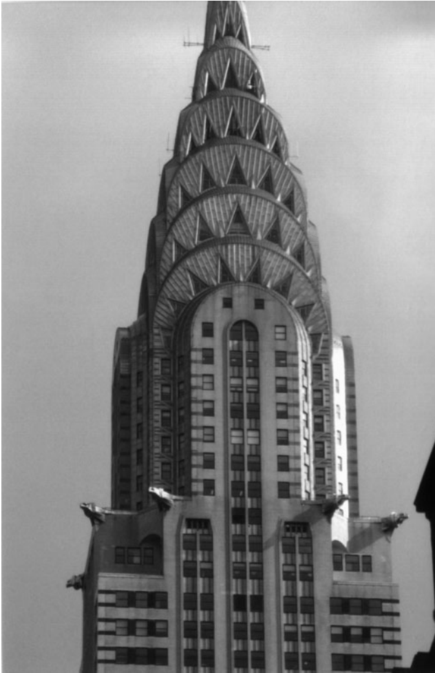
Figure 1.5 Chrysler Building – architect: William Van Allen, 1930.
