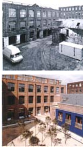
Above: The redevelopment of Britannia Mills has brought new life to these redundant historic warehouses Urban Splash
