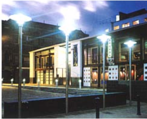
Right: Manchester's Smithfield Buildings: a vacant department store converted into popular new loft apartments
