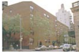
Above: New buildings have filled empty lots on the far west side of New York's Greenwich Village
