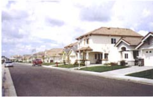
Top right: Suburban housing at Laguna West fails to deliver the density aspired to in the original masterplan
