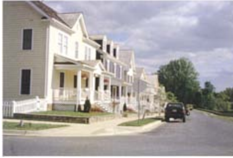
Right: Construction of a traditional neighbourhood at Kentlands, near Washington DC, started in 1990
