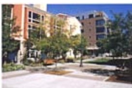
Below: The development plan integrates private space with good quality public open space
