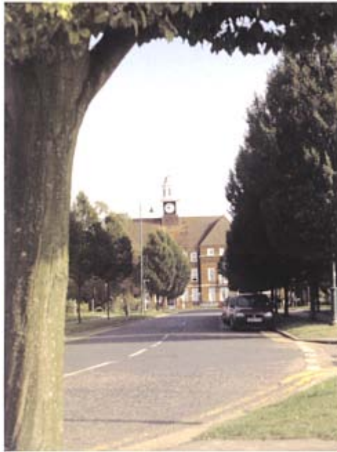
Right: Civic buildings make a significant contribution to the urban structure of Letchworth Garden City
