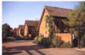
Top: Milton Keynes sought to provide sustainable models for housing using renewable energy and maximizing solar gain
