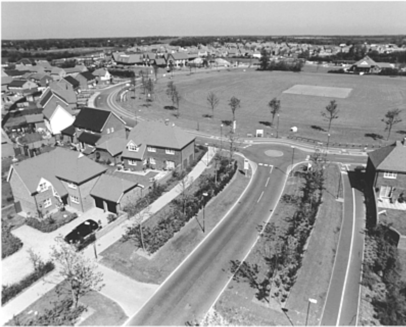
Below: A comprehensive management regime for all of Great Notley's public spaces was put in place at the outset of construction
