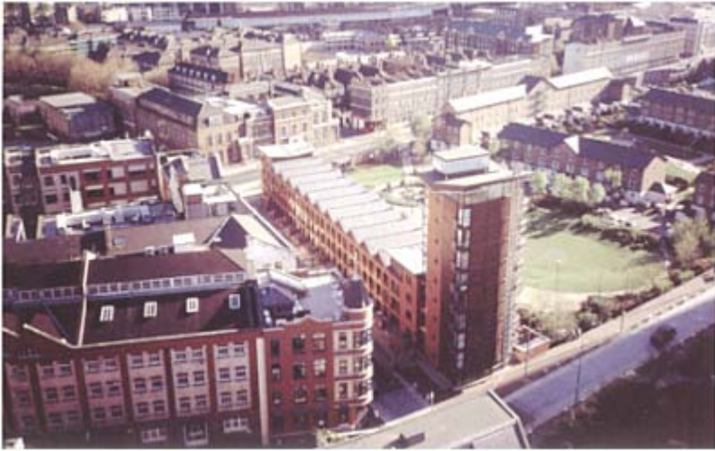
Above: London's Coin Street provides a good mix of offices, shops, flats and houses centred on a public park
