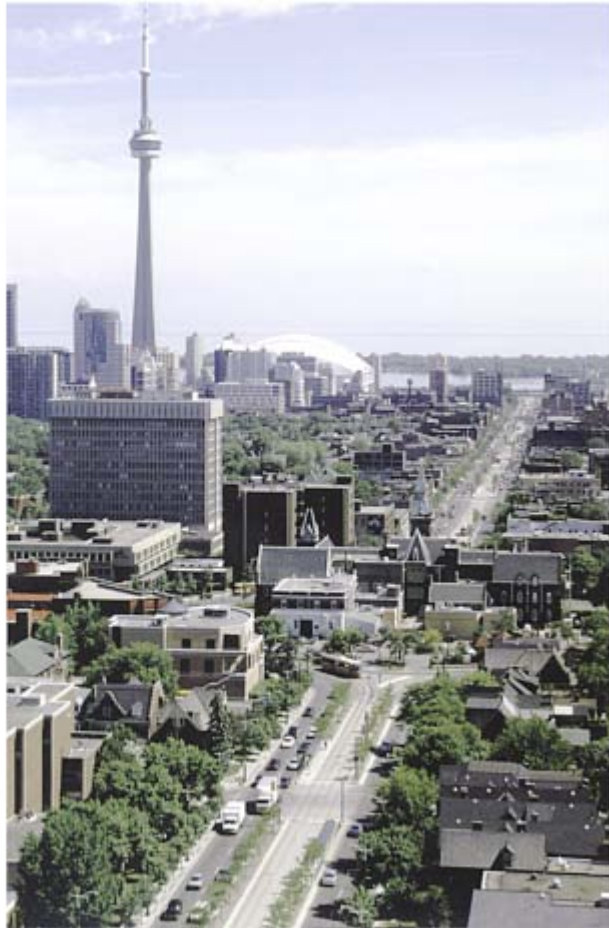
Right: Looking south from Wilcocks Street with the introduction of Light Rail transit
