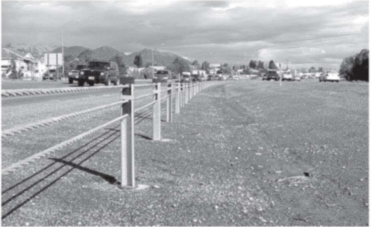
Figure 6.5 The Cable Safety System (CASS)
