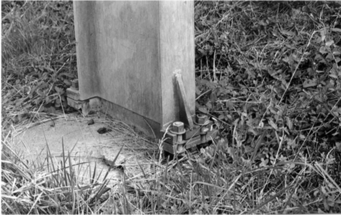
FIGURE 4.5 Typical uni-directional slip base
