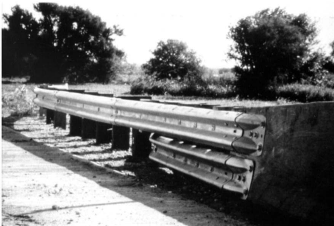
FIGURE 7.17 W-beam transition to vertical concrete rail
