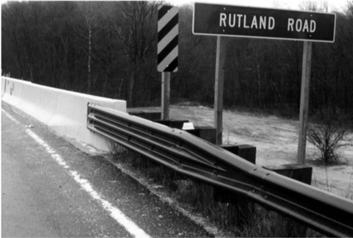
FIGURE 7.19 Thrie-beam transition to modified concrete safety shape
