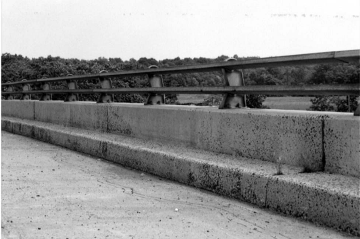
FIGURE 7.12 Presence of brush curb
