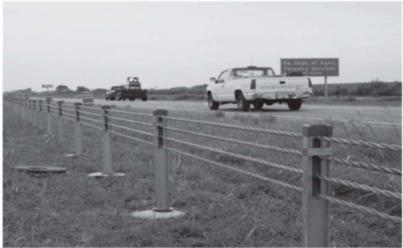
Figure 6.7 Safence Cable Barrier System
