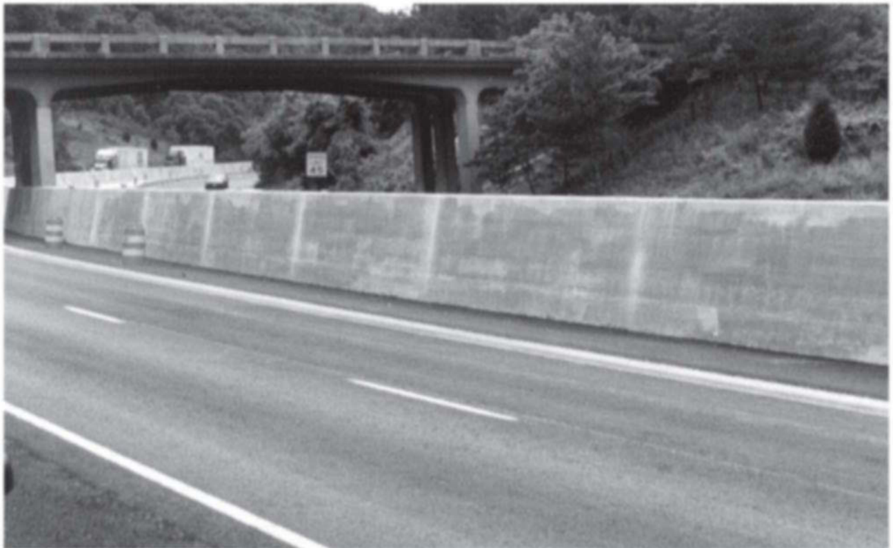
Figure 6.14 Single-slope concrete median barrier
