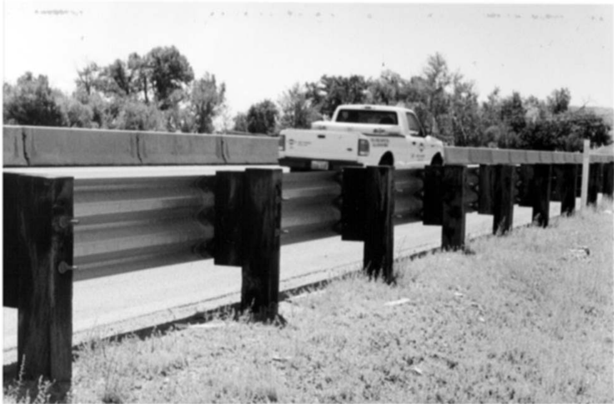
FIGURE 5.11 Wood post thrie-beam barrier
