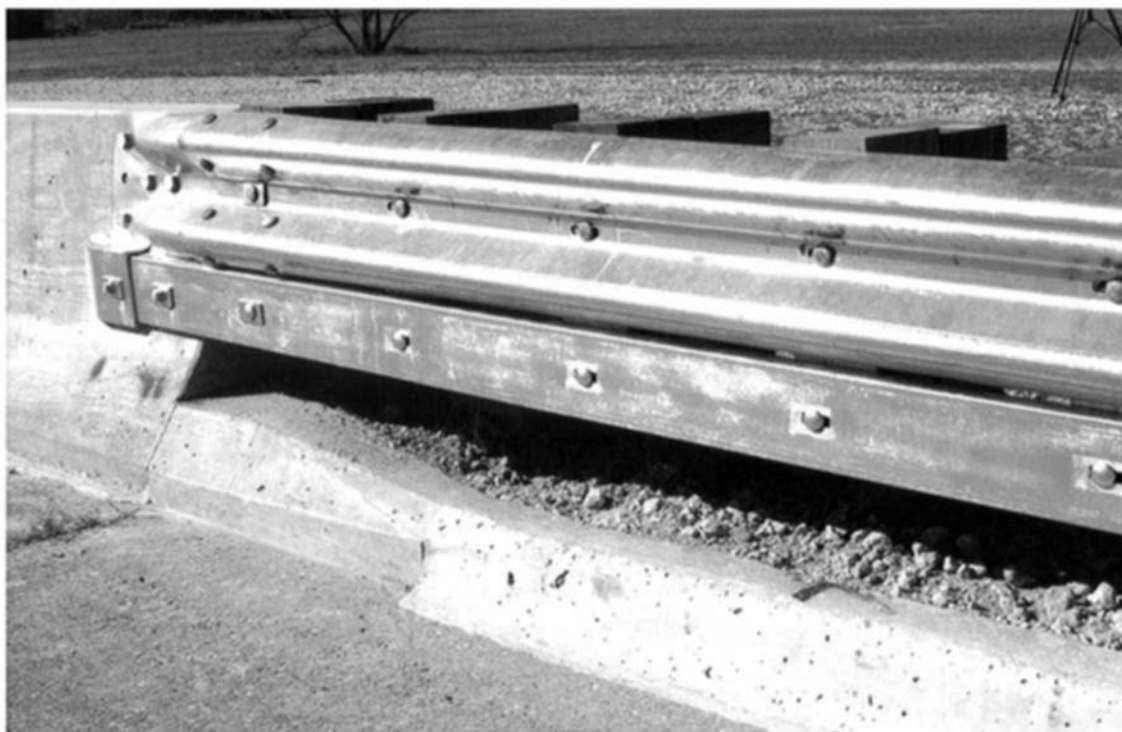
FIGURE 7.18 W-beam transition to modified concrete safety shape
