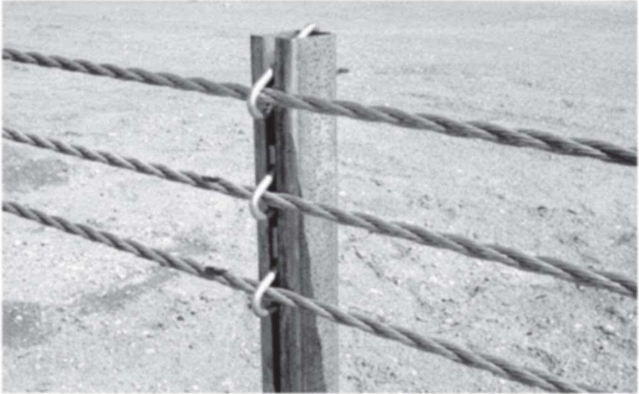
Figure 6.8 Gibraltar Cable Barrier System
