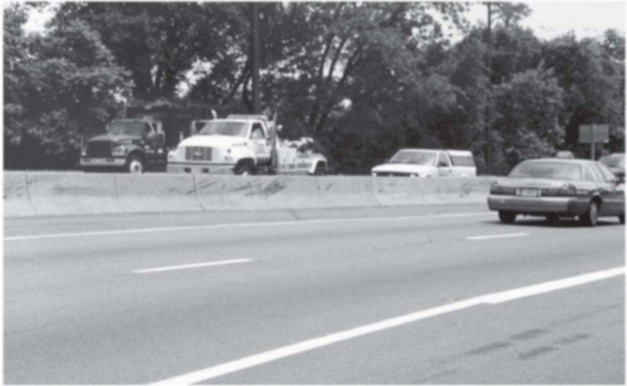
Figure 6.12 Concrete safety-shape median barrier
