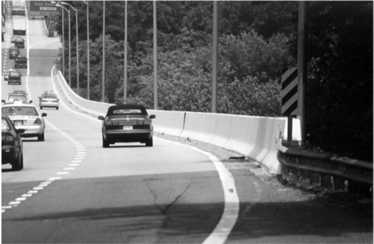
FIGURE 7.5 Tall concrete safety-shape railing
