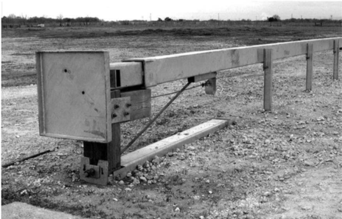
FIGURE 8.4 Wyoming box beam end terminal
