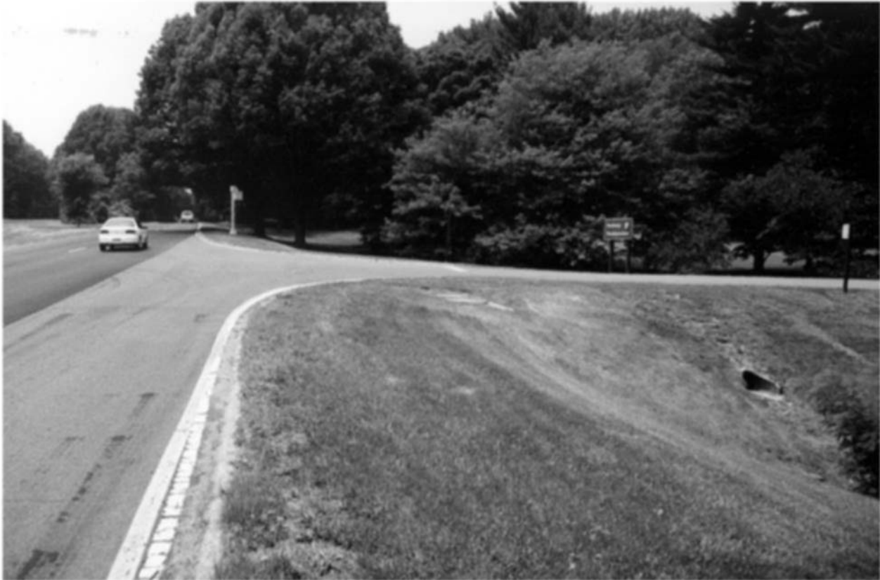
FIGURE 3.3 Preferred cross slope design
