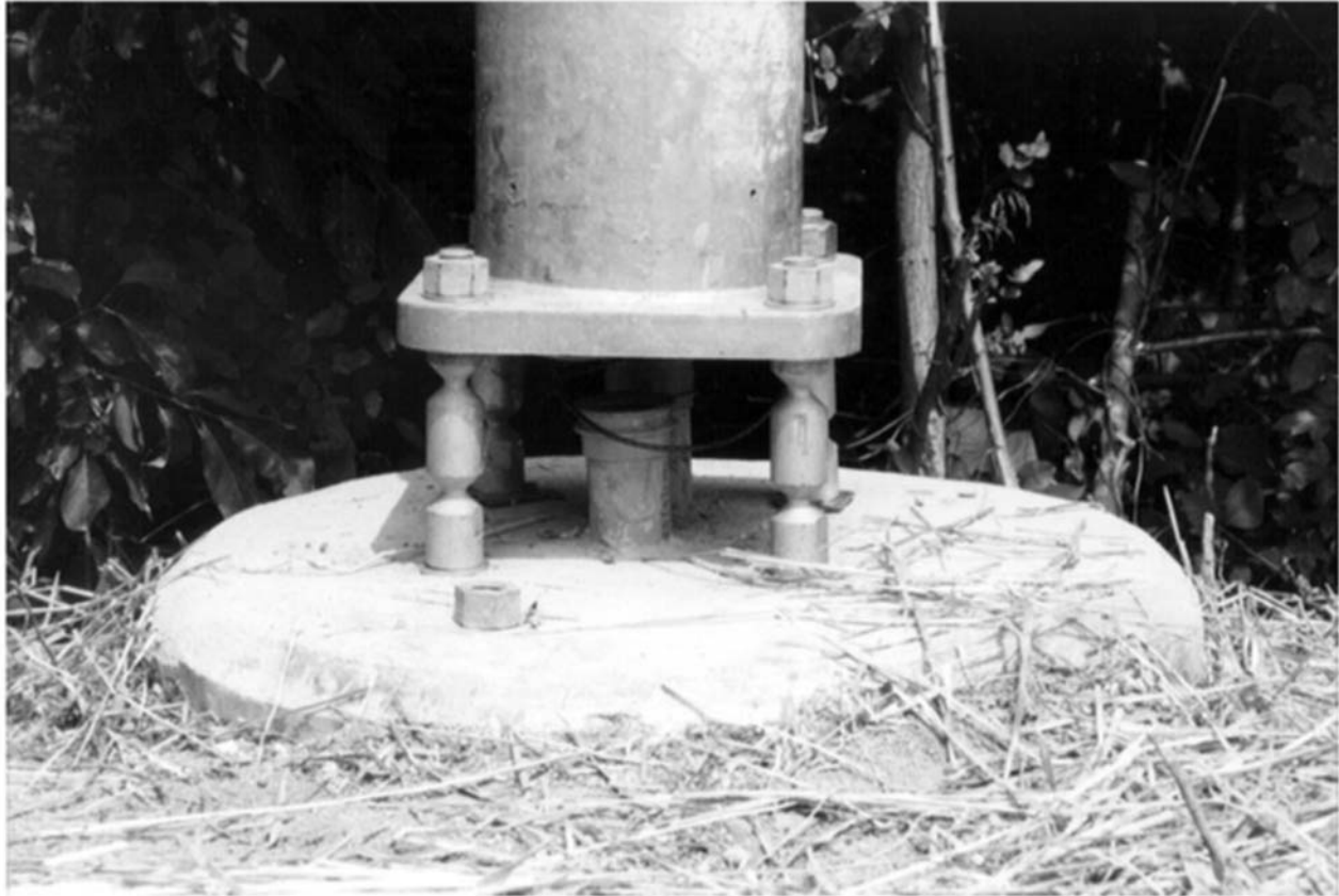
FIGURE 4.13 Example of a frangible coupling design
