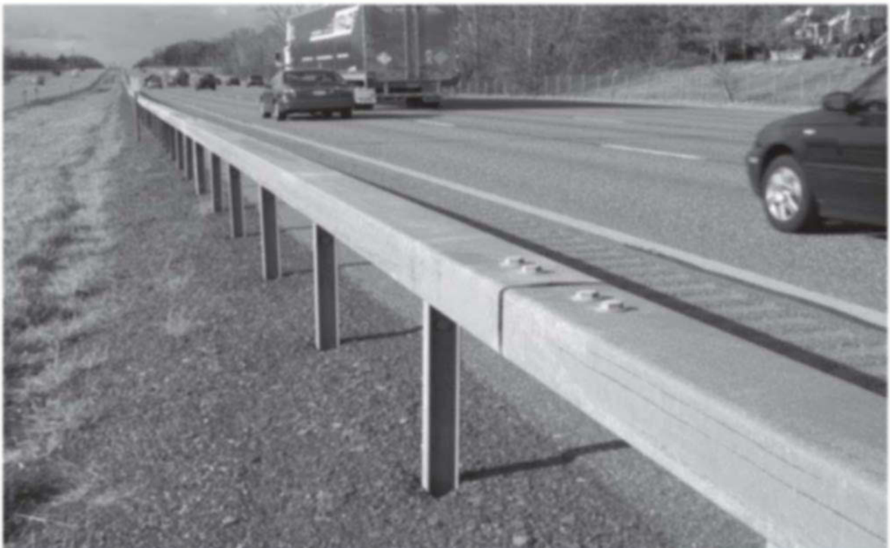
Figure 6.9 Box-beam median barrier
