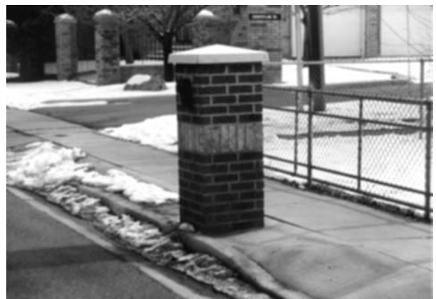
FIGURE 11.2 Examples of hazardous single mailbox installations
