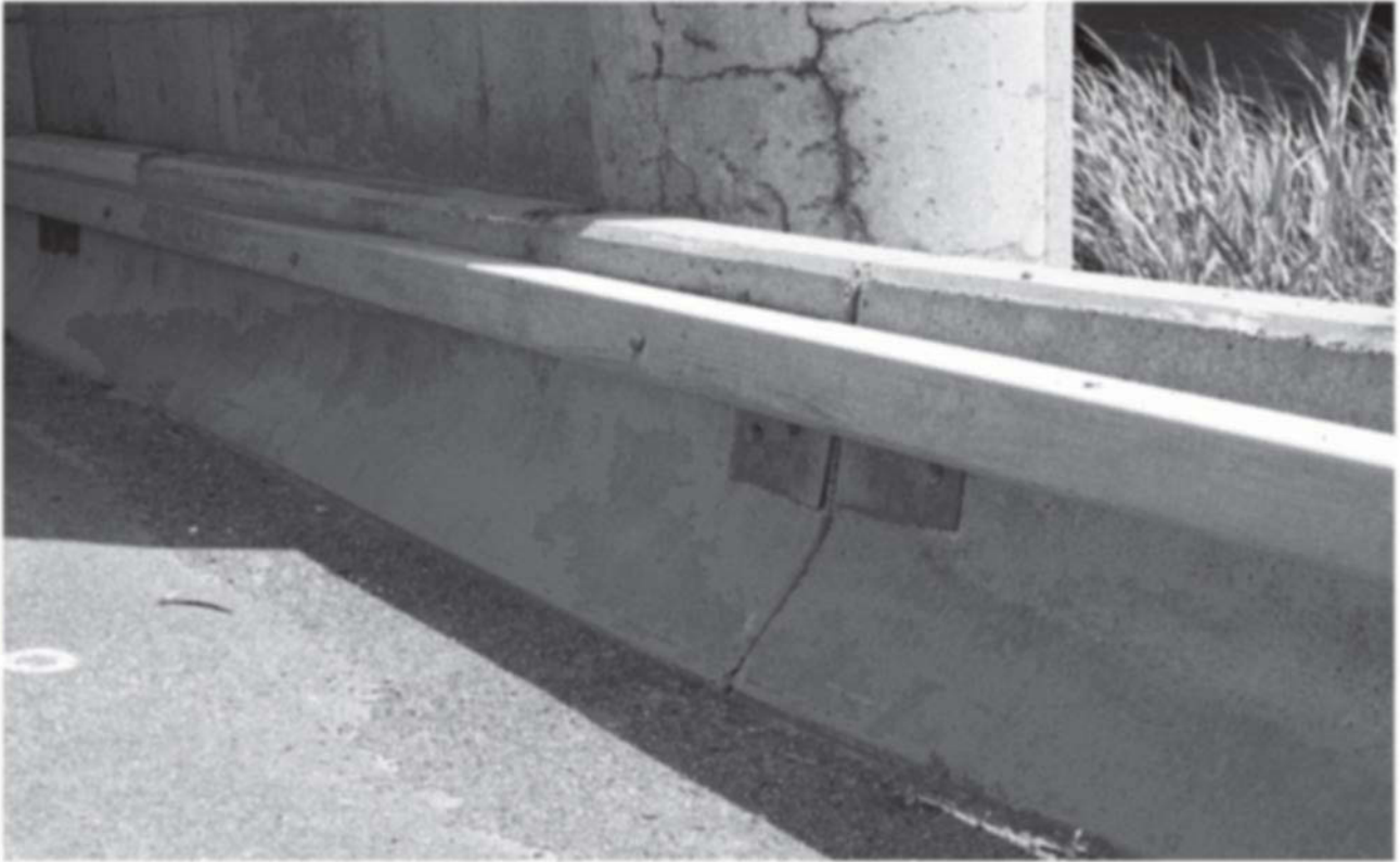
Figure 6.13 New York retrofit of concrete barrier
