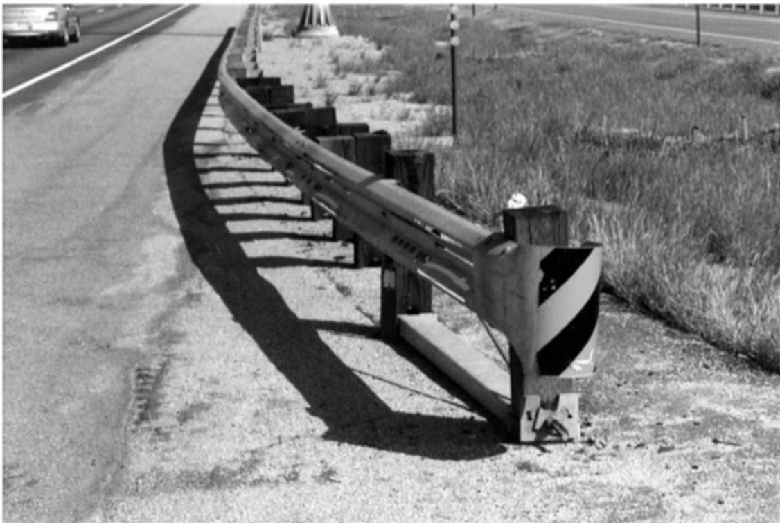
FIGURE 8.10 Slotted rail terminal (SRT-350) with 0.9 m [3 ft] flare
