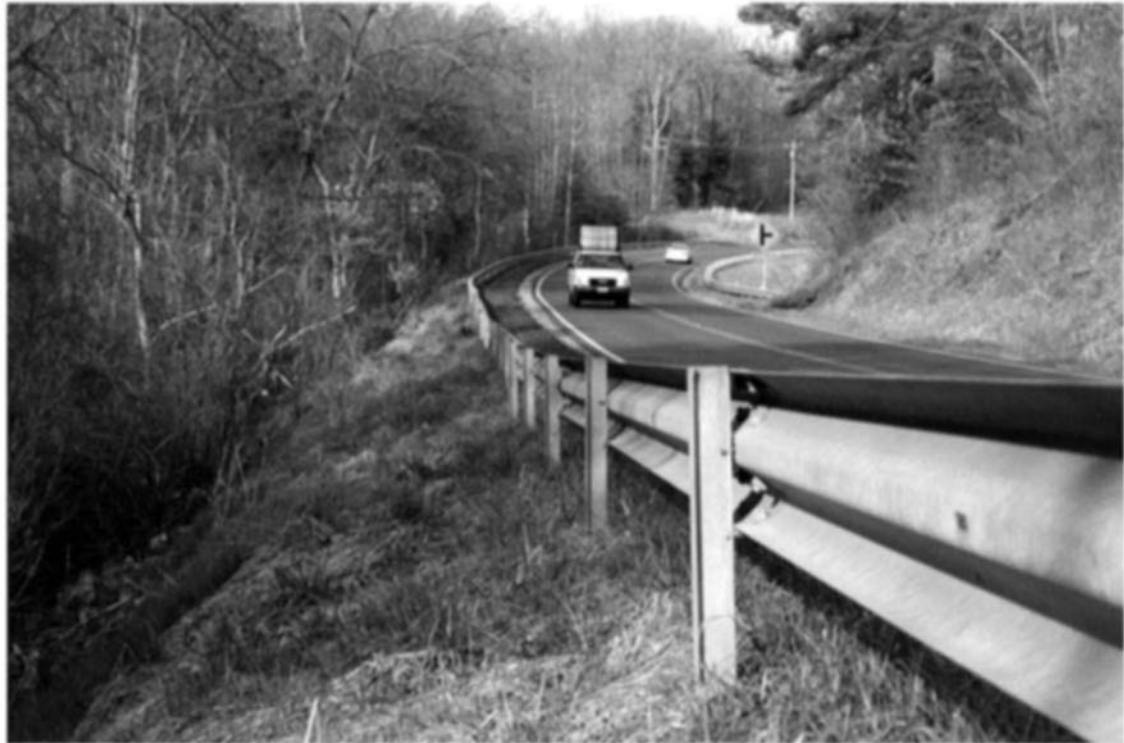
FIGURE 5.6 Weak post W-beam barrier
