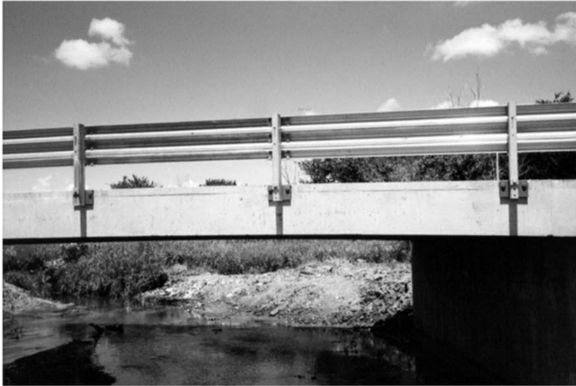
FIGURE 7.1 Side-mounted, three-beam bridge railing
