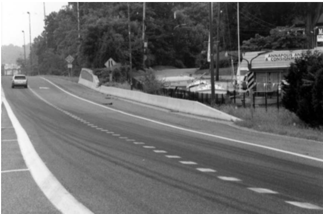
FIGURE 8.19 Sloped concrete end treatment
