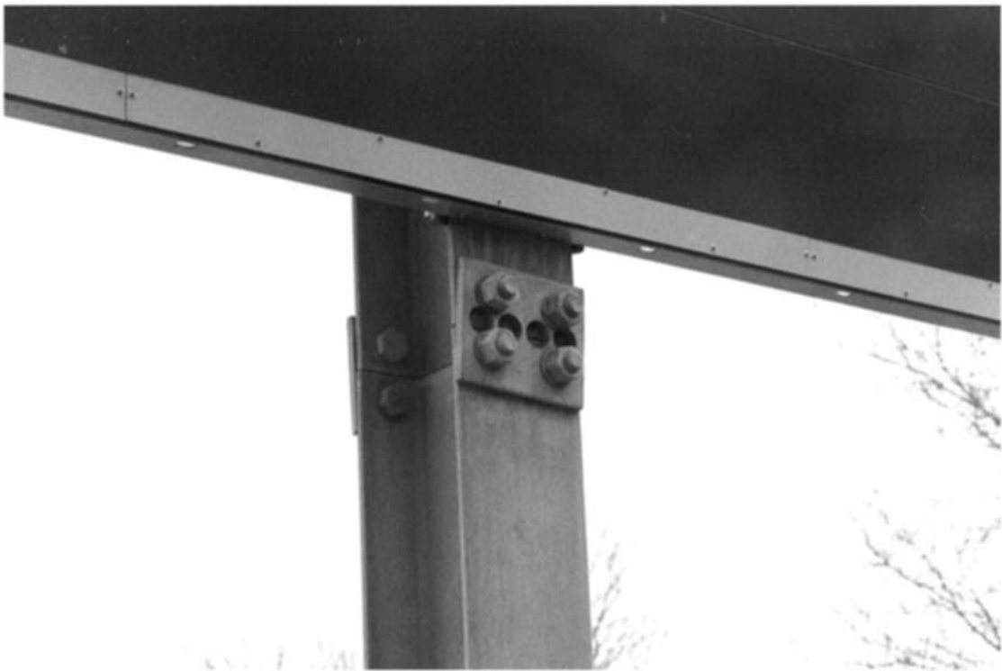
FIGURE 4.7 Perforated fuse plate design
