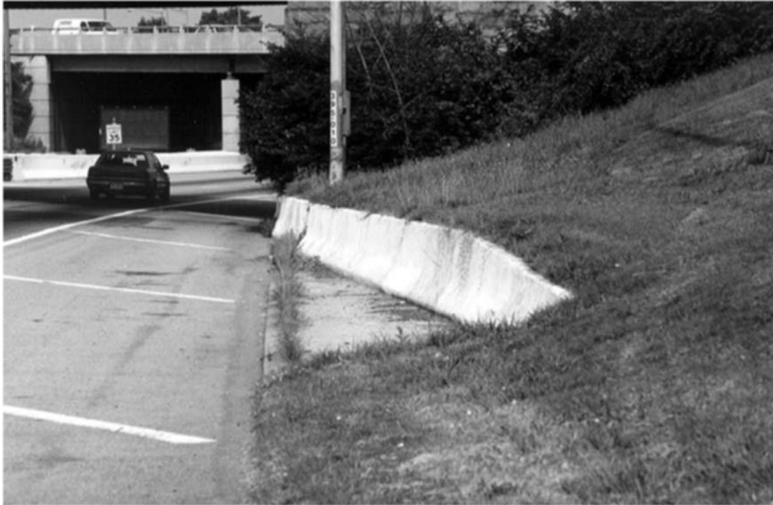
FIGURE 8.5 Barrier anchored in backslope
