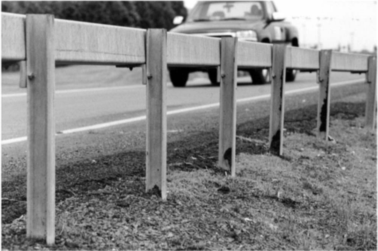
FIGURE 5.8 Weak post box beam barrier
