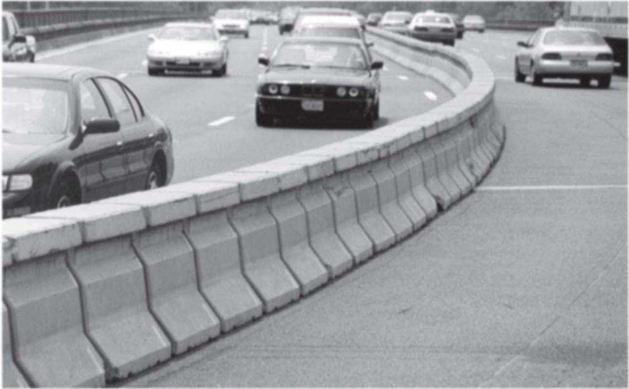
Figure 6.15 Quickchange® moveable barrier system
