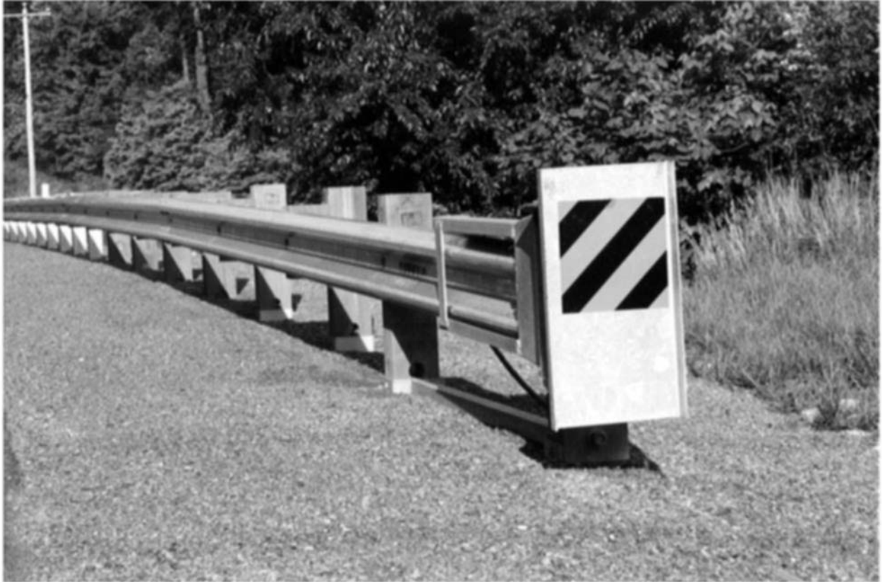
FIGURE 8.15 Extruder Terminal (ET-2000)
