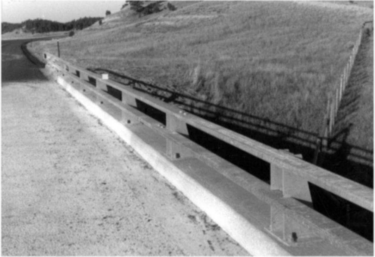
FIGURE 7.2 Wyoming two-tube bridge railing
