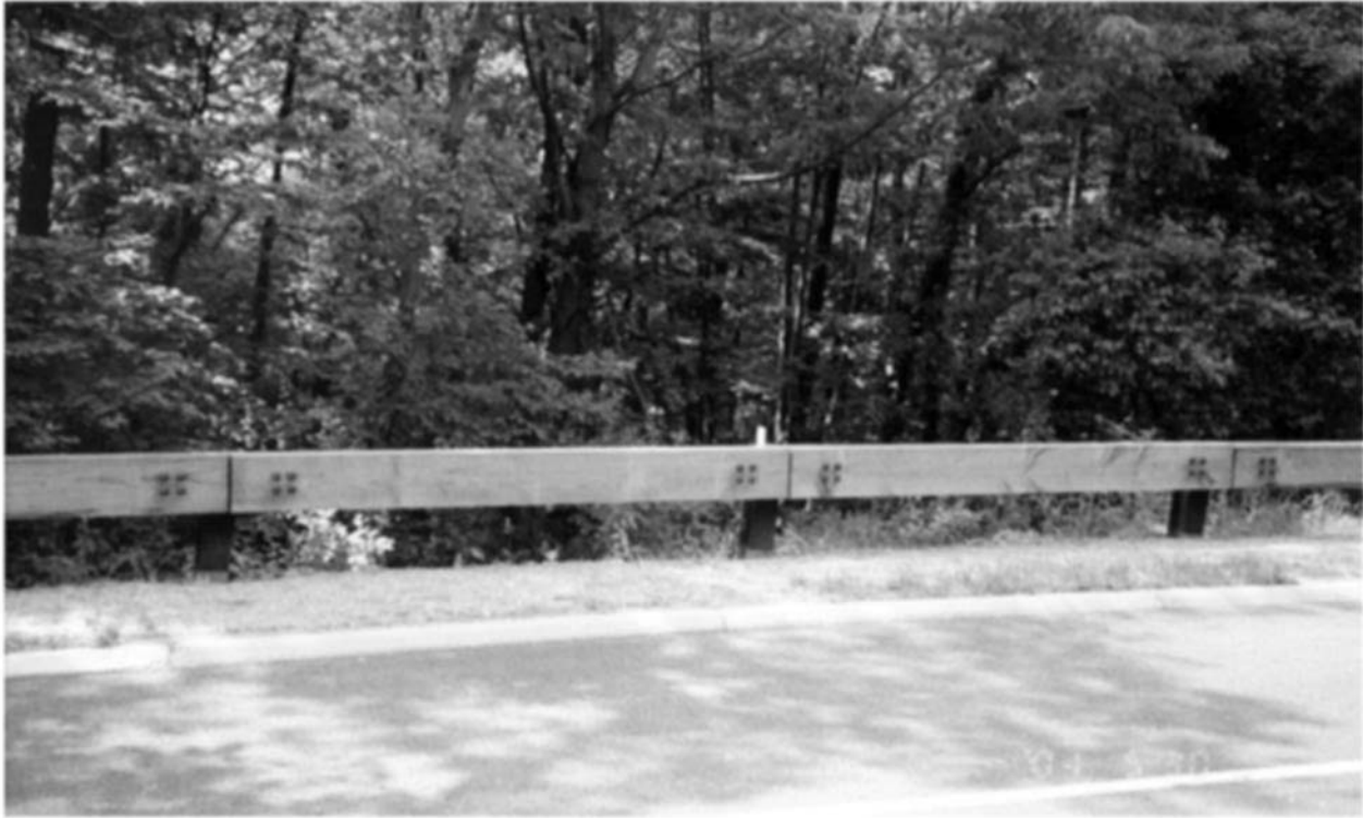
FIGURE 5.13 Merritt Parkway aesthetic guardrail
