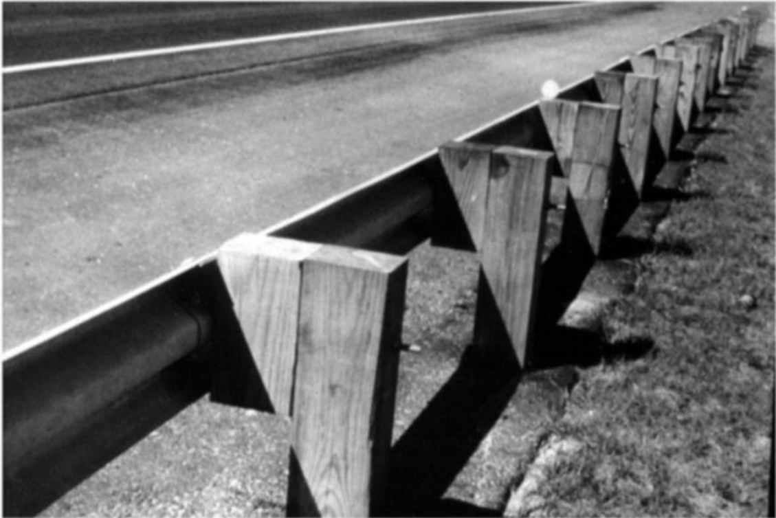
FIGURE 5.10 Wood post W-beam with wood block-outs
