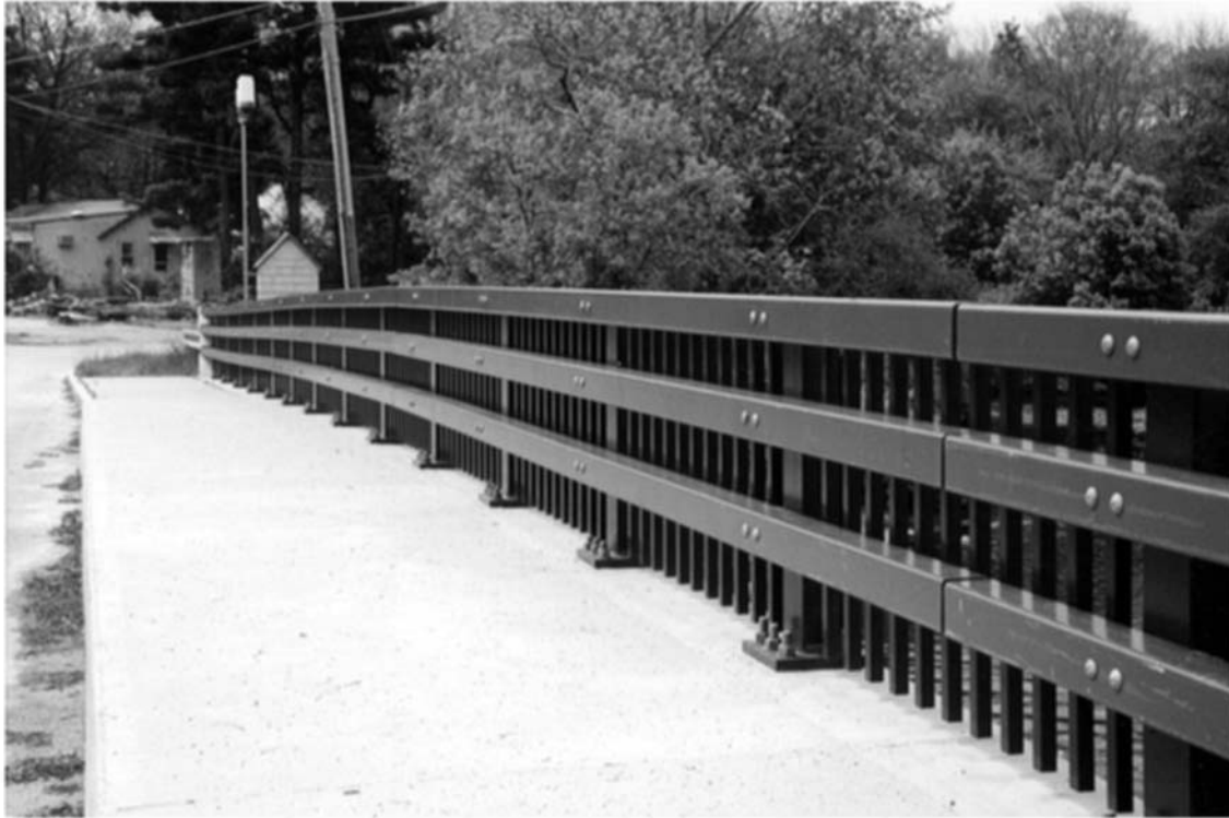
FIGURE 7.3 Massachusetts S3 steel bridge railing
