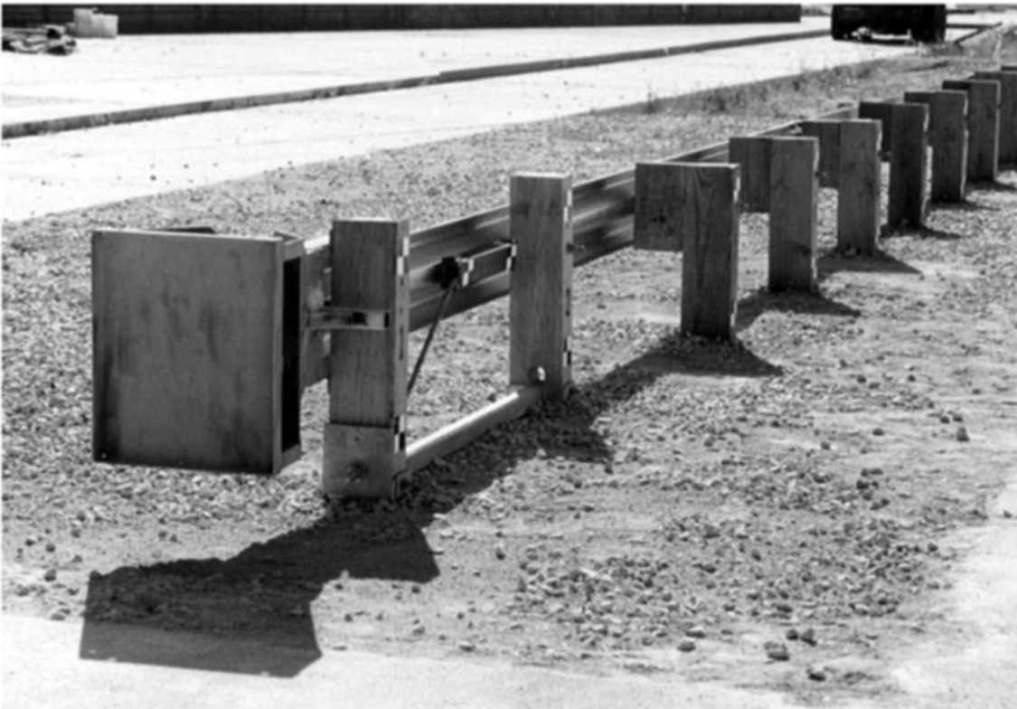
FIGURE 8.14 Beam Eating Steel Terminal (BEST)
