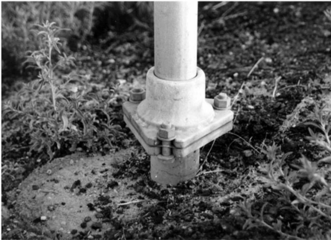
FIGURE 4.9 Multidirectional slip base for small signs
