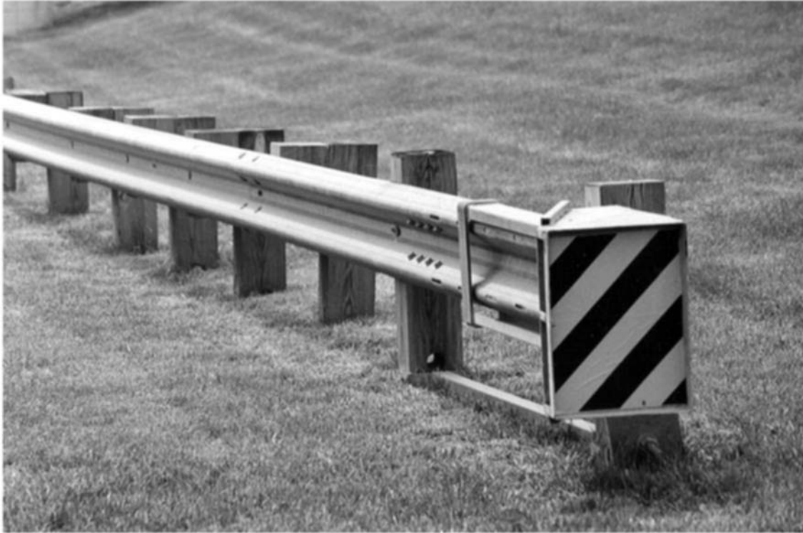
FIGURE 8.13 Flared Energy-Absorbing Terminal (FLEAT)
