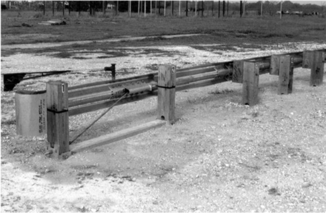
FIGURE 8.9 Slotted rail terminal (SRT-350) with 1.2 m [4 ft] flare
