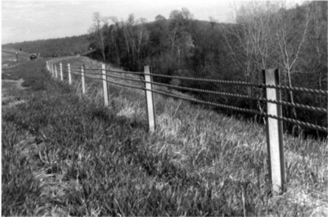
FIGURE 5.5 Three-strand cable barrier
