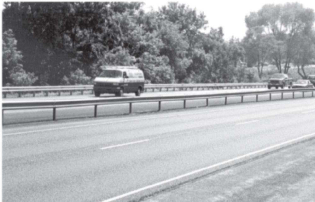
Figure 6.2 Weak-post, W-beam median barrier
