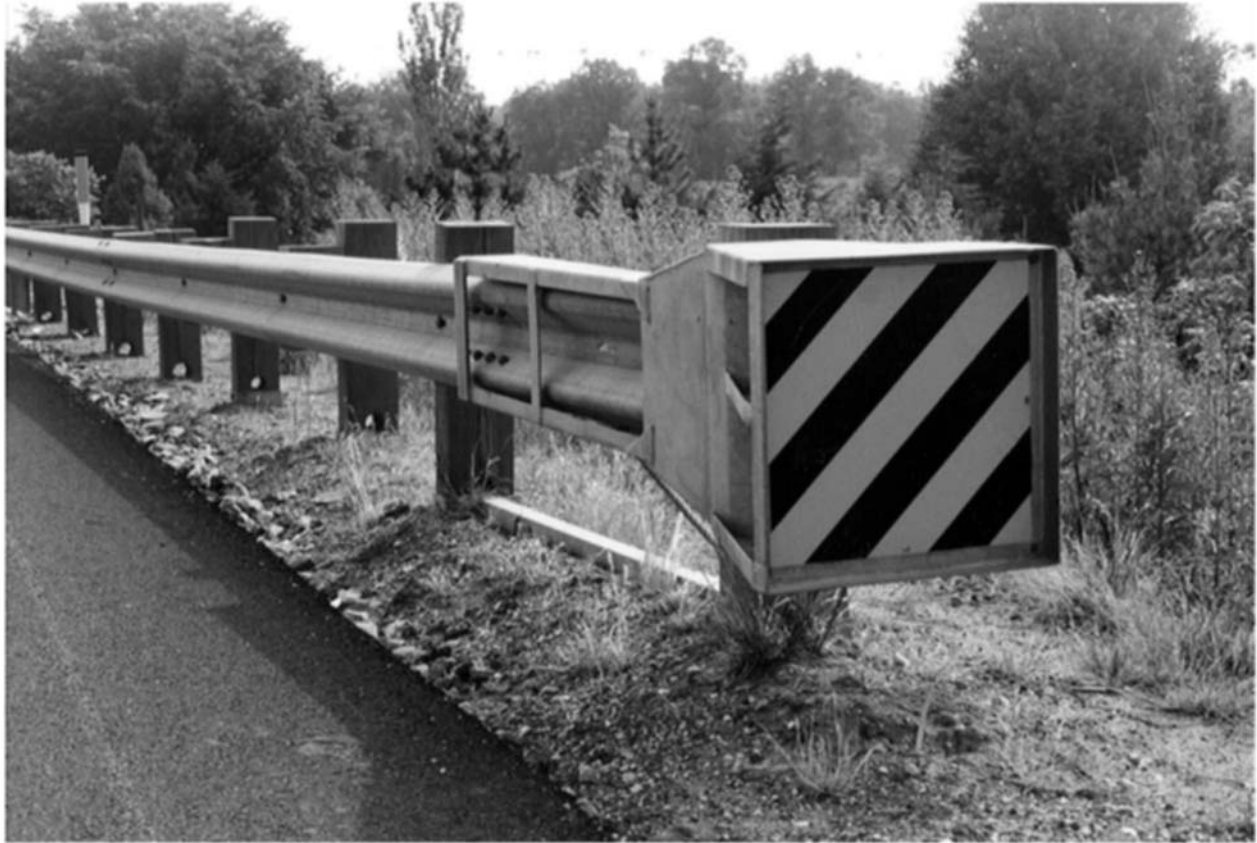
FIGURE 8.16 Sequential Kinking Terminal (SKT-350)
