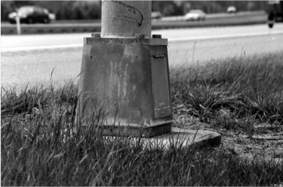
FIGURE 4.11 Example of a cast aluminum transformer base
