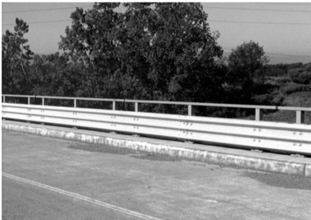
FIGURE 7.14 Thrie-beam retrofit (New York)
