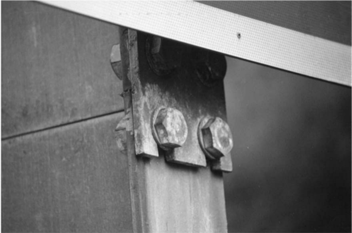
FIGURE 4.6 Slotted fuse plate design
