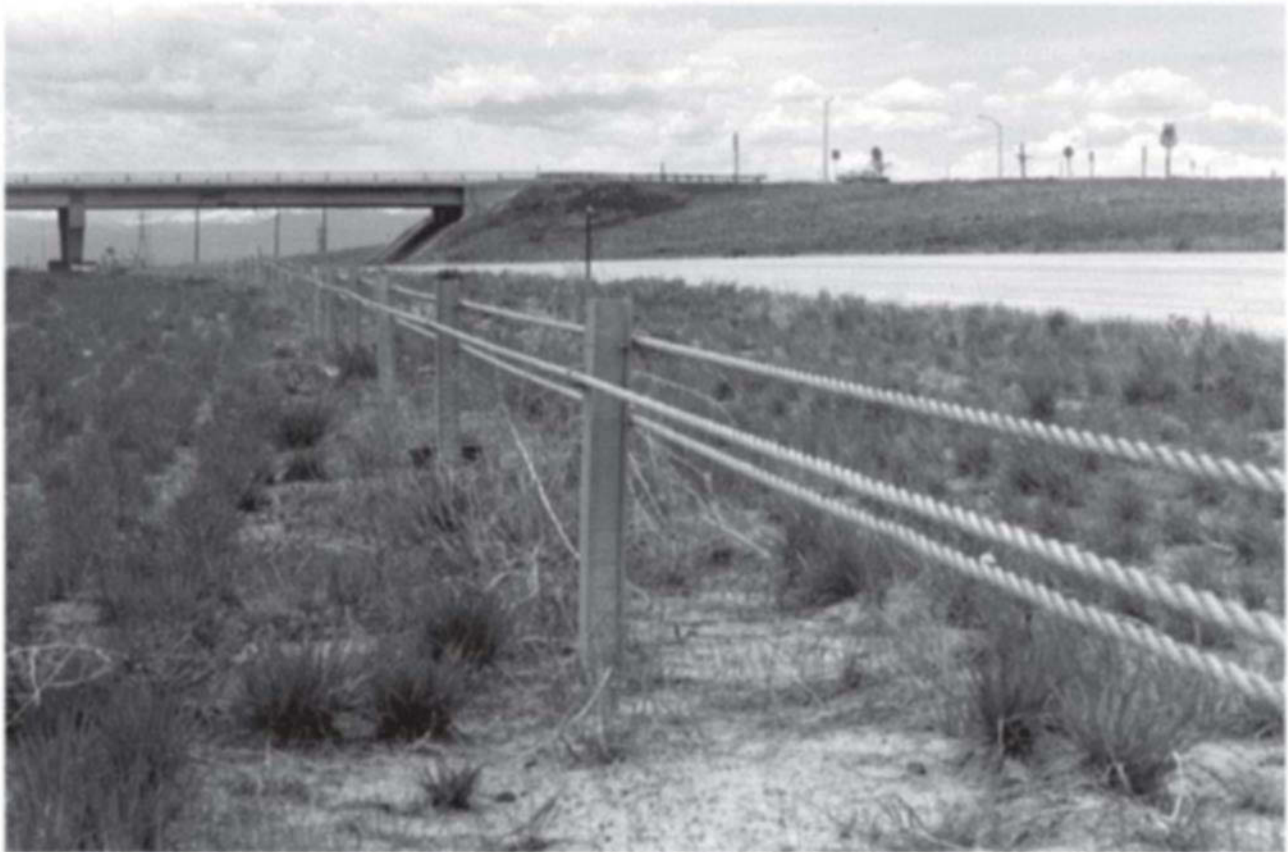
Figure 6.3 Three-strand cable median barrier
