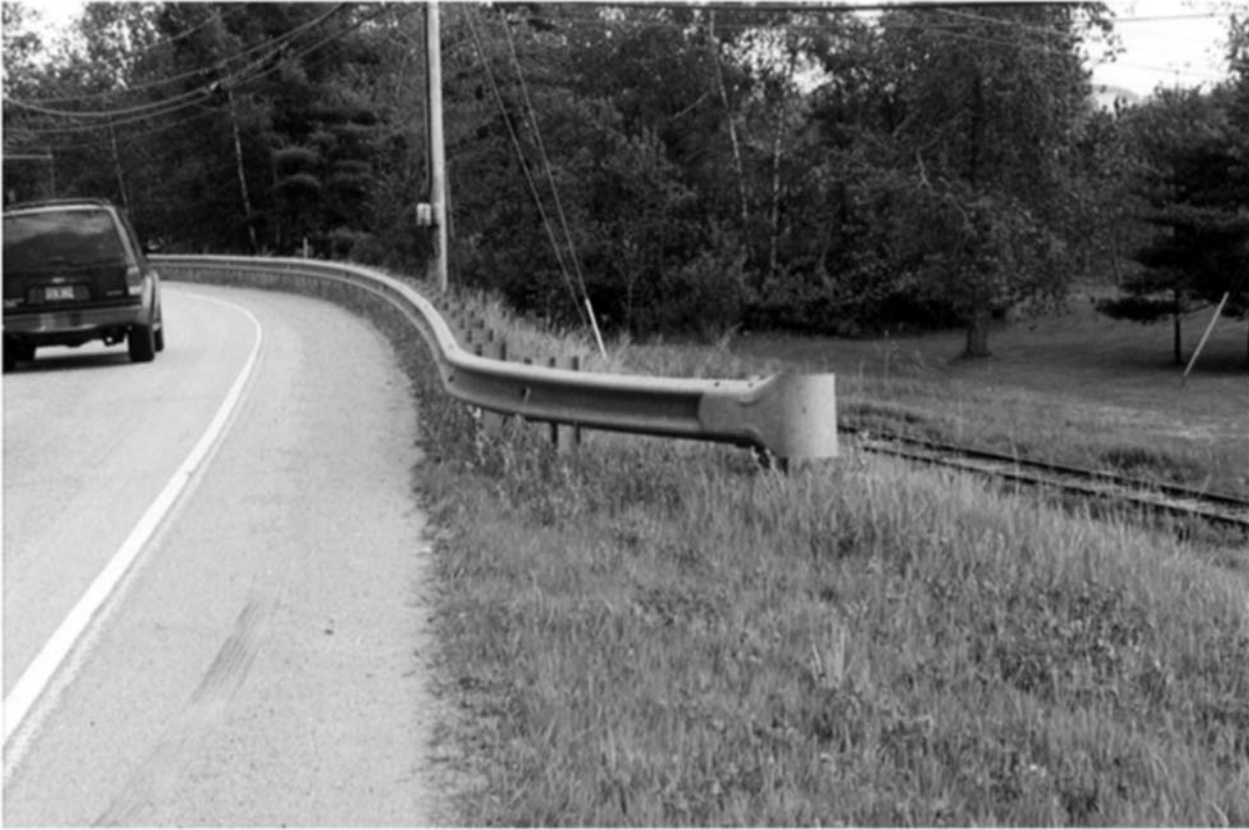
FIGURE 8.12 Vermont low-speed, W-beam guardrail end terminal
