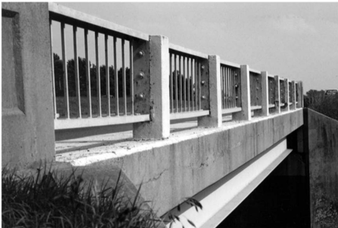
FIGURE 7.11 Snagging potential
