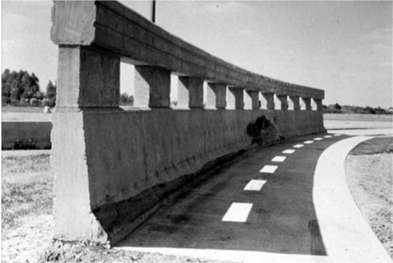
FIGURE 7.6 Texas Type TT (Tank Truck) railing
