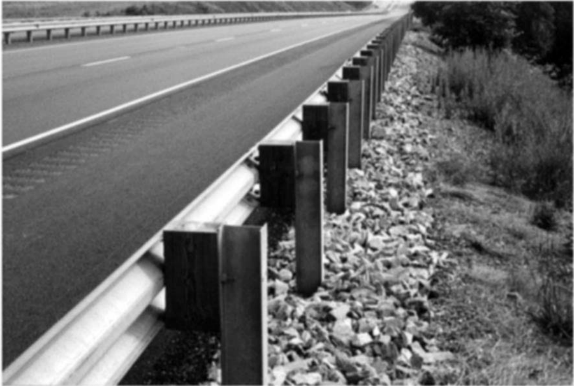
FIGURE 5.9 Steel post W-beam with wood block-outs
