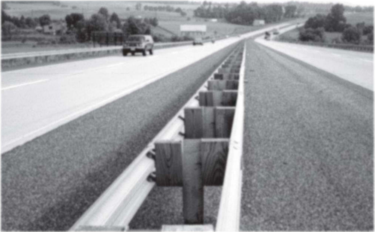
Figure 6.10 Strong-post W-beam median barrier
