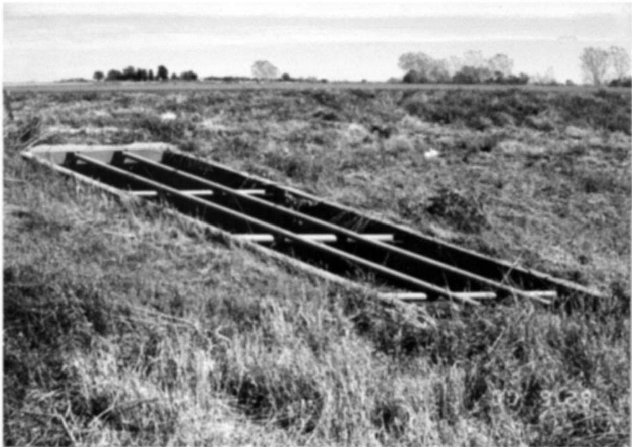
FIGURE 3.9 Safety treatment for cross-drainage culvert
