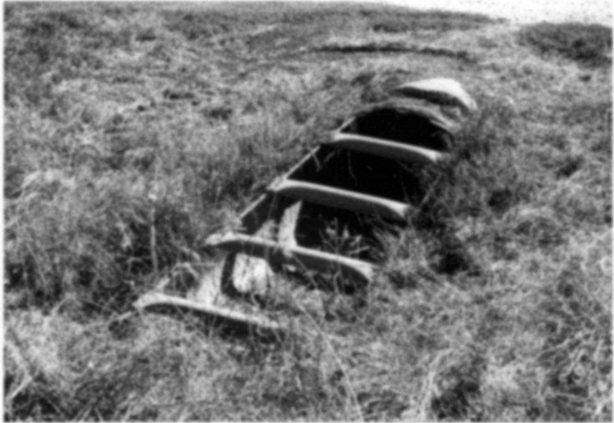
FIGURE 3.12 Safety treatment for parallel drainage pipe
