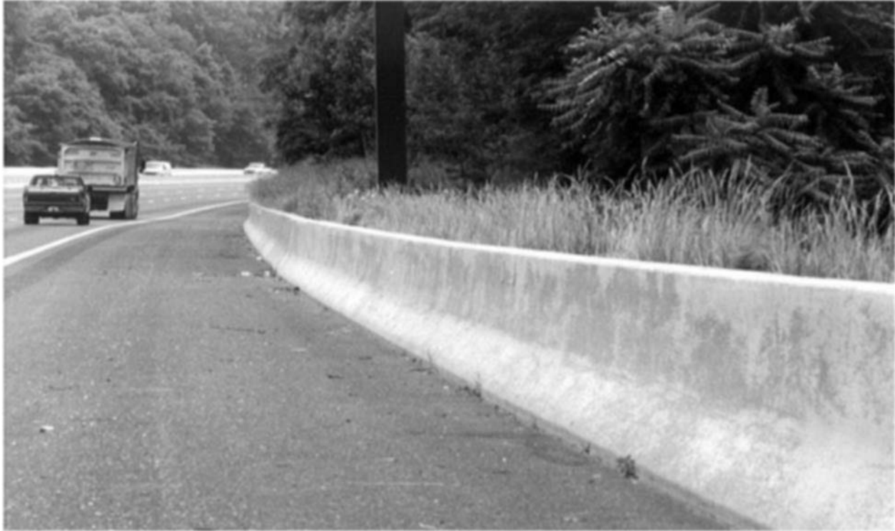
FIGURE 5.15 New Jersey safety-shape barrier
