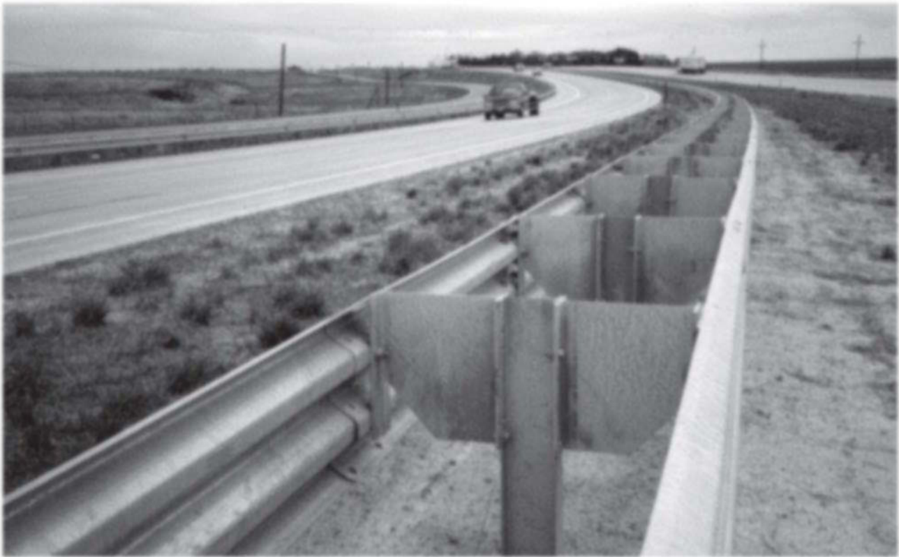
Figure 6.11 Modified thrie-beam median barrier
