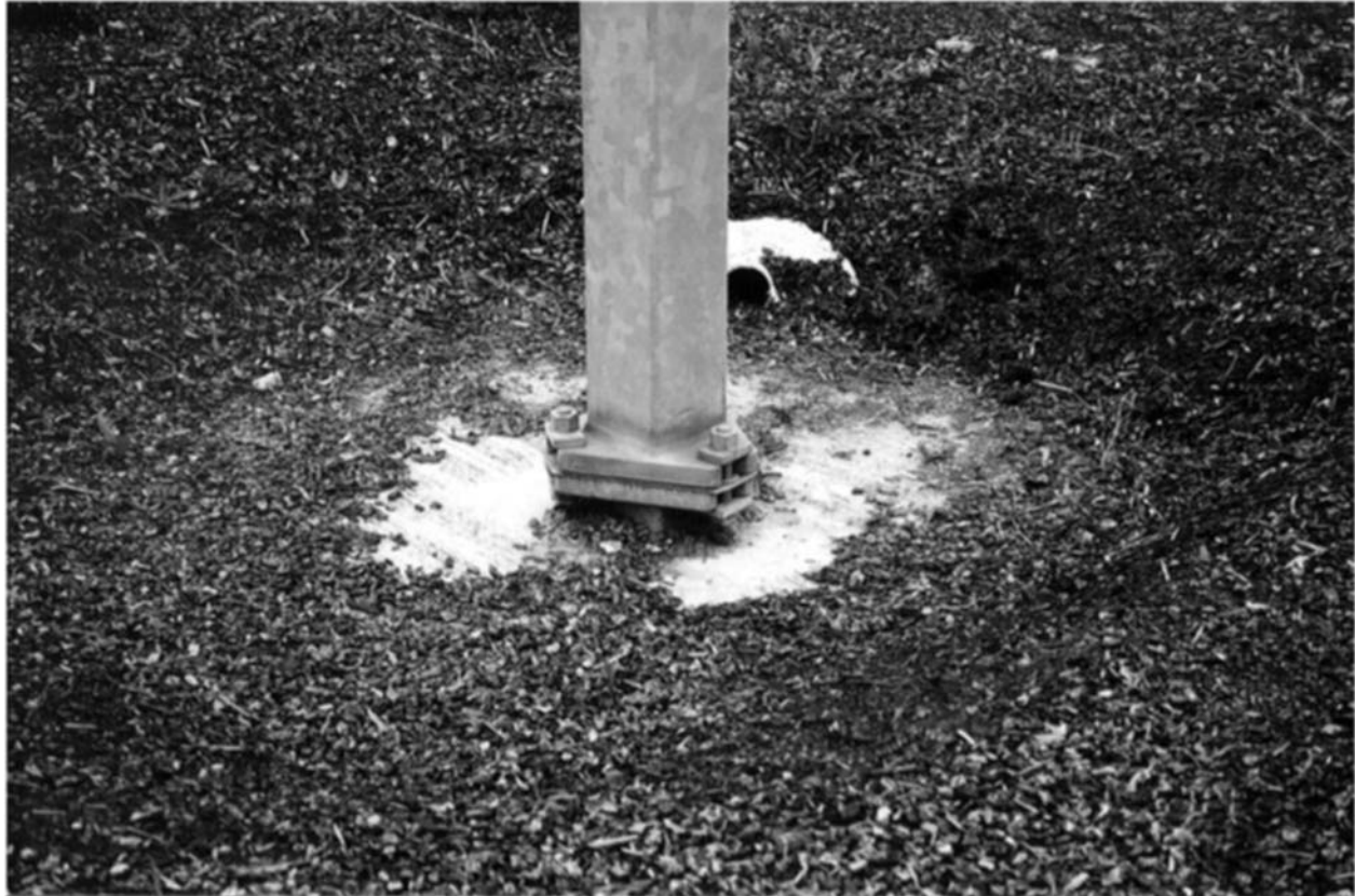
FIGURE 4.10 Oregon 3-bolt slip base
