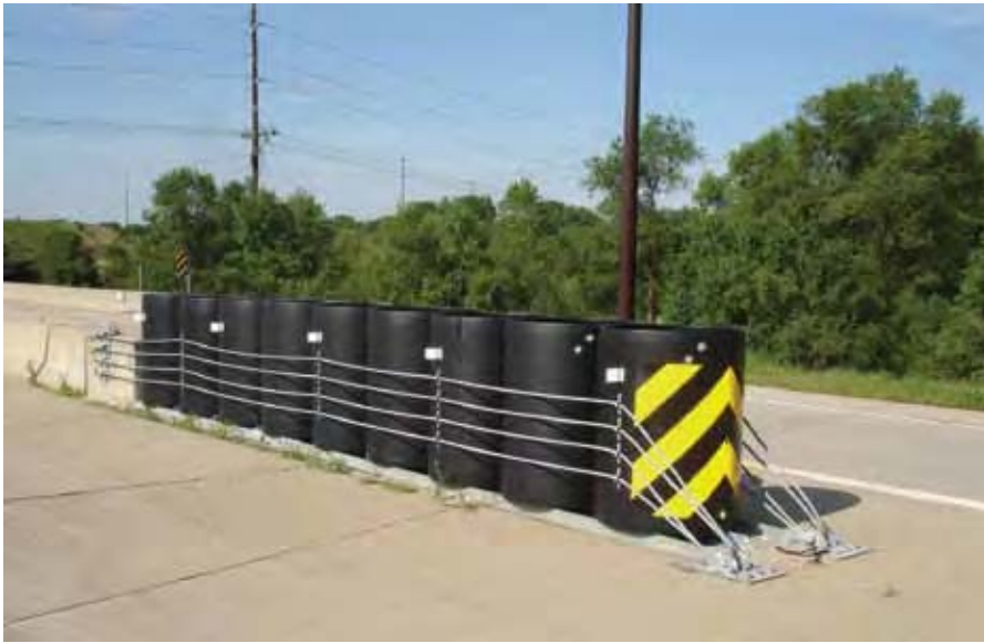
Figure 8-36. Reusable Energy-Absorbing Crash Terminal (REACT 350®)
