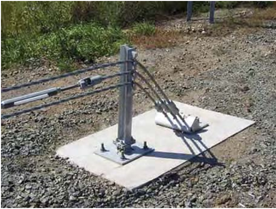
Figure 8-4. Three-Strand Cable Terminal
