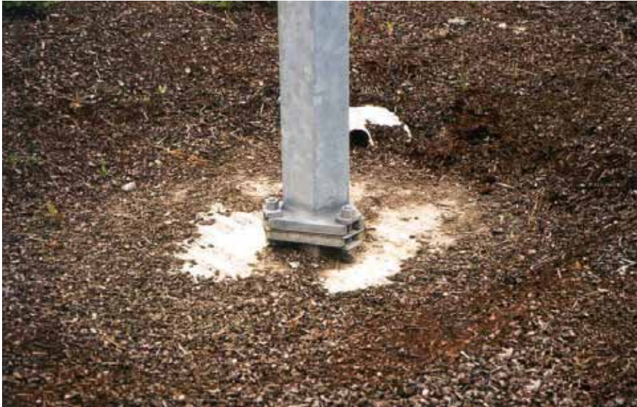
Figure 4-10. Oregon 3-Bolt Slip Base
