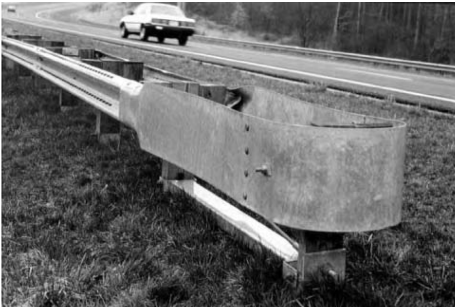
Figure 8-15. Crash Cushion Attenuating Terminal (CAT-350™)
