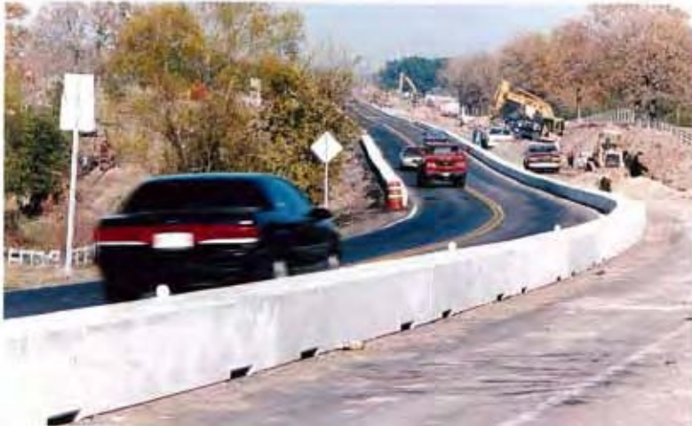
Figure 9-19. Low-Profile Barrier System
