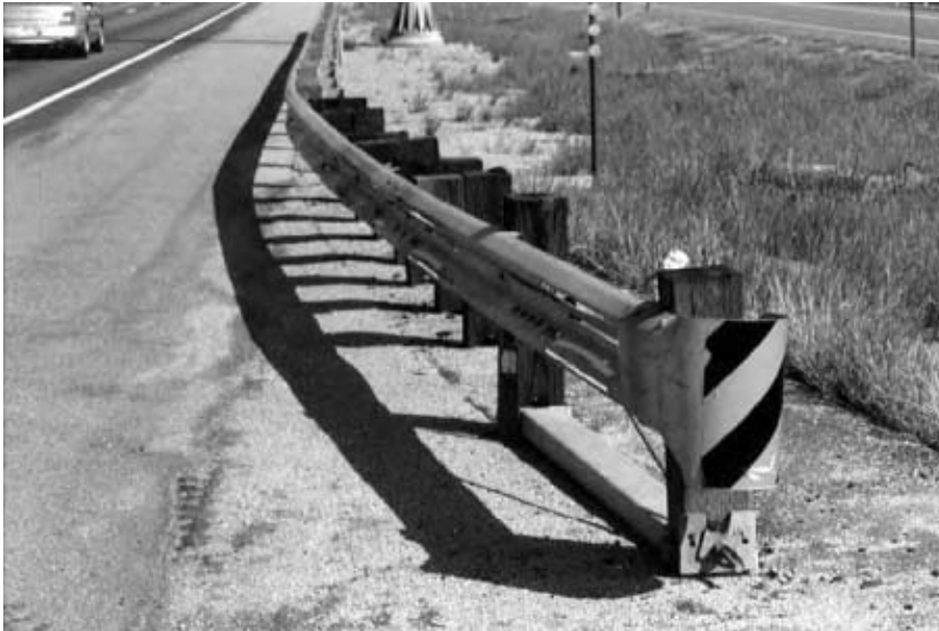
Figure 8-10. Slotted Rail Terminal (SRT-350™)
