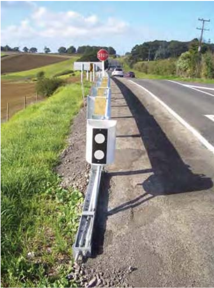
Figure 8-11. X-Tension Guardrail End Terminal
