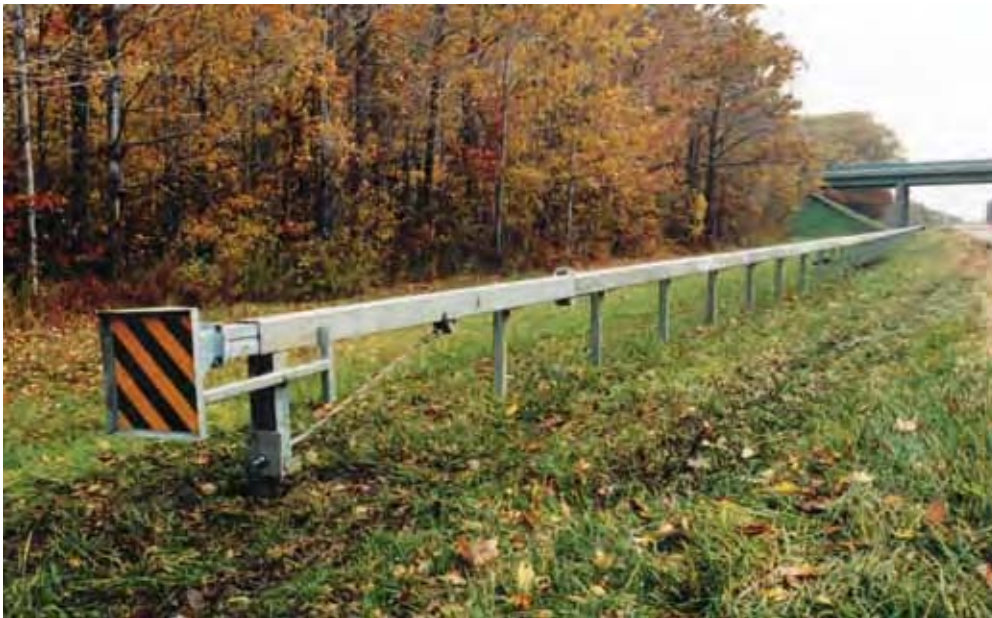
Figure 8-19. Bursting Energy Absorbing Terminal (BEAT™)
