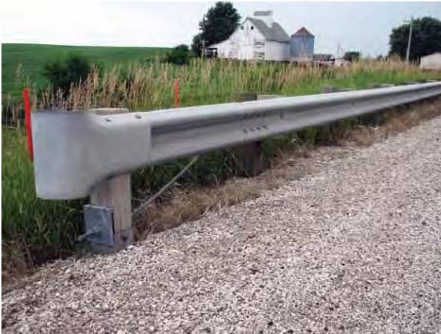
Figure 8-1. Trailing End W-Beam Guardrail Anchorage
