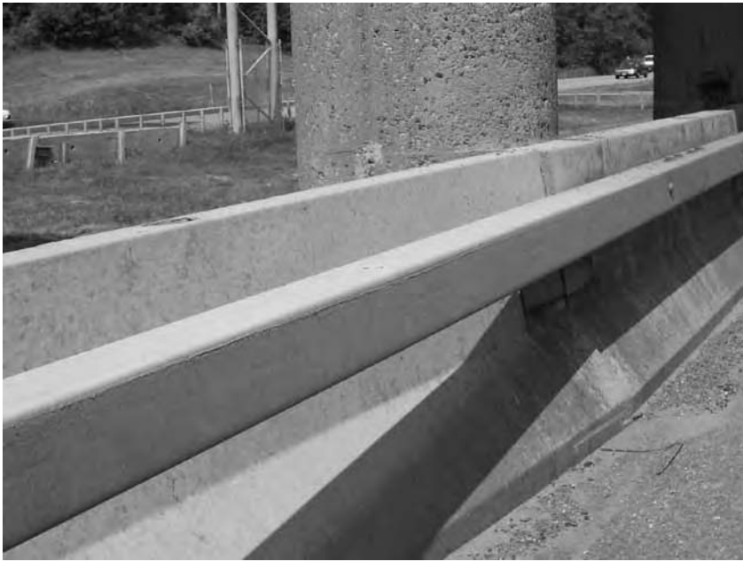
Figure 6-12. New York Modification of Concrete Barrier
