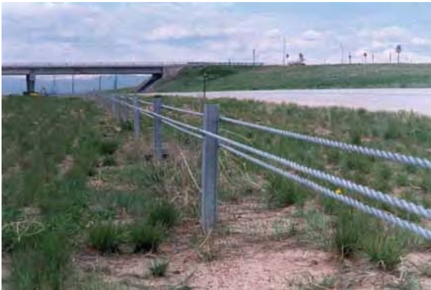
Figure 6-3. Three-Strand Cable Median Barrier
