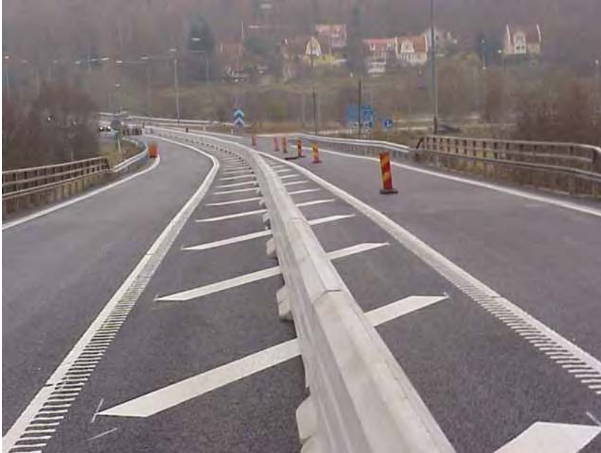
Figure 9-6. GPLINK® Pre-Cast Temporary Concrete Barrier
