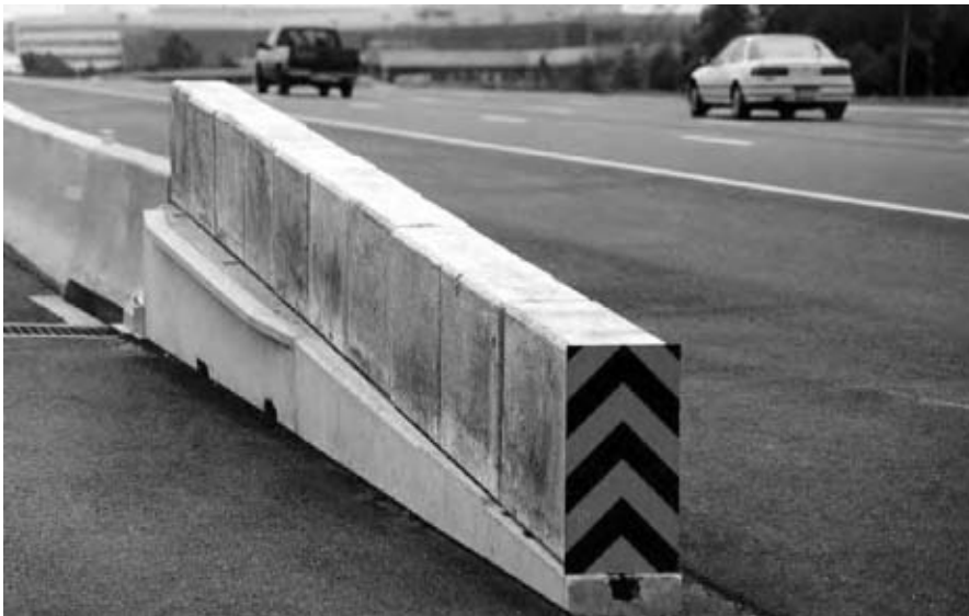
Figure 8-22. Advanced Dynamic Impact Extension Module (ADIEM™)
