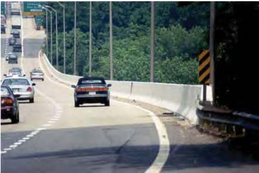
Figure 7-5. 1,067-mm [42-in.] Tall Concrete Safety-Shaped Bridge Railing
