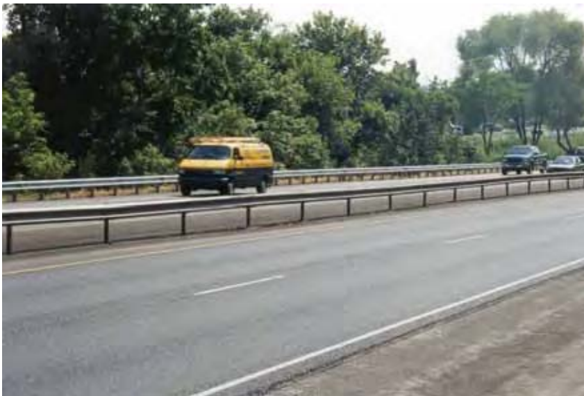
Figure 6-2. Weak-Post W-Beam Median Barrier
