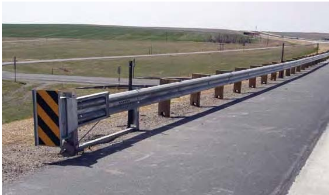
Figure 8-12. Extruder Terminal (ET-Plus™)
