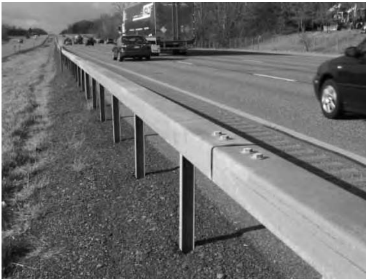
Figure 6-9. Box-Beam Median Barrier
