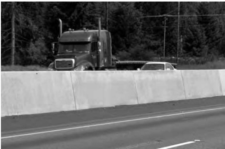
Figure 5-20. Constant Slope Barrier
