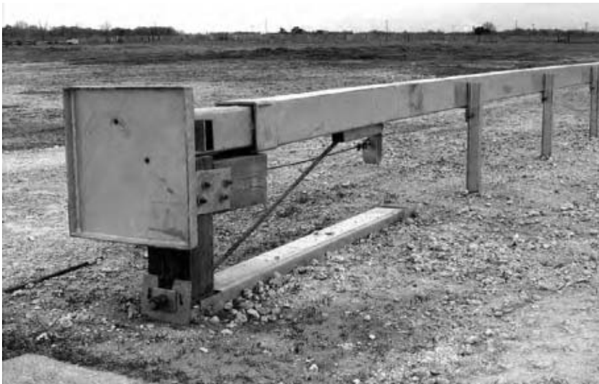
Figure 8-18. Wyoming Box-Beam End Terminal (WY-BET™)
