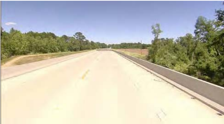
Figure 7-4. Concrete F-Shaped Bridge Railing
