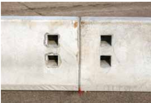
Figure 9-13. Quick-Bolt F-Shaped Concrete Safety Barrier
