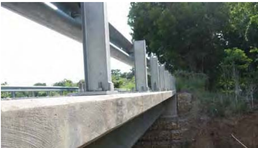
Figure 7-2. Texas T-6 Railing
