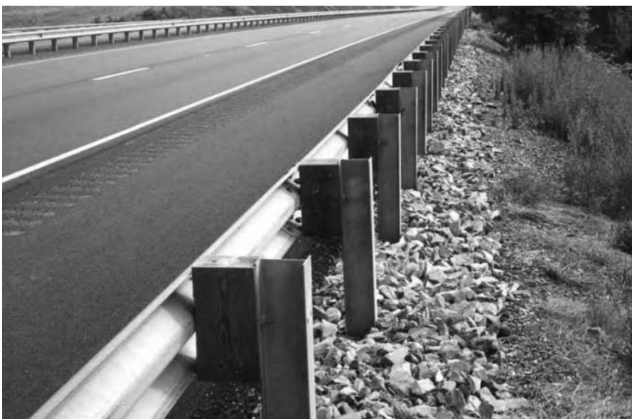
Figure 5-9. Steel-Post W-Beam Guardrail with Wood Blockouts
