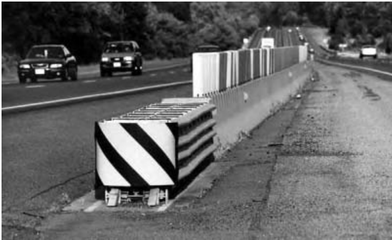
Figure 8-29. Trinity Attenuating Crash Cushion (TRACC™)
