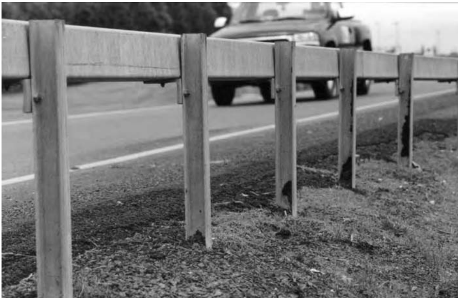
Figure 5-8. Weak-Post Box Beam Guardrail
