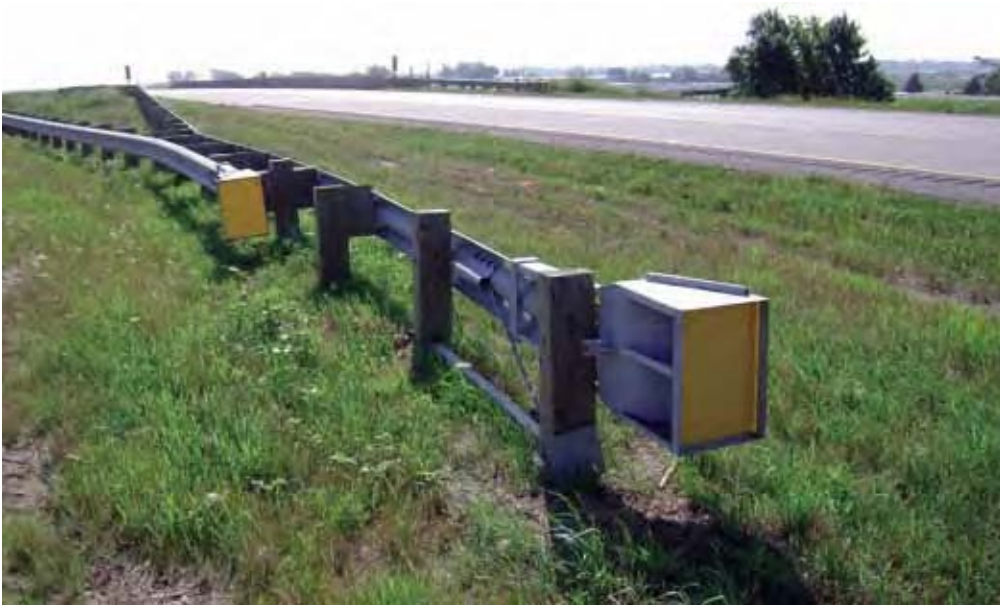
Figure 8-16. FLEAT Median Terminal (FLEAT-MT™)
