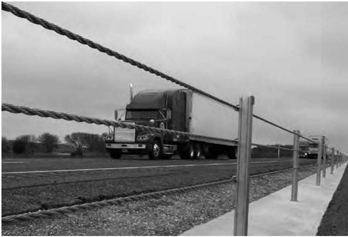
Figure 6-8. Gibraltar Cable Barrier System
