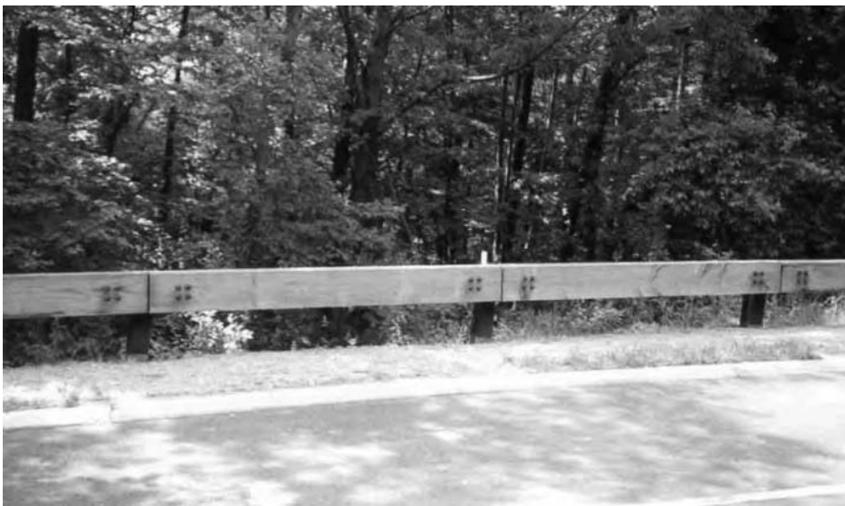
Figure 5-17. Merritt Parkway Aesthetic Guardrail
