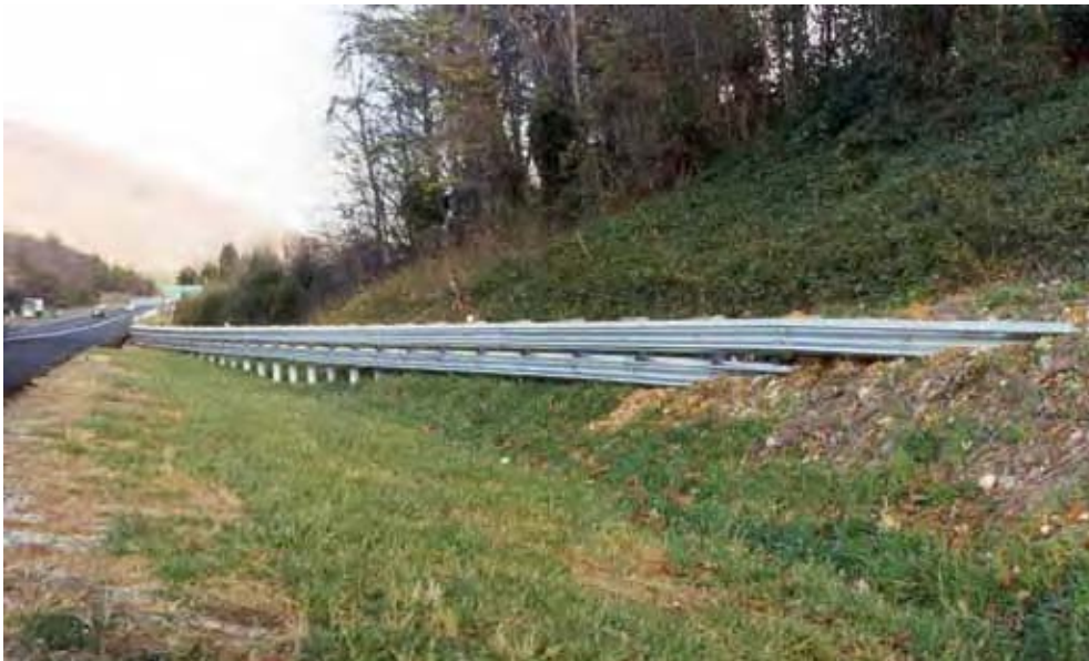
Figure 8-6. W-Beam Guardrail Anchored in Backslope
