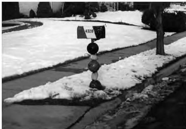
Figure 11-2. Examples of Hazardous Single Mailbox Installations
