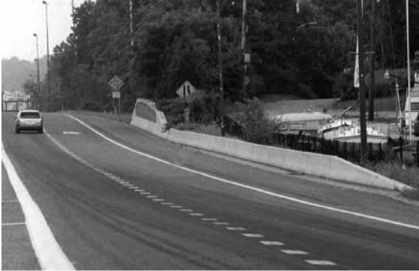
Figure 8-43. Sloped Concrete End Treatment
