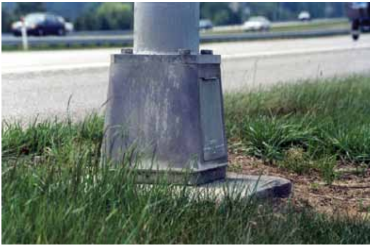
Figure 4-11. Example of a Cast Aluminum Frangible Luminaire
