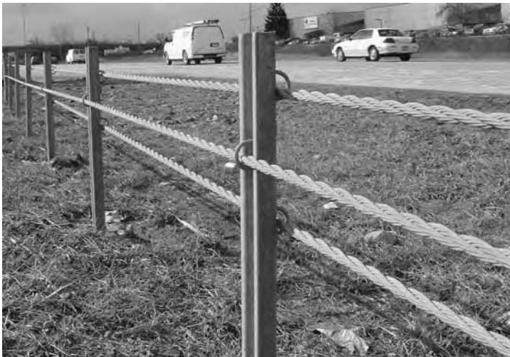
Figure 6-6. NU-CABLE™ High-Tension Cable System
