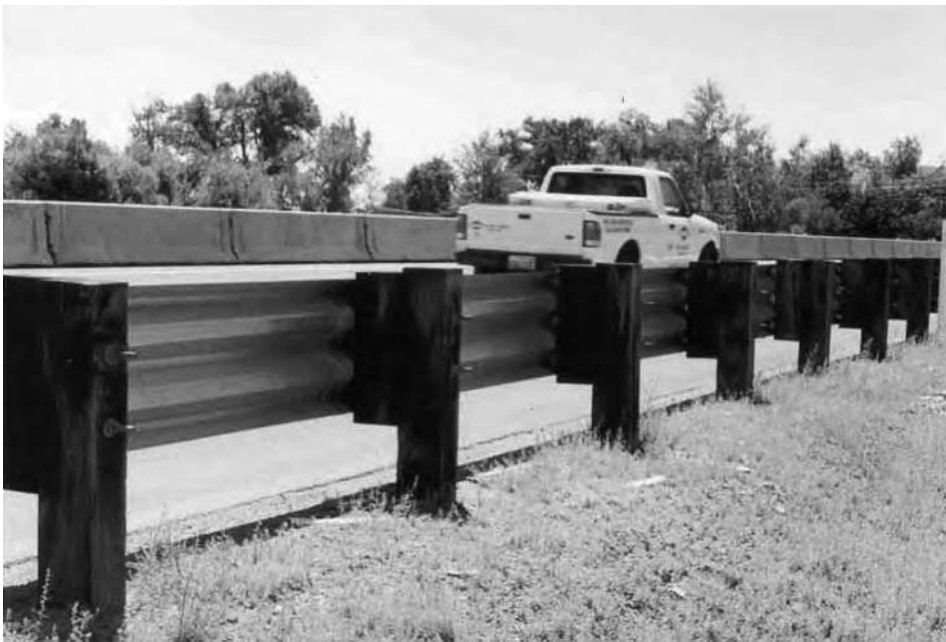
Figure 5-14. Wood-Post Thrie-Beam Guardrail
