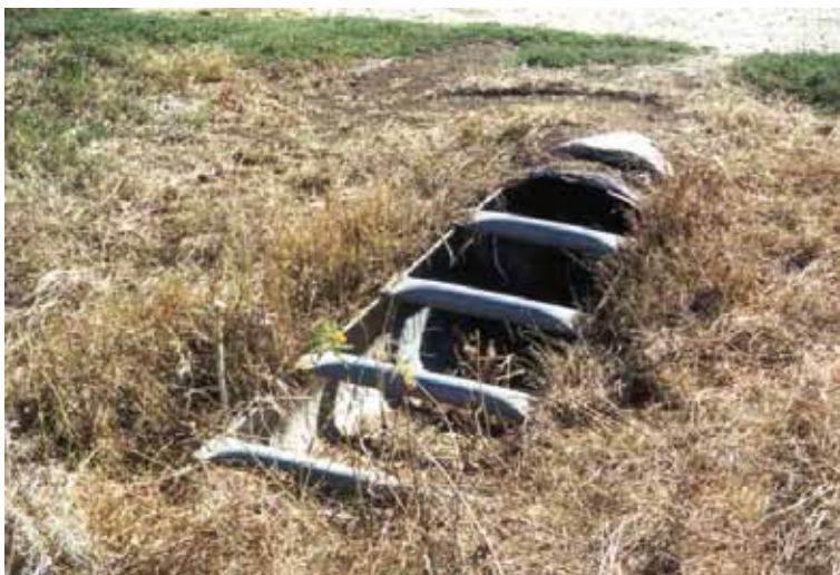
Figure 3-12. Safety Treatment for Parallel Drainage Pipe
