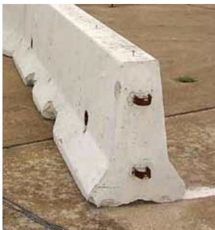
Figure 9-1. Iowa Temporary Concrete Barrier
