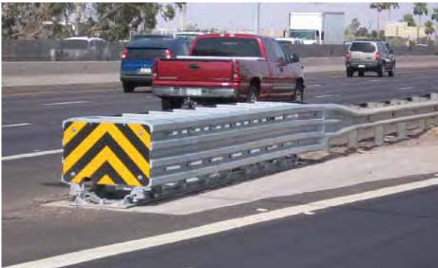
Figure 8-37. Smart Cushion Innovations (SCI-100GM) Crash Cushion
