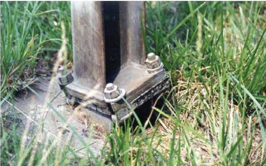
Figure 4-8. Unidirectional Slip Base for Small Signs
