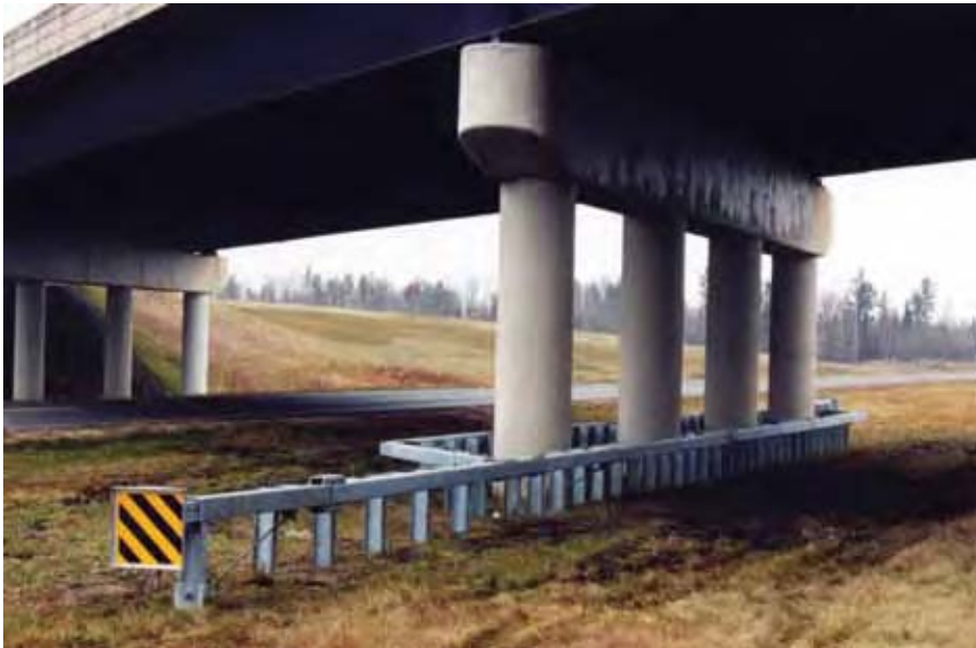
Figure 8-24. Bursting Energy Absorbing Terminal–Bridge Pier (BEAT-BP™) System
