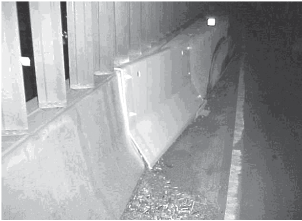
Figure 9-23. Portable Concrete Barrier Steel Plate Transition
