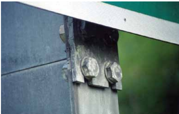
Figure 4-6. Slotted Fuse Plate Design
