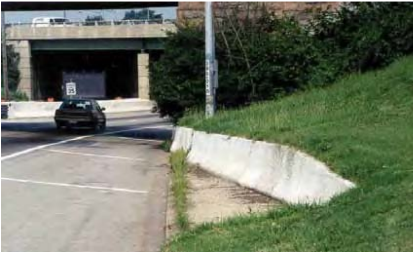
Figure 8-44. Barrier Anchored in Backslope
