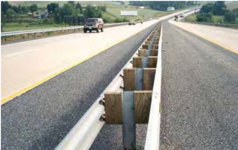
Figure 6-10. Strong-Post W-Beam Median Barrier
