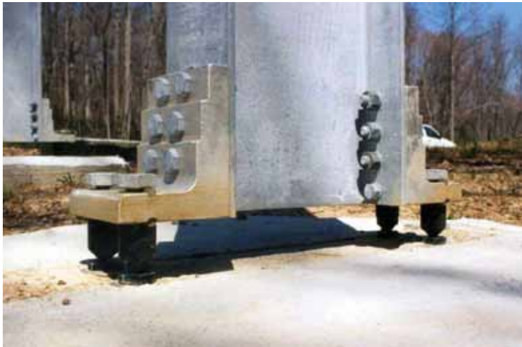
Figure 4-4. Multidirectional Coupler
