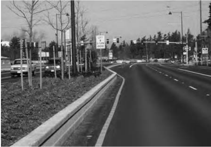
Figure 5-19. Low Profile Barrier
