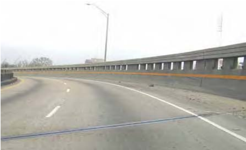
Figure 7-6. Texas Type TT Railing
