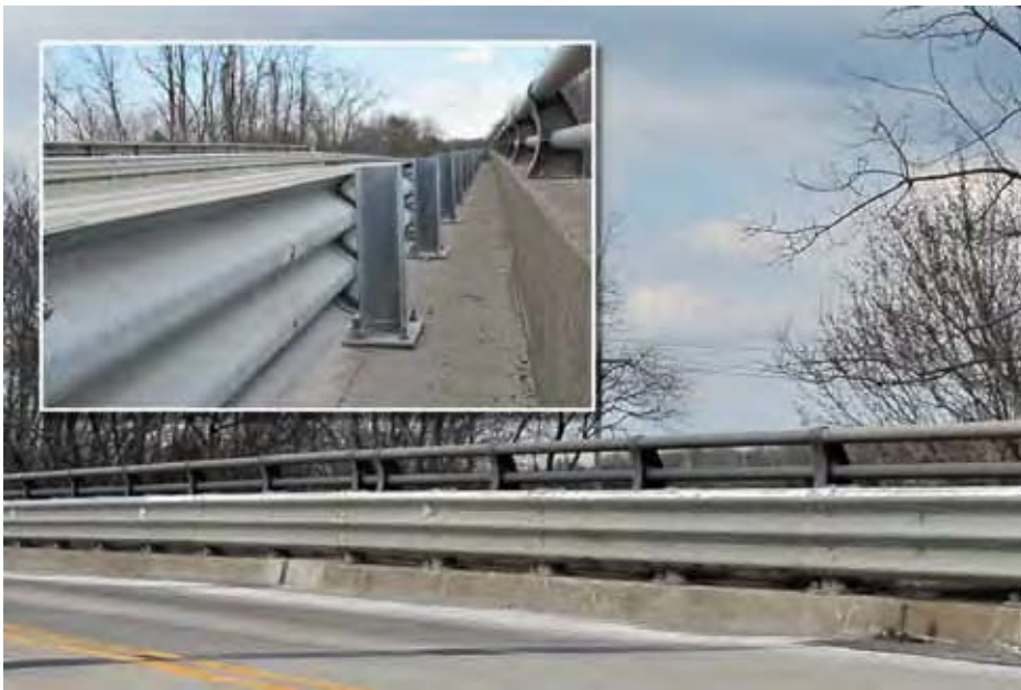
Figure 7-10. Delaware Thrie-Beam Retrofit
