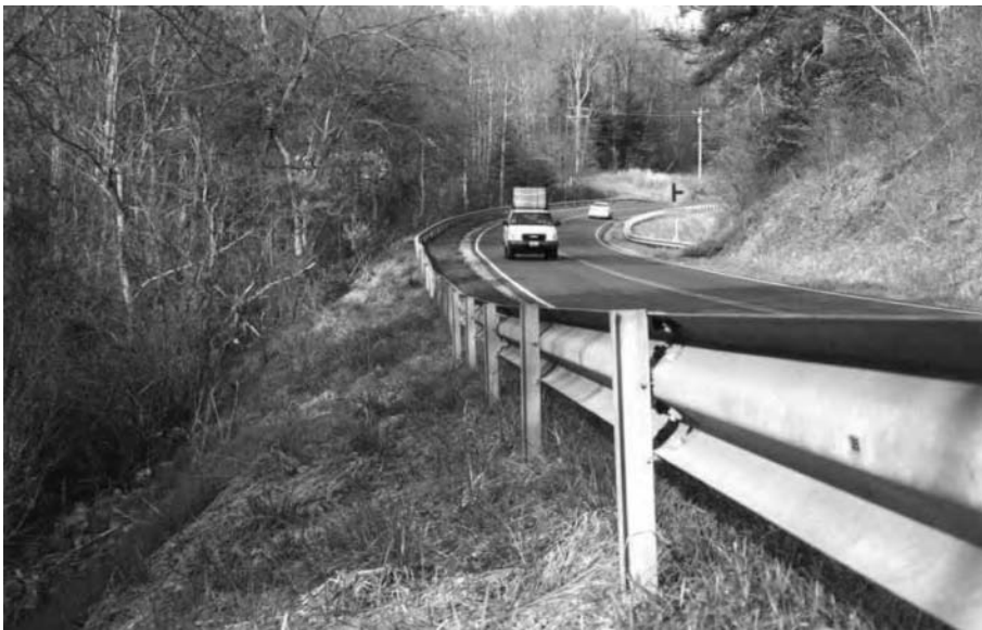
Figure 5-6. Weak-Post W-Beam Guardrail
