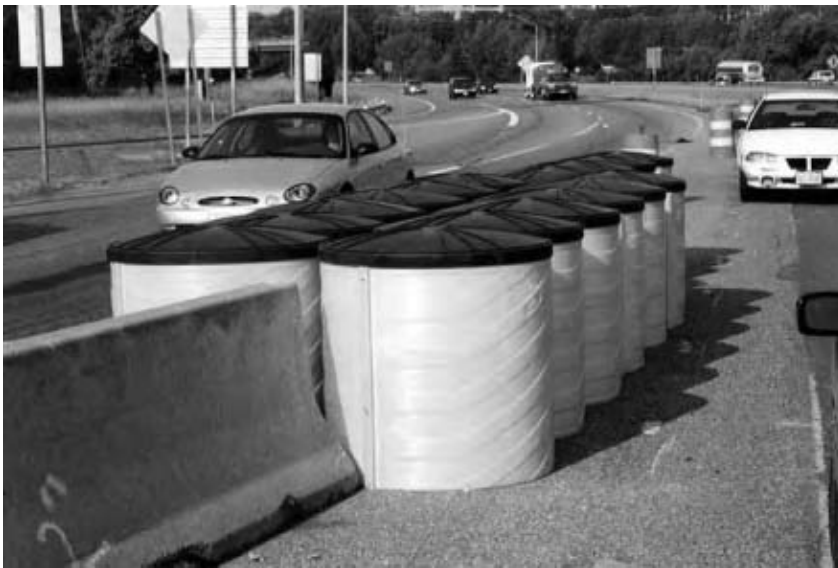
Figure 8-39. The Fitch Universal Barrel®
