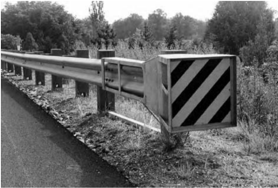
Figure 8-13. Sequential Kinking Terminal (SKT-350™)
