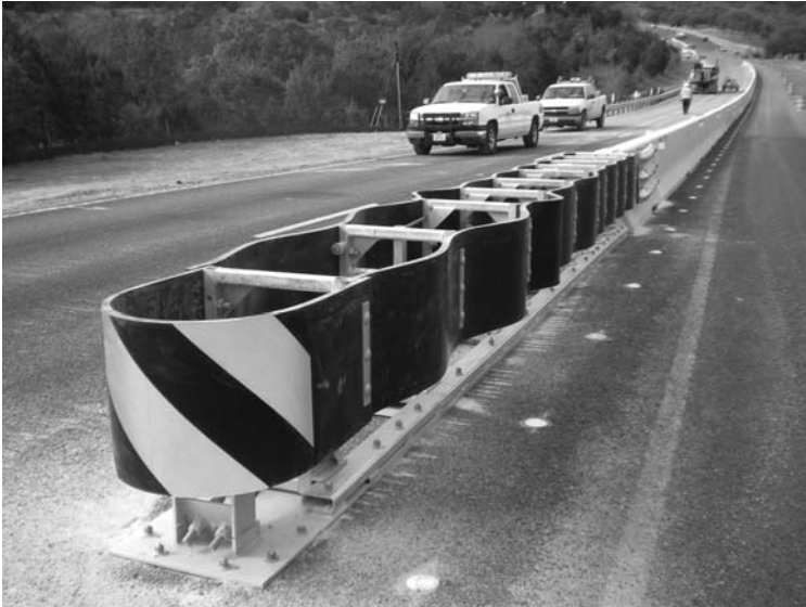
Figure 8-33. Hybrid Energy Absorbing Reusable Terminal (HEART™)
