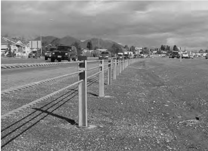
Figure 6-5. The Cable Safety System (CASS)
