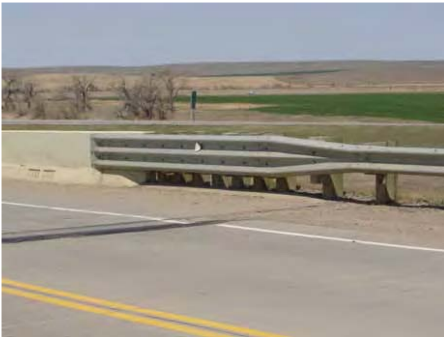
Figure 7-12. Thrie-Beam Transition to Modified Concrete Safety Shape
