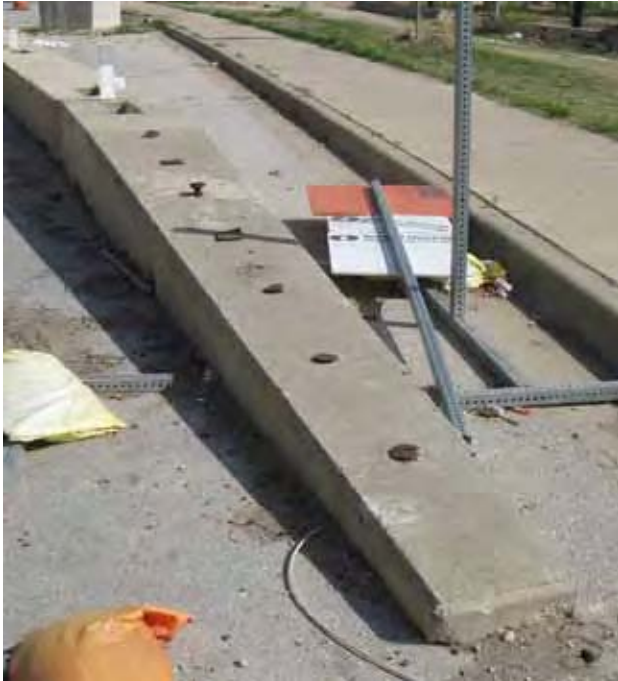
Figure 9-22. Slope-End Treatment for Low-Profile Portable Concrete Barrier
