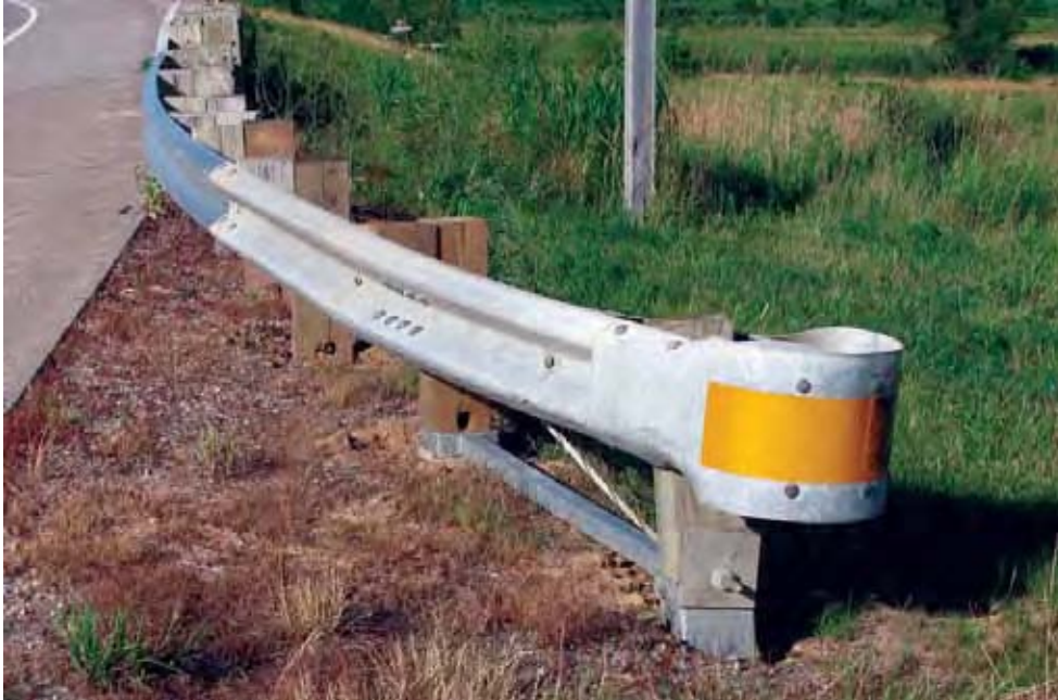
Figure 8-8. Modified Eccentric Loader Terminal (MELT)
