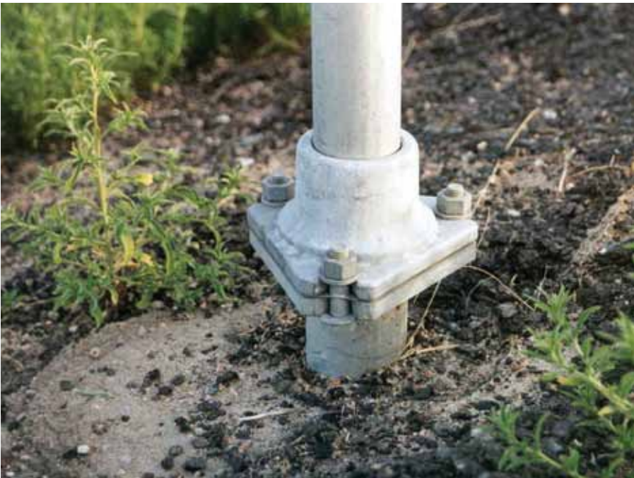
Figure 4-9. Multidirectional Slip Base for Small Signs
