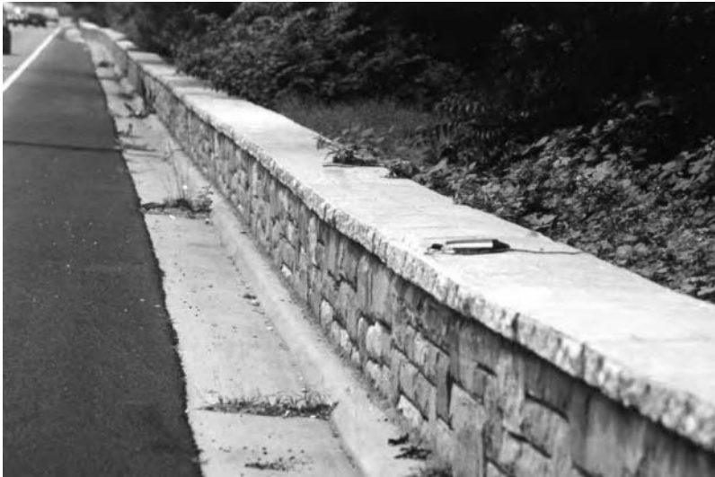
Figure 5-24. Precast Masonry Wall
