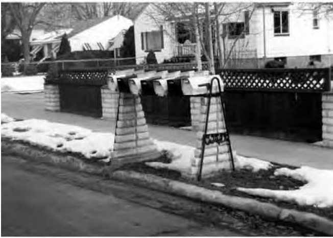
Figure 11-3. Examples of Hazardous Multiple Mailbox Installations
