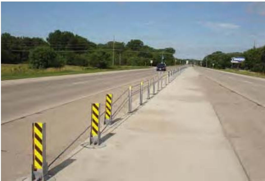
Figure 8-5. CASS™ Cable Terminal (CCT)
