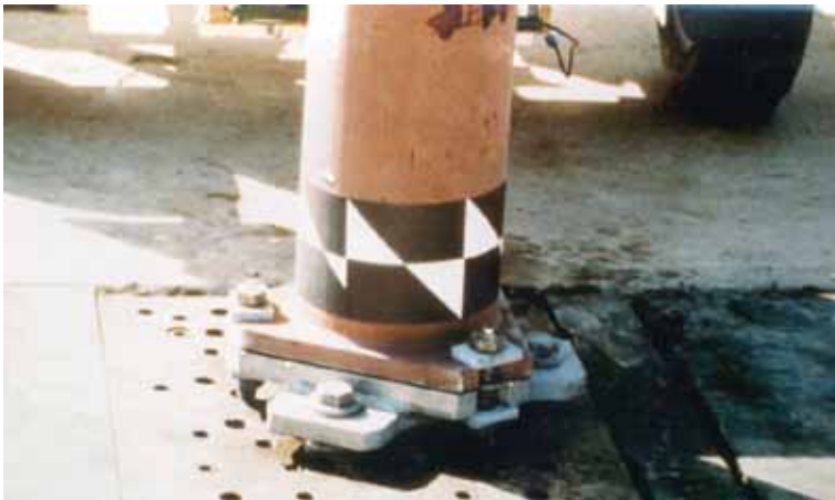
Figure 4-12. Example of a Luminaire Slip Base Design
