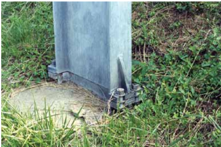
Figure 4-5. Typical Unidirectional Slip Base
