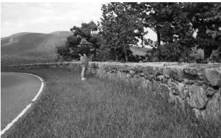
Figure 5-23. Stone Masonry Wall
