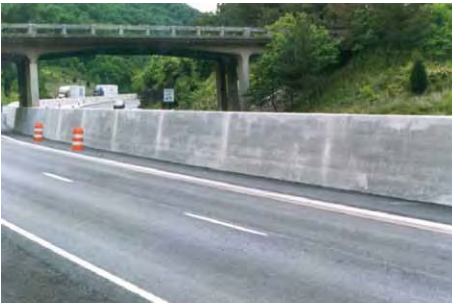
Figure 6-14. Single-Slope Concrete Median Barrier
