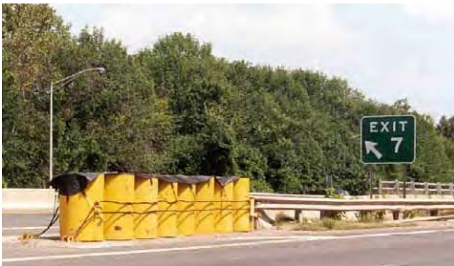
Figure 8-26. Narrow Connecticut Impact Attenuation System (NCIAS)
