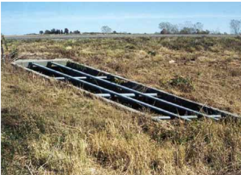
Figure 3-9. Safety Treatment for Cross-Drainage Culvert
