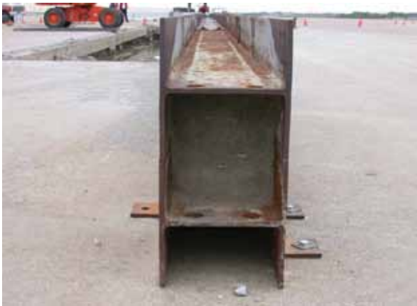
Figure 9-12. Iowa DOT Tie-Down Steel H-Section Temporary Barrier
