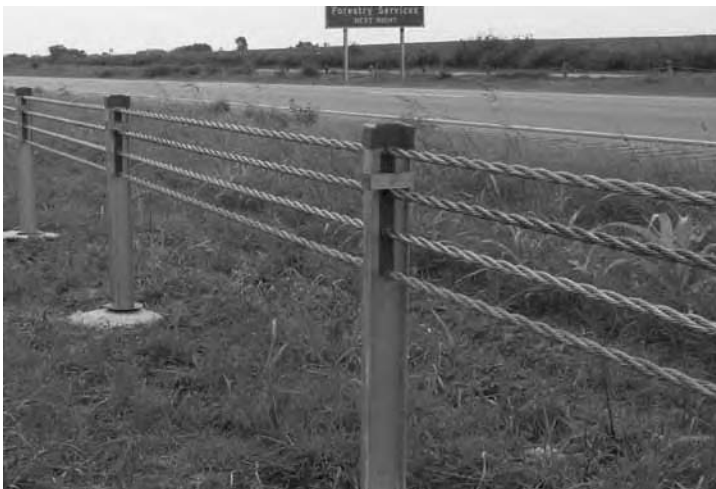
Figure 6-7. Safence Cable Barrier System
