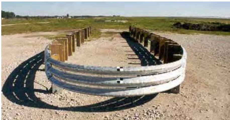
Figure 8-20. Bullnose Guardrail System
