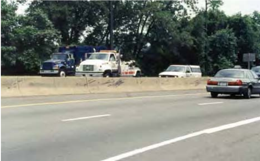
Figure 6-13. Concrete Safety-Shape Median Barrier
