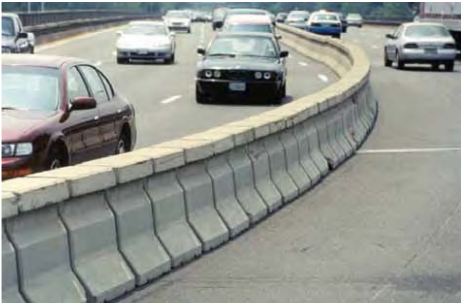
Figure 6-15. Standard Quickchange® Moveable Barrier System
