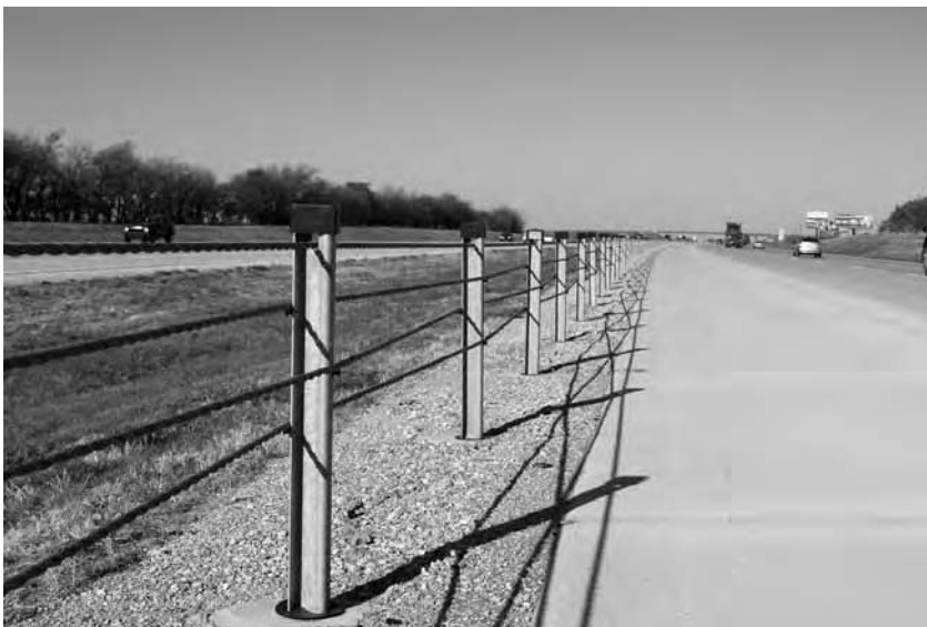
Figure 6-4. Brifen Wire Rope Safety Fence
