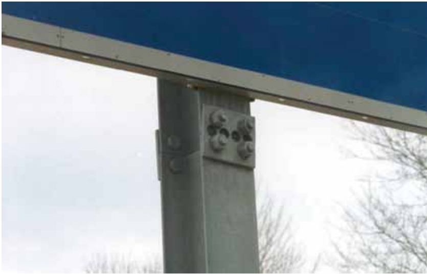
Figure 4-7. Perforated Fuse Plate Design
