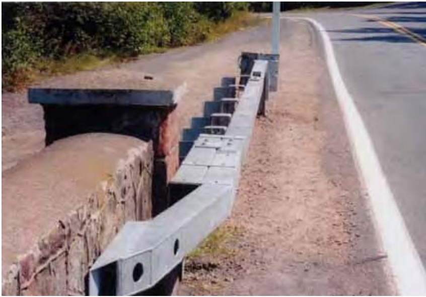
Figure 8-23. Bursting Energy Absorbing Terminal–Single Sided Crash Cushion (BEAT-SSCC™) System
