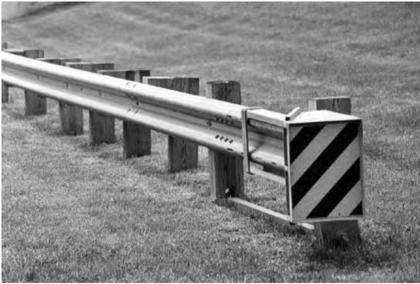
Figure 8-9. Flared Energy-Absorbing Terminal (FLEAT™)
