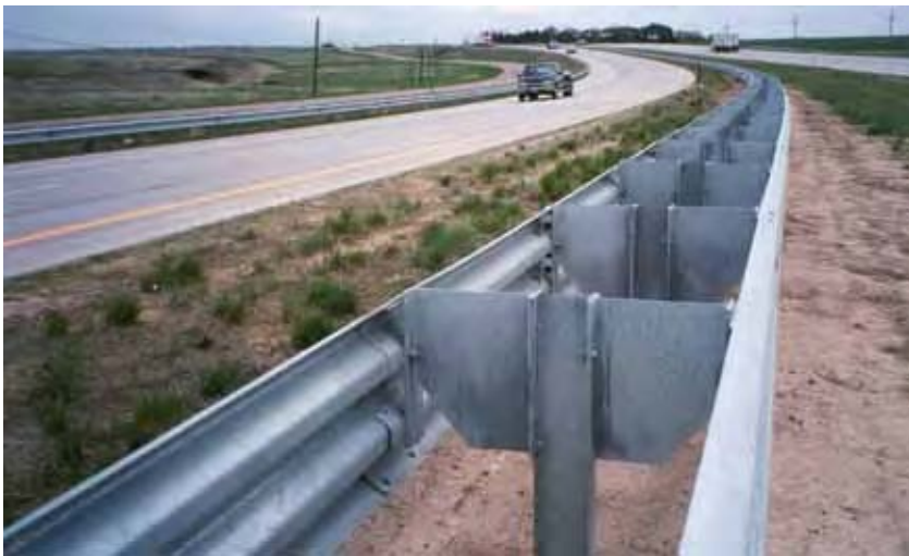
Figure 6-11. Modified Thrie-Beam Median Barrier
