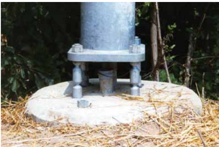
Figure 4-13. Example of a Frangible Coupling Design
