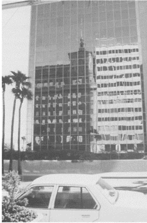
Plate 7.2 The glass façade of an office building in Phoenix AZ, reflects the architectural style of the late modern period
