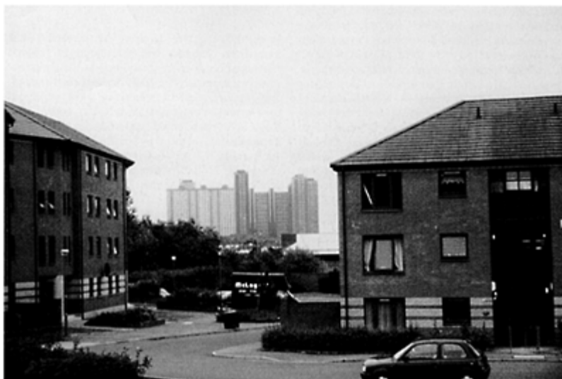
Plate 11.2 The thirty-one-storey Red Road tower blocks erected in Glasgow in the 1960s were designed to house 4,000 people at an average density of 180 persons per acre (440 per hectare). The newly built ‘tenements’ in the foreground reflect the more recent response to meeting public-housing needs through the activities of housing associations
