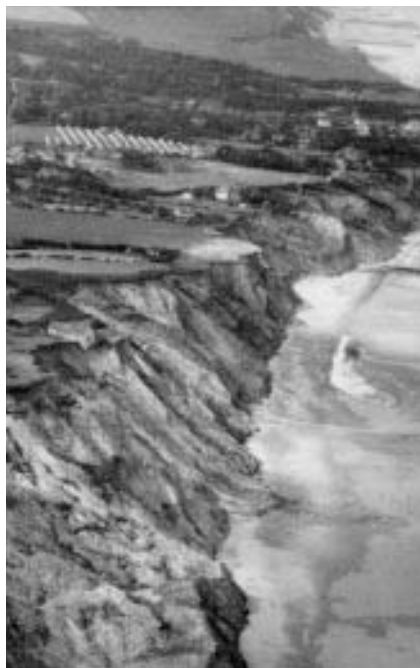
Figure 1.9 The only solution to saving buildings built near eroding coastlines may be to move them lock, stock and barrel to a site further inland. Here, the cliff edge has reached the building at the centre left of the photograph. A number of other buildings further up the coastline are also at risk
