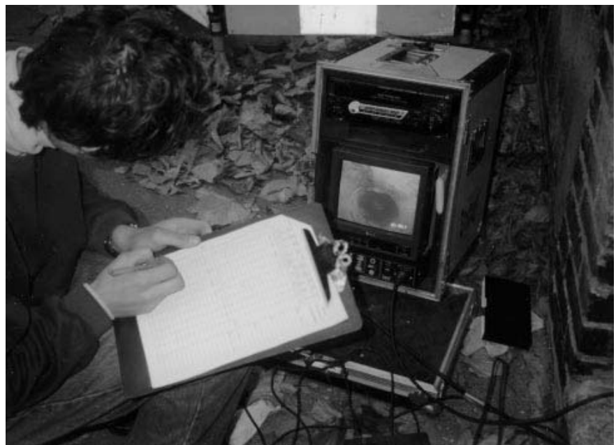
Figure 4.19 CCTV inspection of a drain
