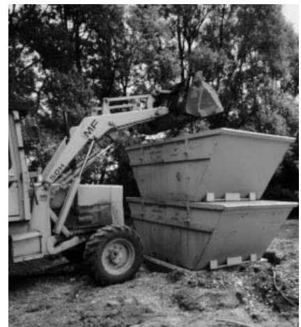
Figure 2.5 A simple loading test in progress to assess the effectiveness of vibro treatment
