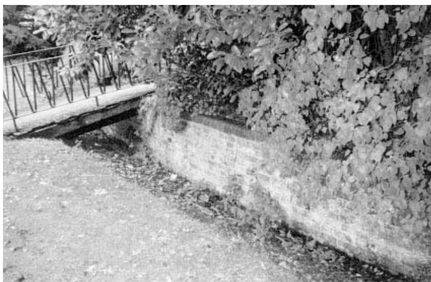
Figure 5.2 The ha-ha on the BRE site at Garston used for assessing the performance of brickwork in aggressive conditions
