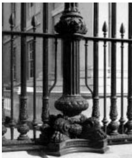
Figure 5.22 Decorative cast iron railings at the British Museum
