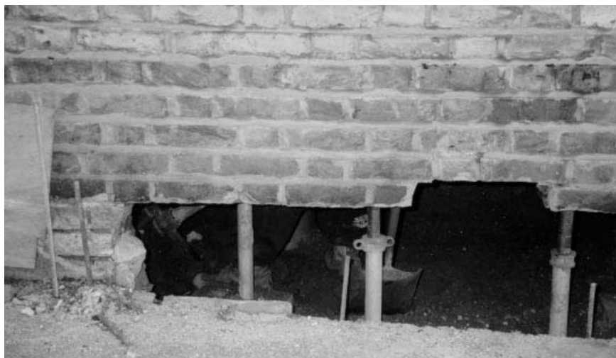
Figure 2.18 A section of an external one-brick wall removed to accommodate the toe of the floor slab
