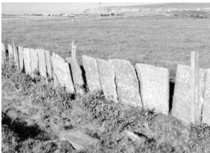
Figure 0.18 Caithness flags used to form a fence. The slabs were not sufficiently high to be stock-proof
