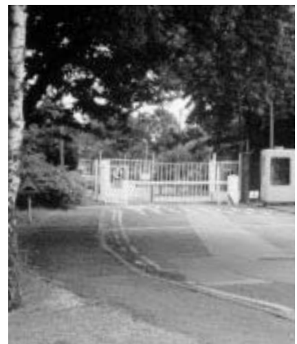
Figure 5.28 Controlled access vehicle and pedestrian gates in steel bar and tube with bracing in sheet steel
