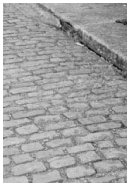
Figure 6.6 Coursed stone setts laid to camber
