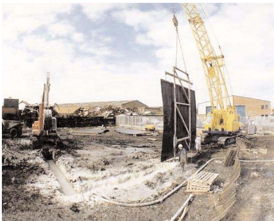
Figure 1.16 Installation of an impermeable membrane into a contamination containment system at a brownfield site
