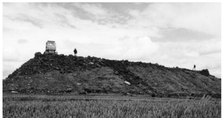
Figure 2.6 Surcharging poor ground prior to the development of a site
