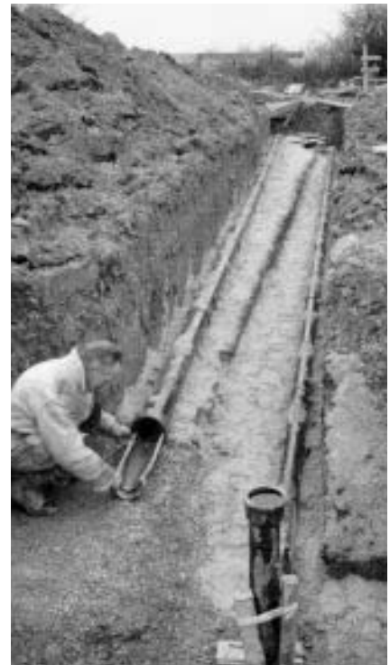
Figure 4.13 Laying pitch fibre pipes in a common trench in 1960. The fittings are of cast iron
