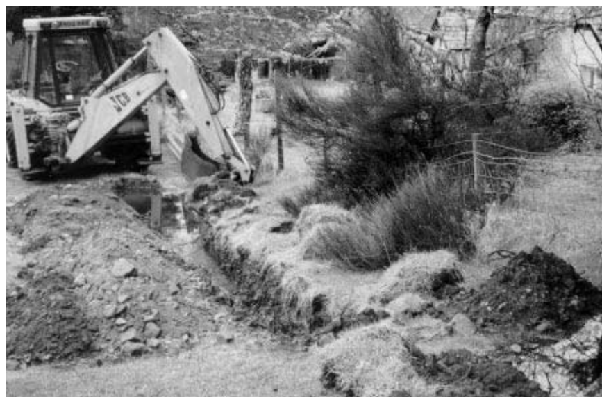
Figure 4.20 Excavating for a surface water drain
