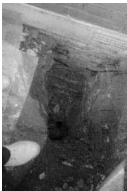
Figure 2.26 A narrow diameter hole has been excavated in a confined space alongside a one brick solid external wall to establish the depth and width of what turned out to be brick footings. Both depth and width had to be established by probing with a long crowbar. The footings were on shrinkable clay, and were unusually deep for an Edwardian house. Tree roots are visible in the sides of the excavation
