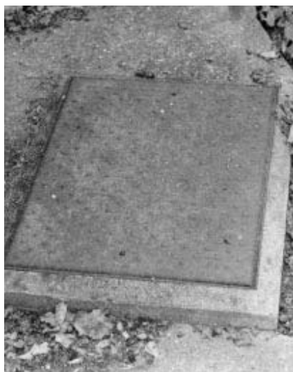
Figure 4.16 A 10 year old steel manhole cover
