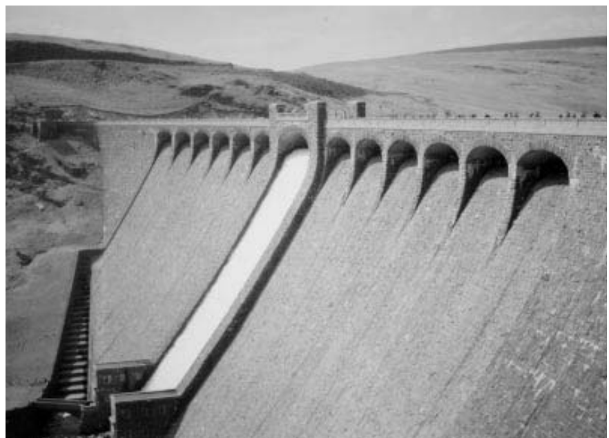
Figure 0.19 The dam at one of the Elan Valley reservoirs from which Birmingham takes part of its water requirements
