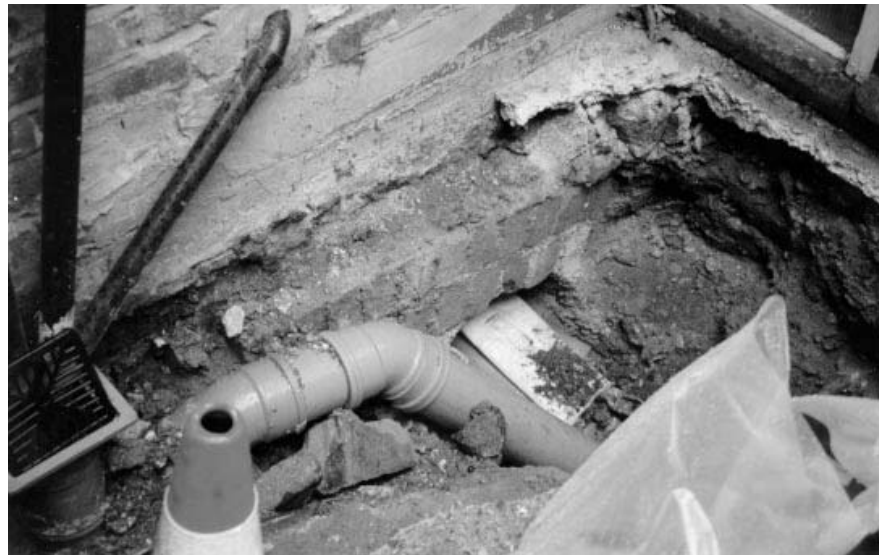
Figure 4.12 PVC drain pipes being laid as replacements for salt glazed pipes cracked as a result of movements of the shrinkable clay ground
