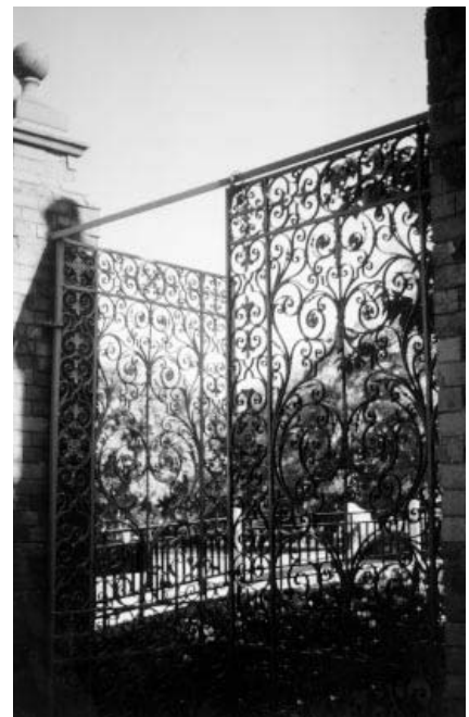
Figure 5.27 A pair of wrought iron gates made for a country house by a skilled blacksmith around 1910. Although wrought iron is reasonably durable, unless gates of this kind are regularly maintained, they will gradually deteriorate. The main problem is corrosion of the inside surfaces of the bands which hold adjacent scrolls together
