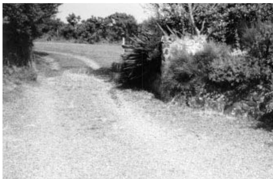
Figure 6.9 A domestic driveway consisting of a hard binding gravel base dressed with fine gravel
