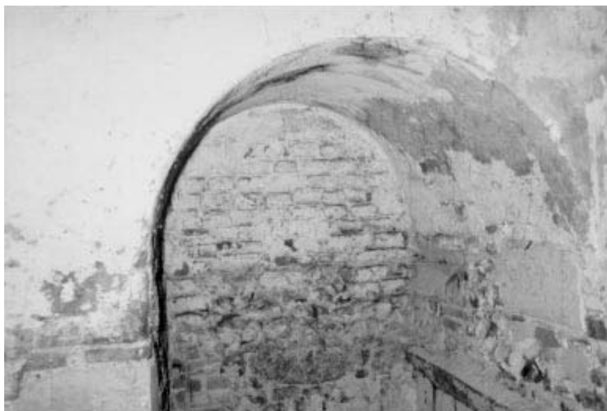
Figure 3.9 In spite of the mixture of materials in this domestic cellar, no structural distress is apparent
