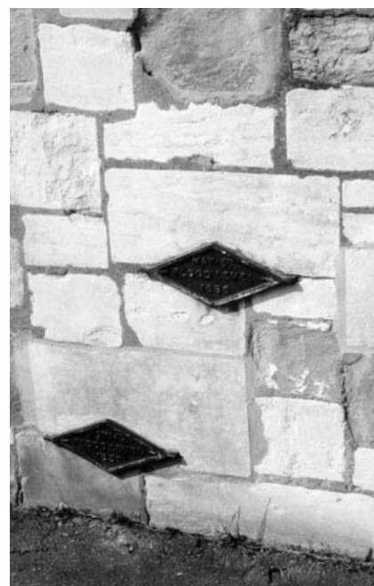
Figure 1.23 Flood level depth tablets at Upton-upon-Severn
