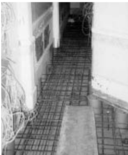
Figure 2.17 Reinforcement in place before casting the floor slab
