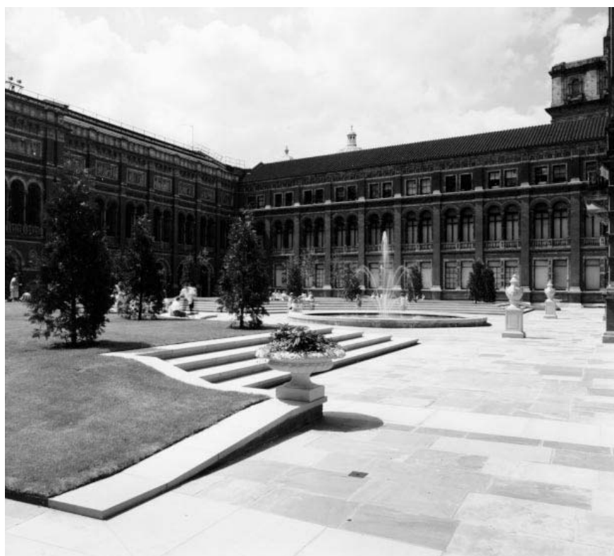
Figure 6.1 The York stone paved courtyard of the Victoria and Albert Museum
