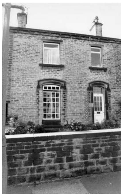
Figure 5.14 A low boundary wall to a front garden in Yorkshire, adjoining a public pavement and built in a similar stone to that of the house
