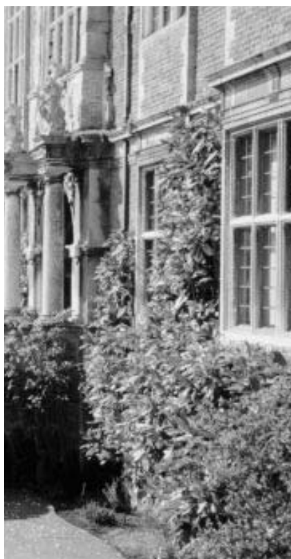
Figure 6.17 Climbing plants should be cut back and trimmed to ensure that they do not have any detrimental effect on the building fabric
