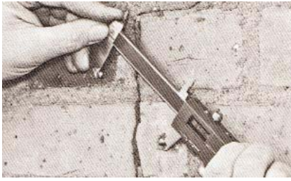
Figure 2.11 Crack measurement using brass screws
