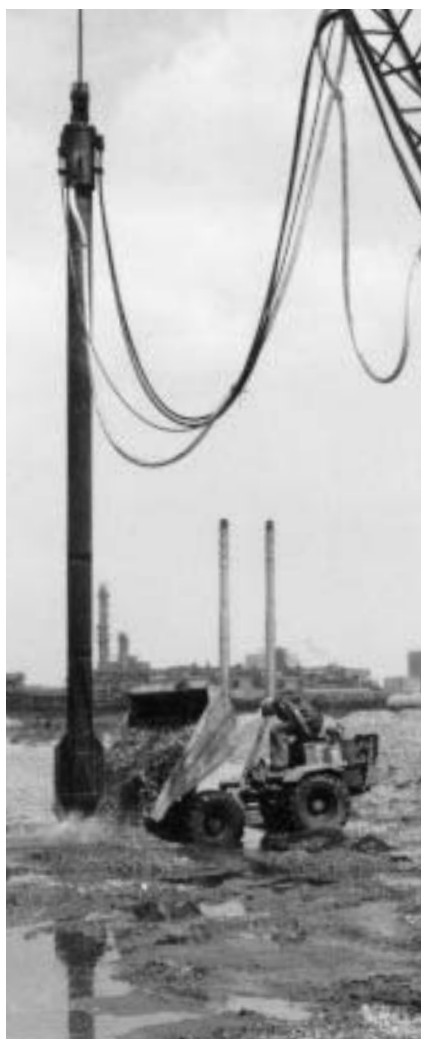
Figure 2.4 Vibro stone column ground improvement
