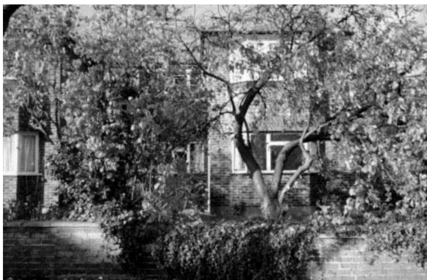
Figure 1.29 Trees are often considered a valuable amenity to be protected, but they may affect the stability of buildings if they are too close to them
