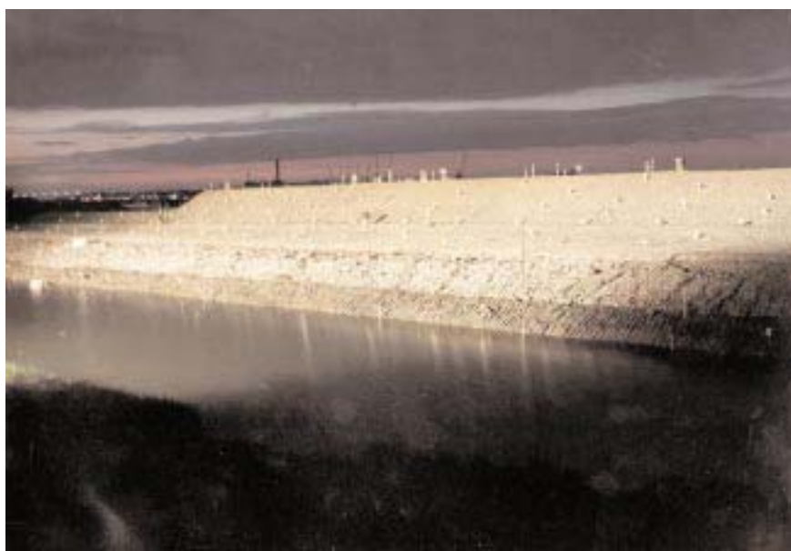
Figure 1.20 River flood protection embankment
