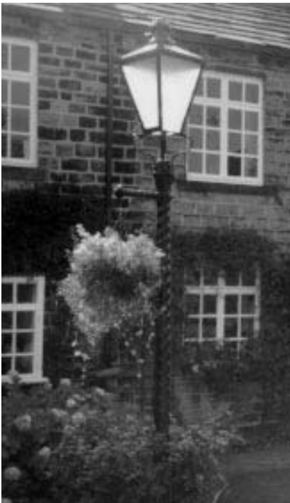
Figure 5.37 An old gas street lighting column and lantern has been adapted to illuminate this pedestrian access. The horizontal bar was to support the top of the lamplighter’s ladder
