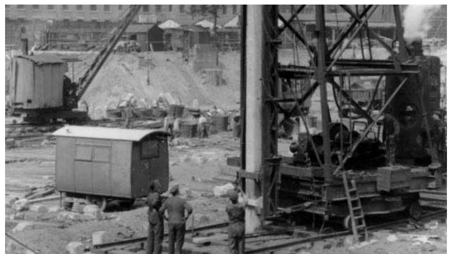
Figure 0.11 A steam piling rig being used for driving concrete piles in the 1930s. Heads of driven piles can be seen, but the remains of broken piles litter the site
