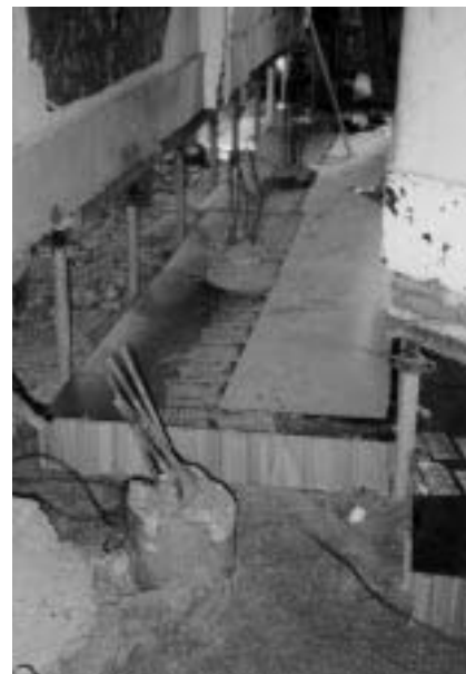
Figure 2.16 Deformable packing being inserted between the piles to carry the reinforced concrete floor slab. On each side of the photograph, jacks support the internal partitions
