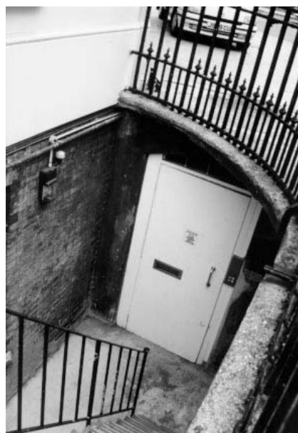
Figure 3.28 Access to this basement is provided from street level independently of the dwelling above
