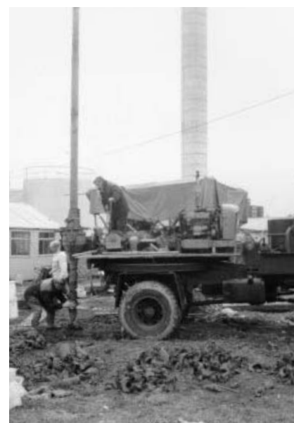
Figure 2.39 A lorry-mounted boring rig in operation in 1970
