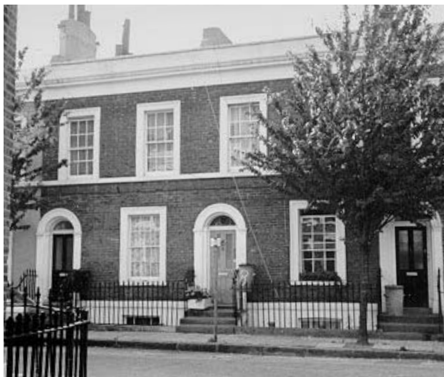
Figure 3.29 No access from street level is provided to these basements from the fronts of the dwellings
