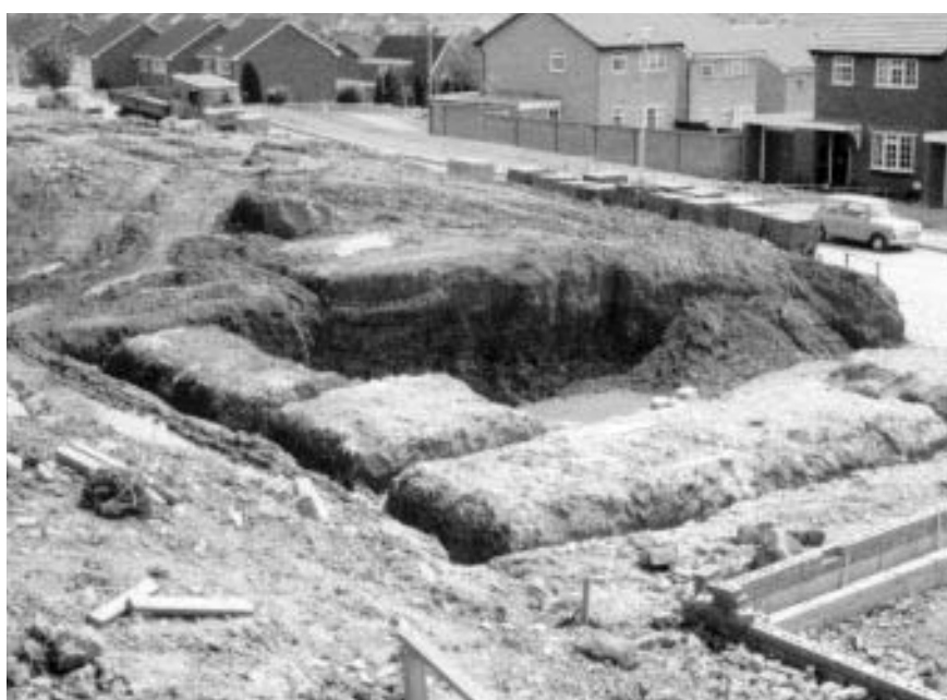
Figure 2.1 Adequate foundations are crucial to the stability of even the smallest of buildings. Here, a sloping site of disturbed ground has given rise to a number of awkward problems for the contractor
