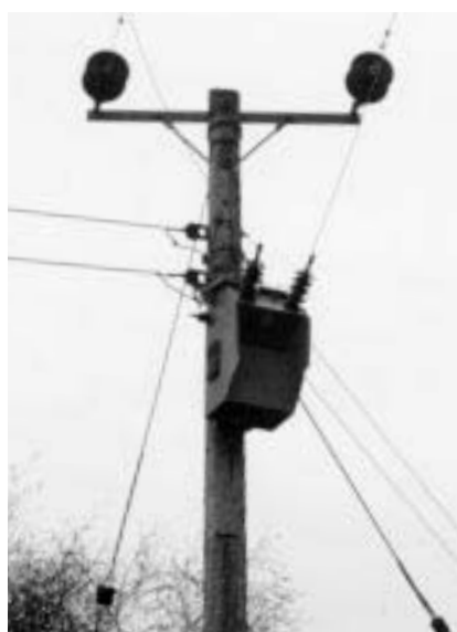
Figure 4.27 Electricity cables to rural locations are normally of the overhead kind. Responsibility for adequate and safe performance normally lies with the utility company
