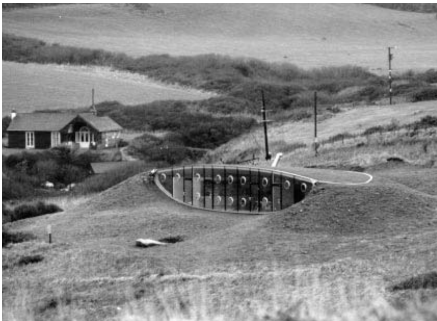
Figure 3.31 An underground house near the Pembrokeshire coast
