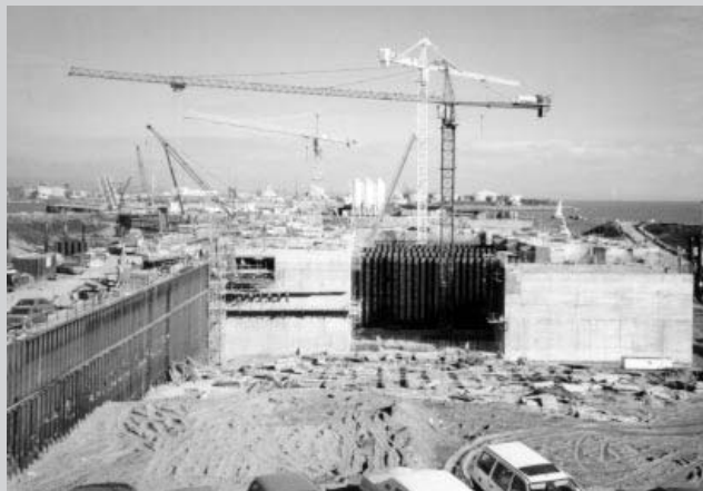
Figure 3.17 The main locks of the Cardiff Bay barrage under construction
