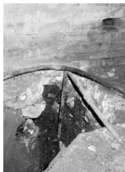
Figure 4.28 Rehabilitation work under way on a Victorian house. Excavation has been used to find the routes of the old services installations
