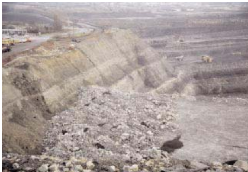
Figure 1.17 Backfilling of a deep opencast quarry. The 'high-wall' will present potential problems of differential settlement once the site has been developed
