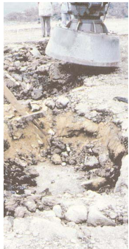
Figure 2.3 Close-up of the footprint of the rapid impact compactor
