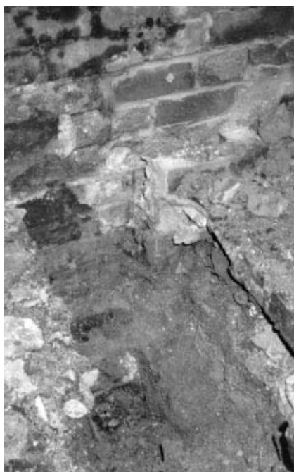
Figure 2.27 A variety of contaminants has obviously been in contact with this 100 year old clay brickwork below DPC level, but only minor damage has resulted. There is also evidence of previous alterations and some repointing
