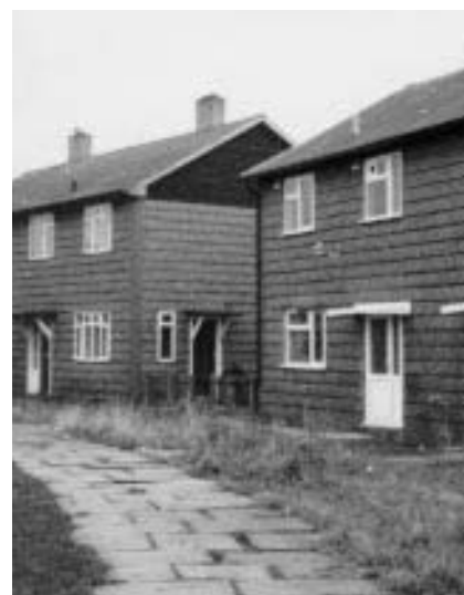
Figure 6.2 This concrete flag pavement was probably founded on inadequate bedding and now presents a considerable hazard for pedestrians
