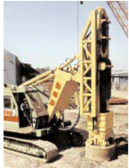
Figure 2.2 A rapid impact compactor
