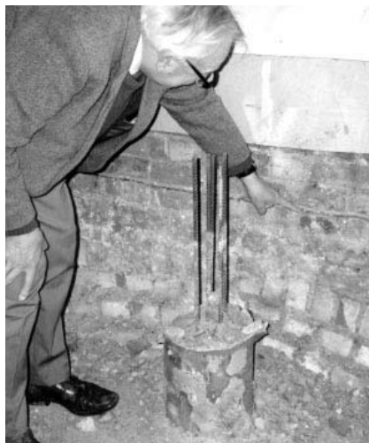
Figure 2.15 A pile adjacent to the separating wall. The DPC is being indicated. The original foundations were on piers of brickwork founded at approximately 2 m depth, bridged by brick arches spanning 2.5 m. One of these arches can be seen behind the pile reinforcement
