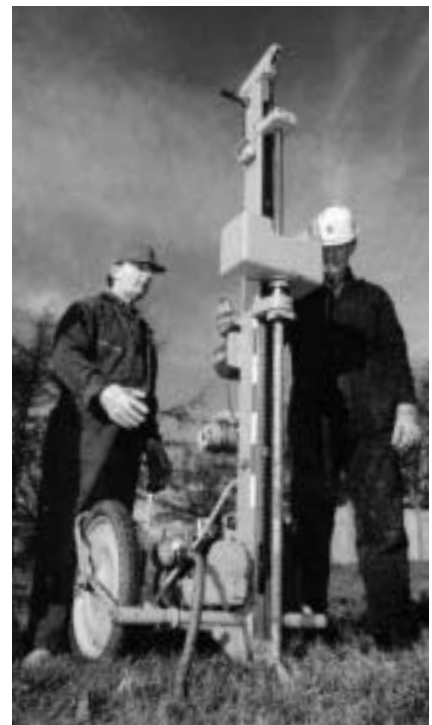
Figure 1.10 Soil conditions under test
