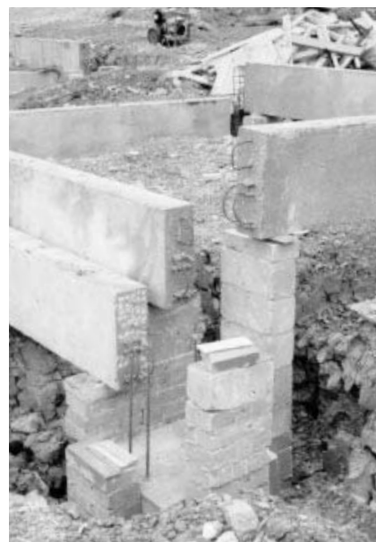
Figure 2.33 Ground beams being prepared for incorporation into pad foundations on a steeply sloping site
