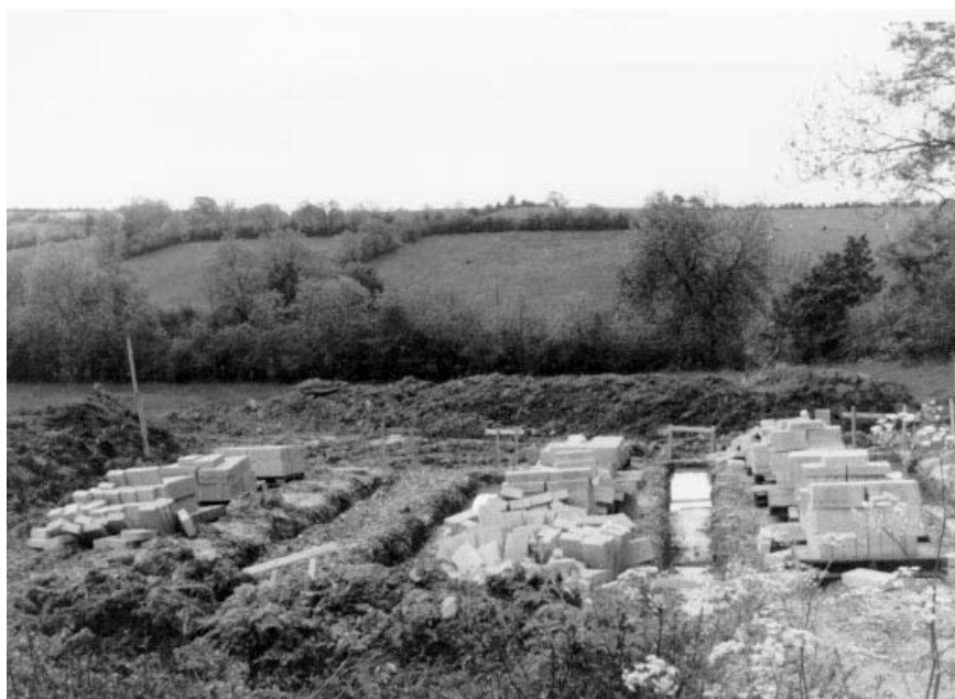
Figure 2.28 Concrete strip footings
