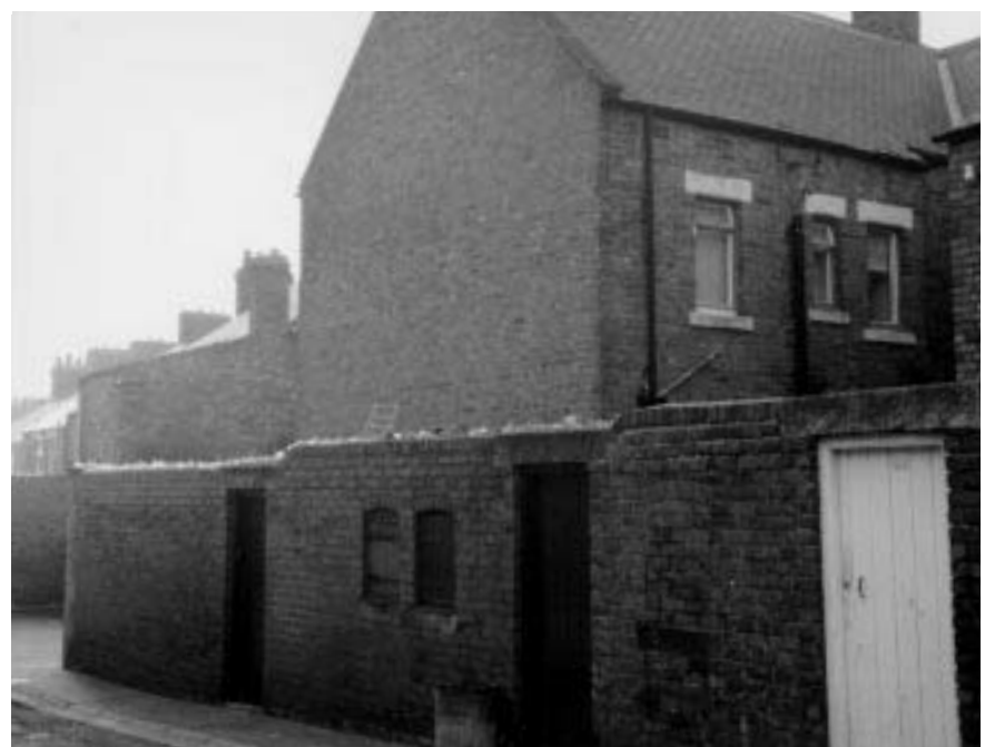
Figure 0.16 A recent defensive modification: broken glass set in mortar surmounts this freestanding brick perimeter wall
