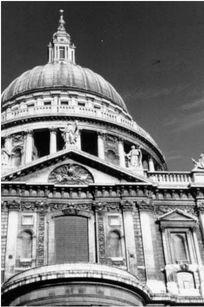
Figure 0.10 Masonry on the south transept of St Paul's Cathedral. It is said that these walls were founded on brick piers extending down to the gravel bed above the London Clay
