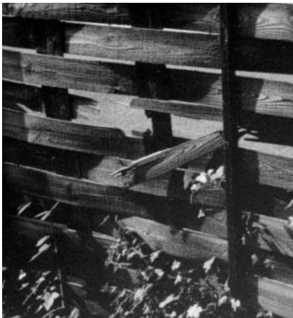
Figure 5.29 Forty year old woven wood fence panels, probably larch. Although rot-free, they become very brittle with time and are easily damaged
