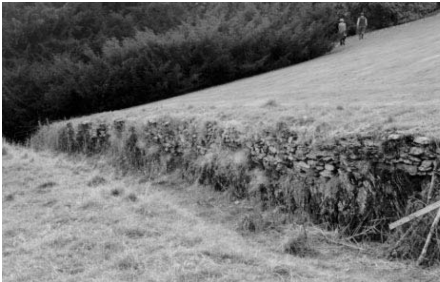
Figure 5.3 Excavation for this ha-ha has revealed a limestone seam to create a more-or-less vertical barrier to livestock
