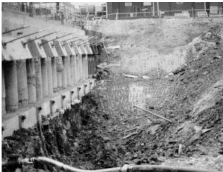
Figure 5.5 An anchored piled wall
