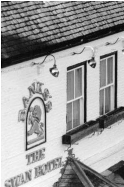
Figure 5.38 Swan-necked floodlight fittings on the Swan Hotel! The lighting arrangements here serve both commercial and amenity requirements
