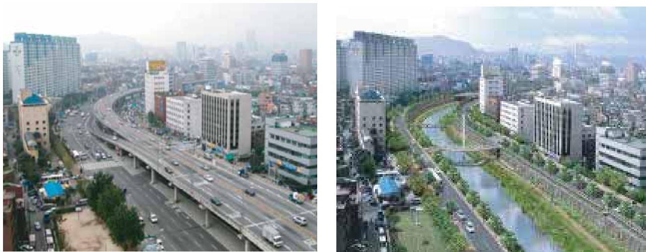
Figure 8 Restoration of Cheong Gye Cheon (before and after)
