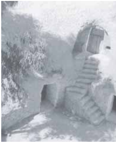
Source: Nick Baker and Koen Steemers, 2000, Energy and Environment in Architecture, Taylor & Francis.
