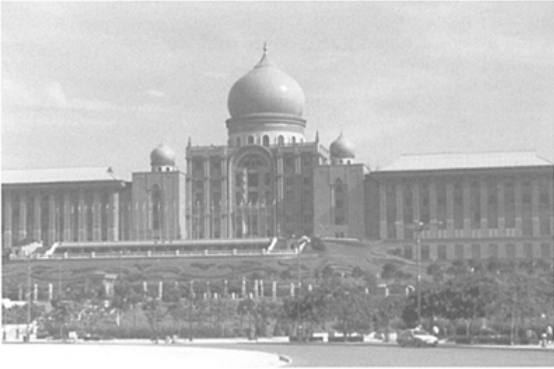
Figure 6.5 The Prime Minister's office at Putrajaya.
