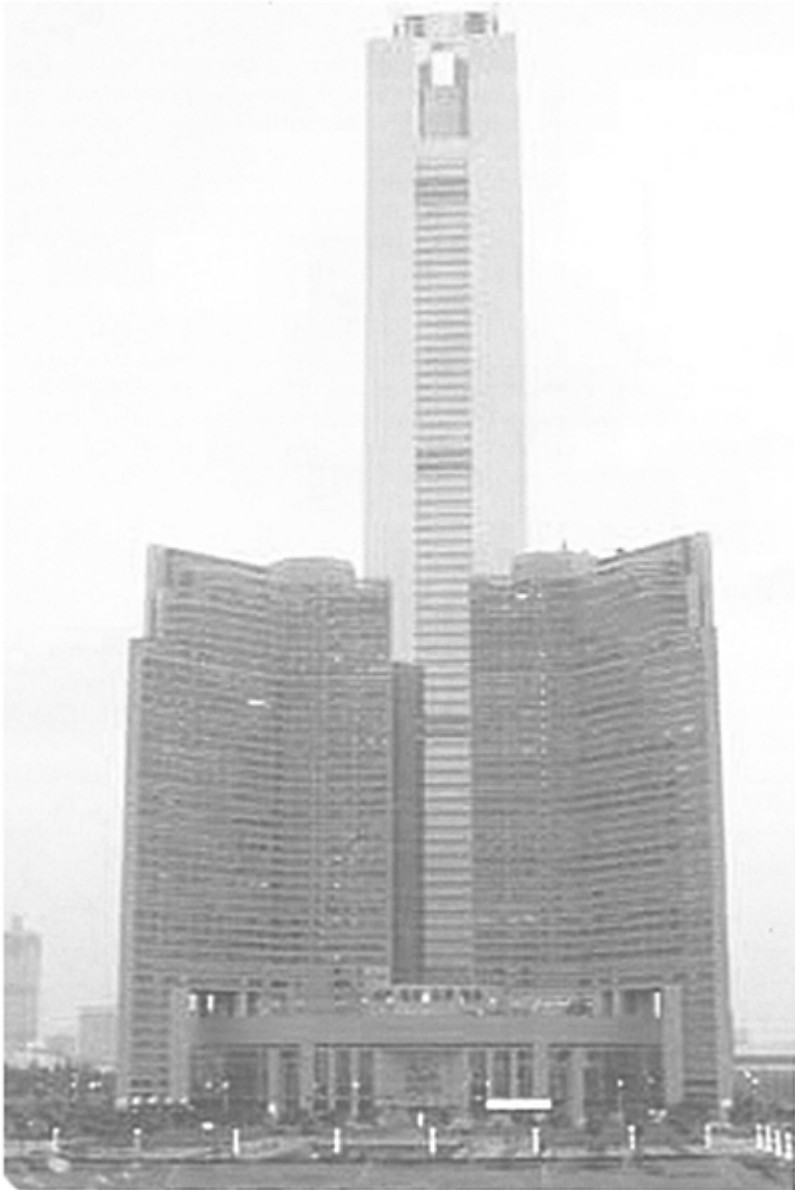
Figure 3.4 The Zhongxin Building is the most magnificent modern construction in Guangzhou dating from the late 1990s. It is one of the highest buildings in China, as high as 381 m.
