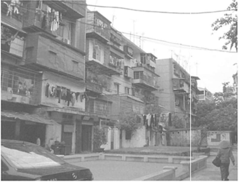
Figure 4.2 Popular housing for the poor: extensions to a block in KTT Kim Lien (photograph Hans Schenk).
