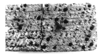
Figure 21.3 Hide beetle (*Dermestes ater*) damage to a Douglas fir roofing member
