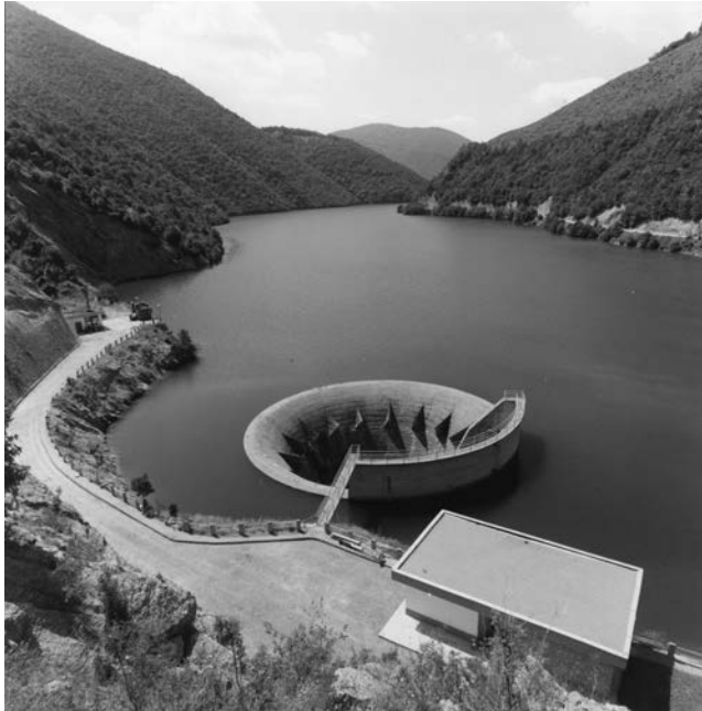
Figure 27.28 The shaft spillway of Globochica dam (Macedonia).
