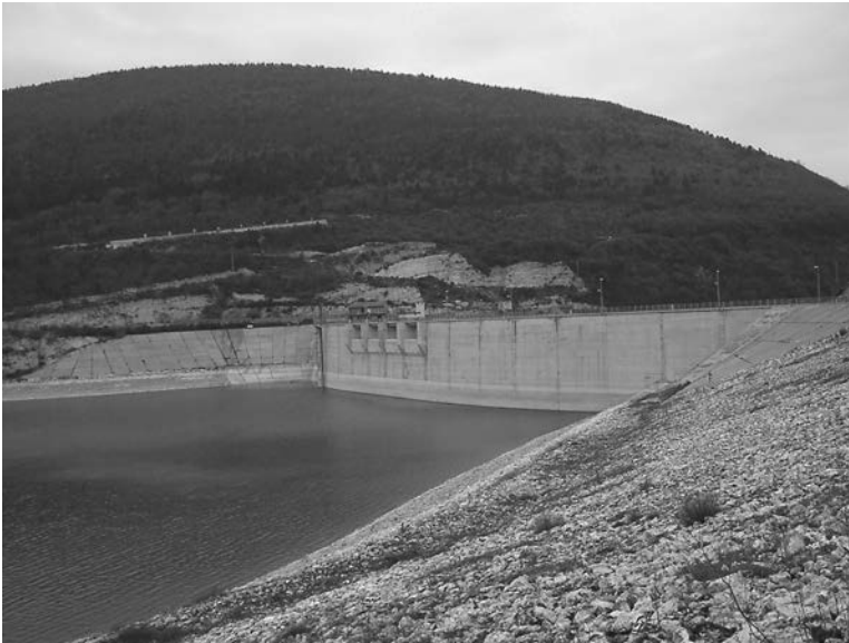
Figure 33.8 The Castreccioni dam (Italy), with linings on both banks, protected by concrete slabs or rockfill.
