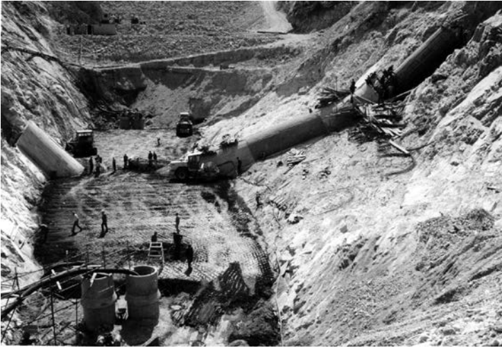
Figure 5.1 Kozyak dam (Macedonia) – early construction stage.
