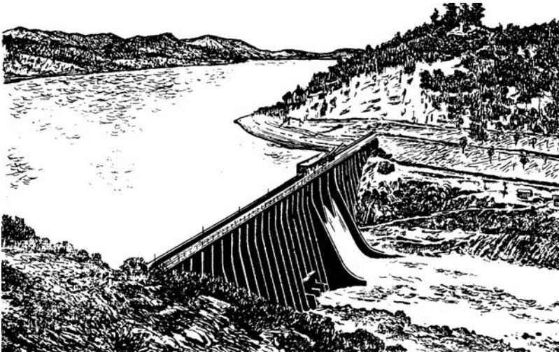
Figure 26.3 General view of the Stoney Gorge buttress dam (after Grishin et al., 1979).
