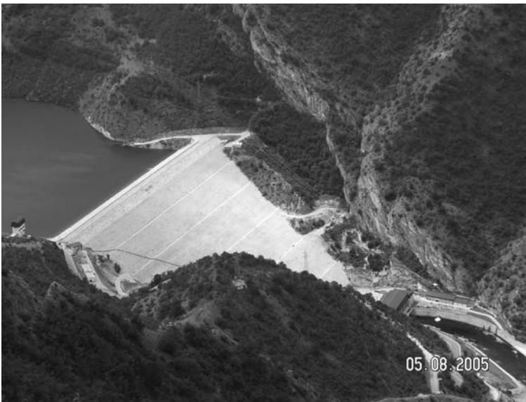
Figure 1.10 Kozyak dam, the highest in Macedonia.
