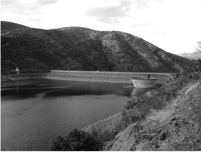
Figure 11.14 Tikvesh dam (Macedonia), with reservoir water level at 15 m below normal.
