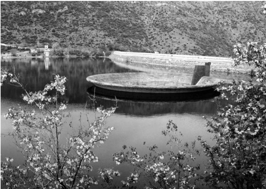
Figure 27.33 The shaft spillway of Tikvesh dam (Macedonia).
