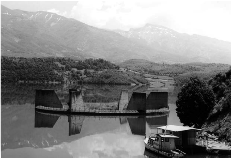
Figure 27.31 The shaft spillway at Shpilje dam (Macedonia).
