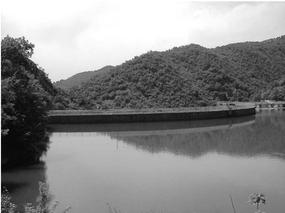
Figure 20.17 Gratche dam, with the spillway on the right side.
