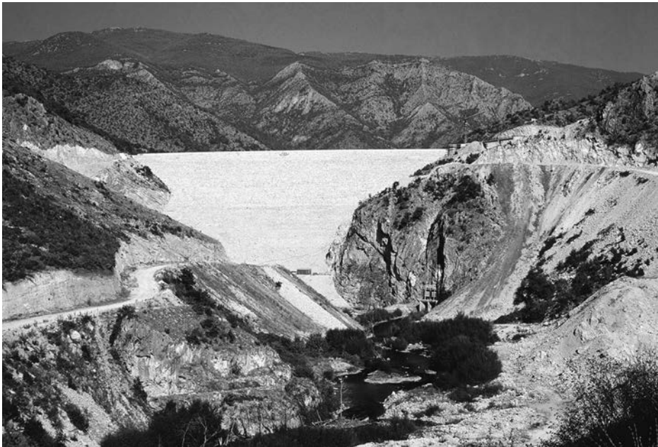
Figure 11.28 Upstream view of Kozyak dam before the dam closure in 2003.
