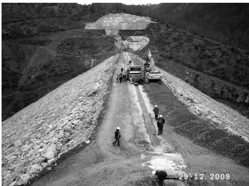
Figure 14.30 Knezhevo dam, placement of the last asphaltic concrete layer.
