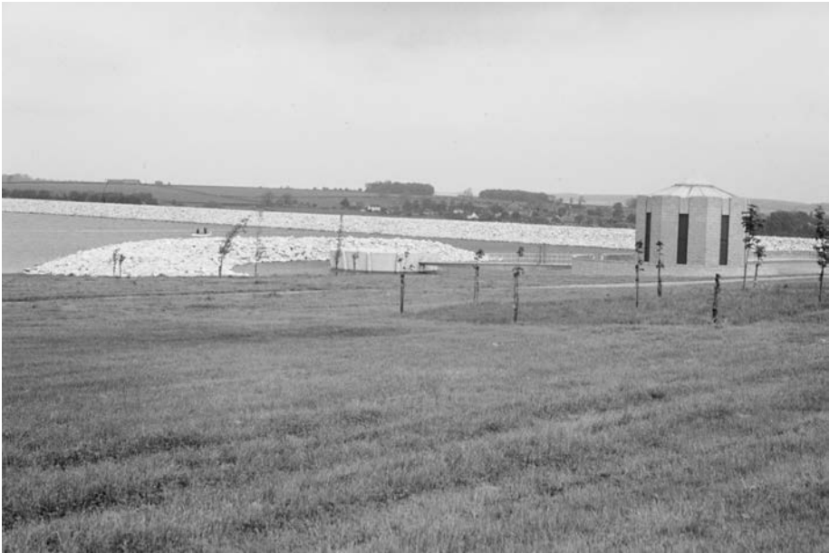
Figure 33.15 The Empingham dam, which forms the Rutland reservoir.
