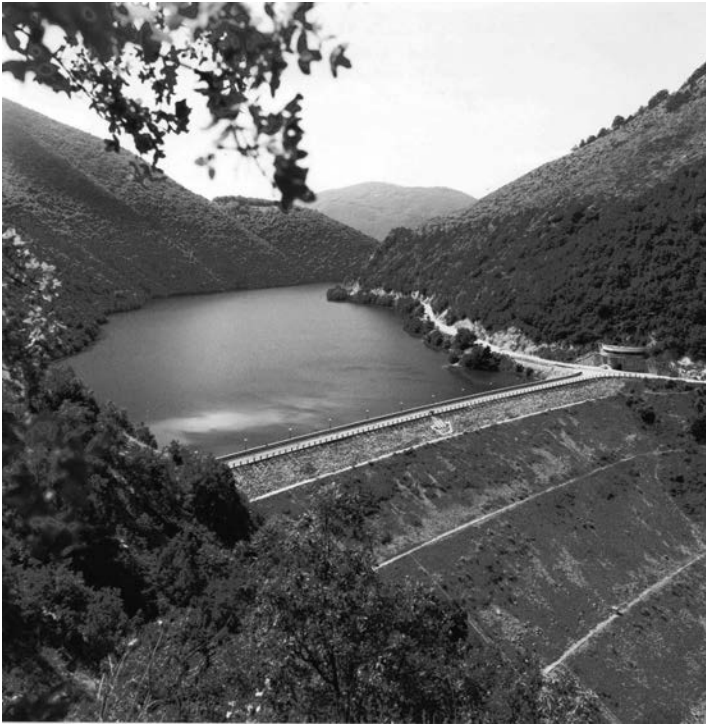
Figure 5.2 Globochica dam (Macedonia), some 20 years after its construction (service period).
