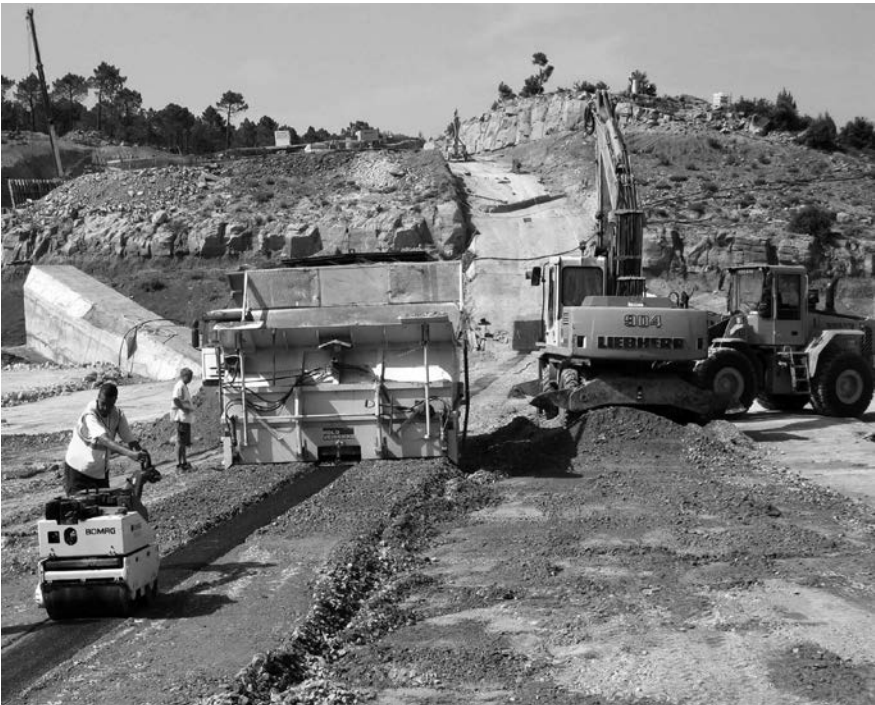
Figure 14.16 Compaction of the asphaltic concrete core by small vibratory roller.
