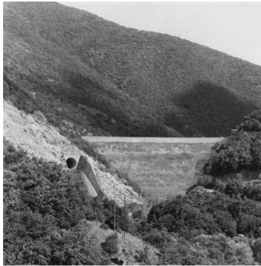
Figure 27.30 The exit of the outlet tunnel and the surface chute of Globochica dam (Macedonia).
