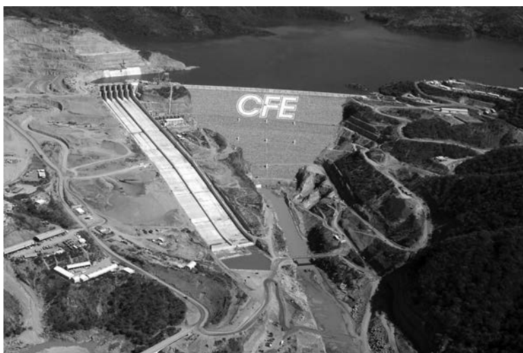
Figure 1.15 Spillway works at concrete faced rockfill dam El Cajón (Mexico), H = 189 m, commissioned 2006, with controlled spillway, chute channel and flip bucket (courtesy Mr. Humberto Marengo).
