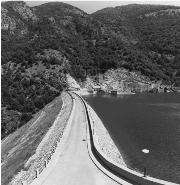
Figure 11.4 The crest of Globochica dam (Macedonia).
