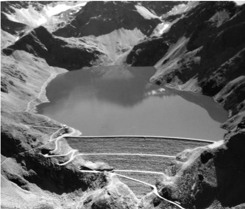
Figure 14.8 Finstertal dam and reservoir (Austria).
