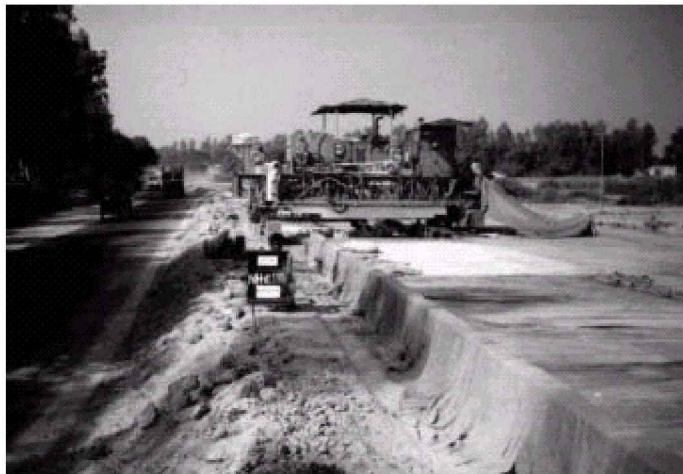
Figure 13.20 Concrete pavement construction by slip form paver (Courtesy: Mr. Pinaki Roychowdhury).
