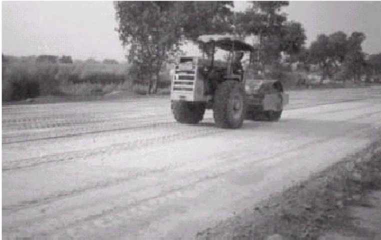
Figure 13.11 Compaction of subgrade on NH-25 (Courtesy: NHAI and ICT Ltd., Kanpur).
