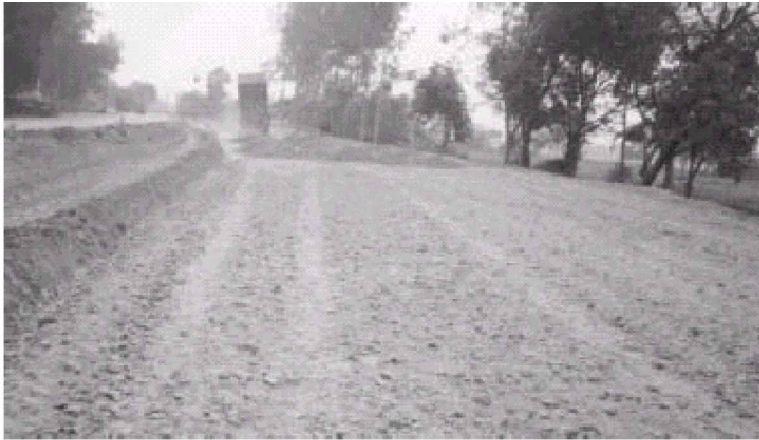
Figure 13.12 Dumping and spread of GSB (Courtesy: NHAI and ICT Ltd., Kanpur).
