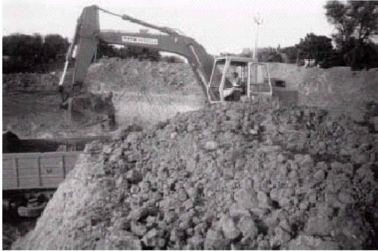
Figure 13.10 Earth excavation in progress (Courtesy: Mr. Pinaki Roychowdhury).
