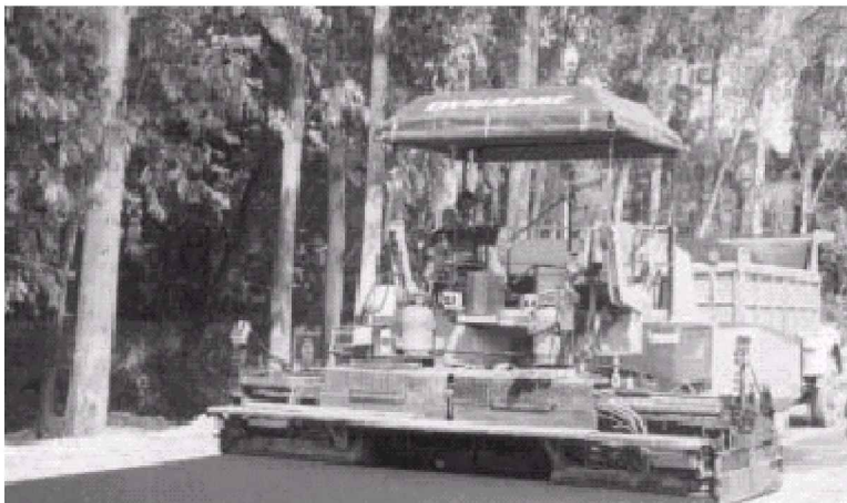
Figure 13.8 A paver finisher in operation (Courtesy: Lucknow, NHAI).
