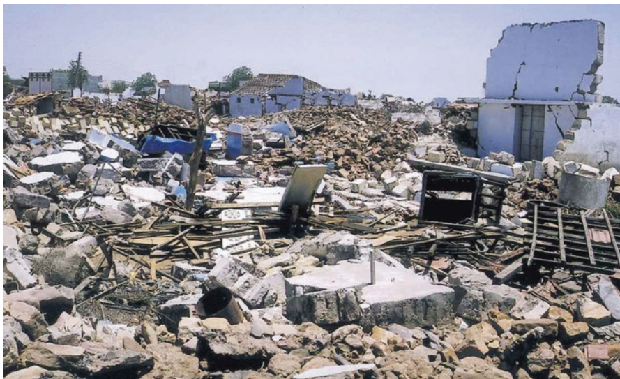
Fig. 1.4 Damage during 2001 Bhuj earthquake
