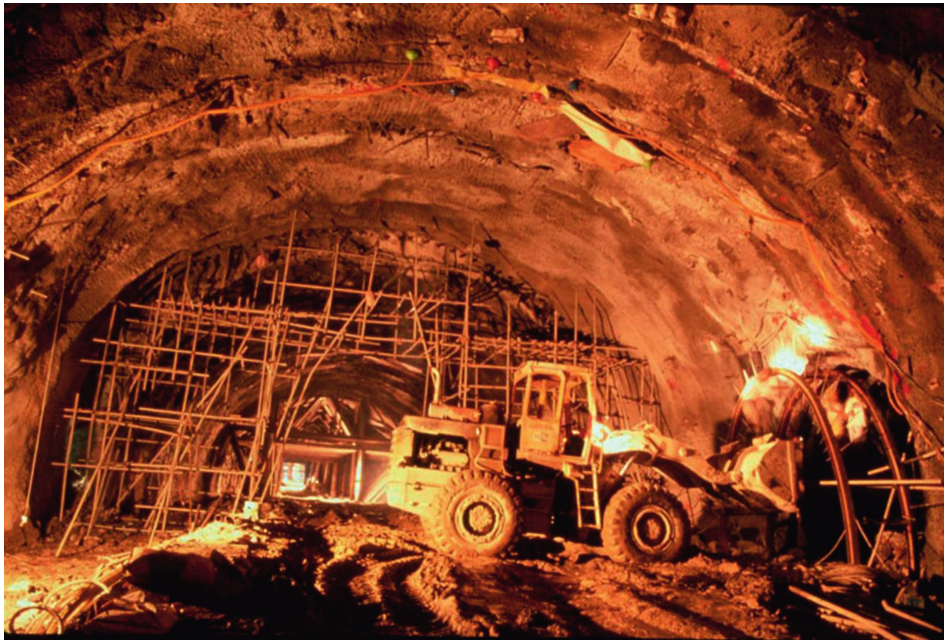
Figure 19.3 Emergency support works for large tunnel collapse.
