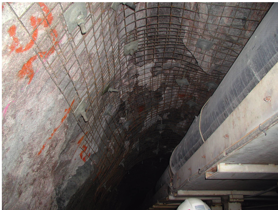
Figure 7.9 Continuous overstepping along small diameter TBM tunnels.
