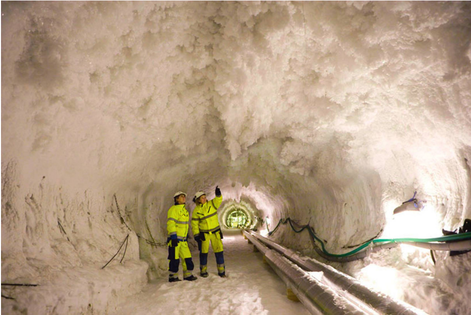
Figure 9.9 Ground freezing at Hallandsås.
