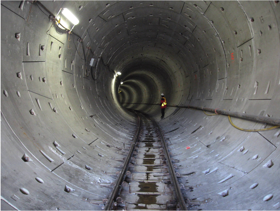
Figure 19.9 Pre-cast concrete lining – Canada Line.
