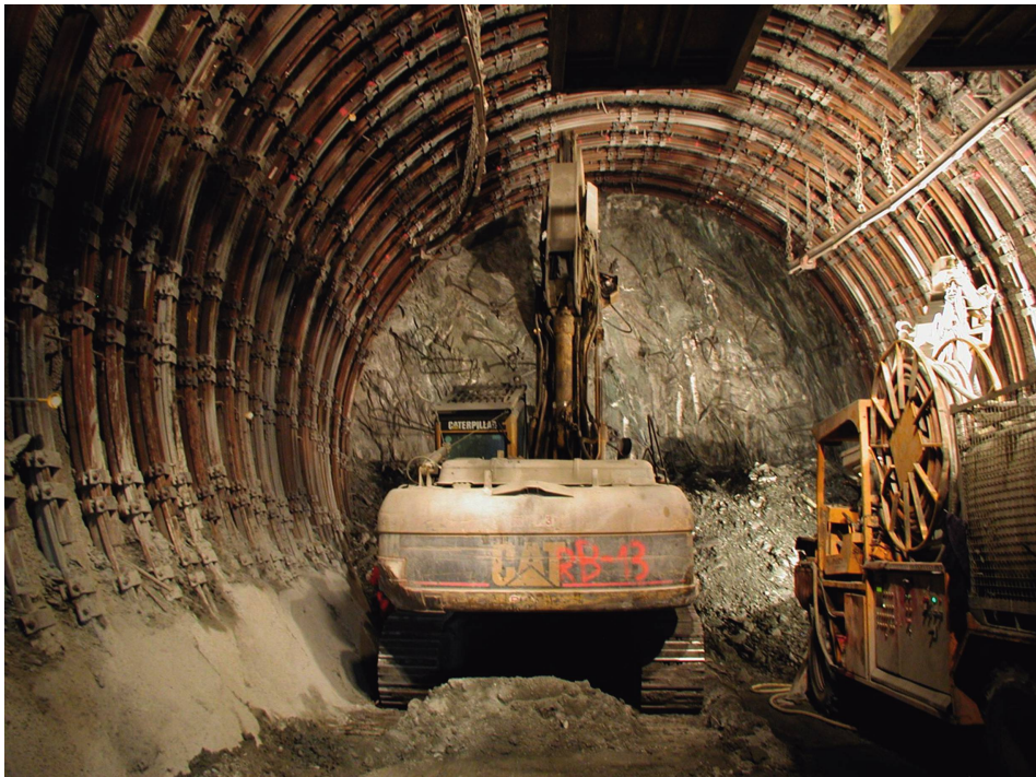
Figure 9.4 Yielding steel ribs for squeezing ground.
