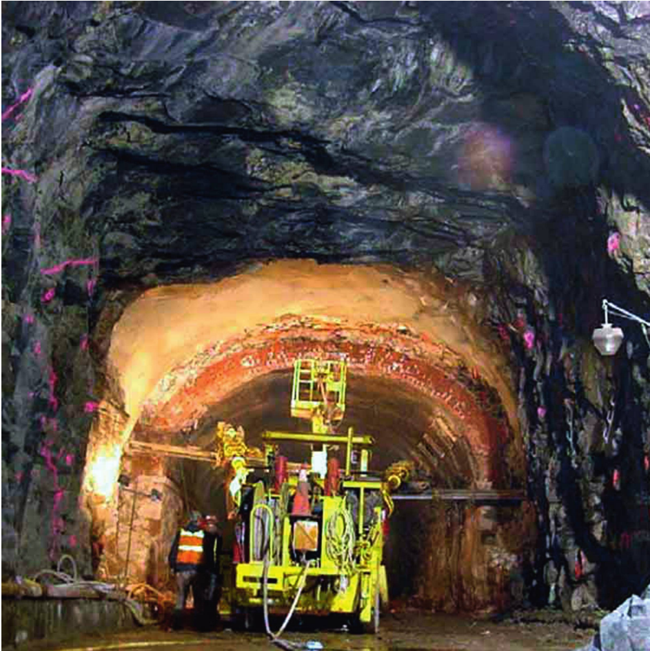
Figure 18.1 Renovation of Weehawken Rail Tunnel.
