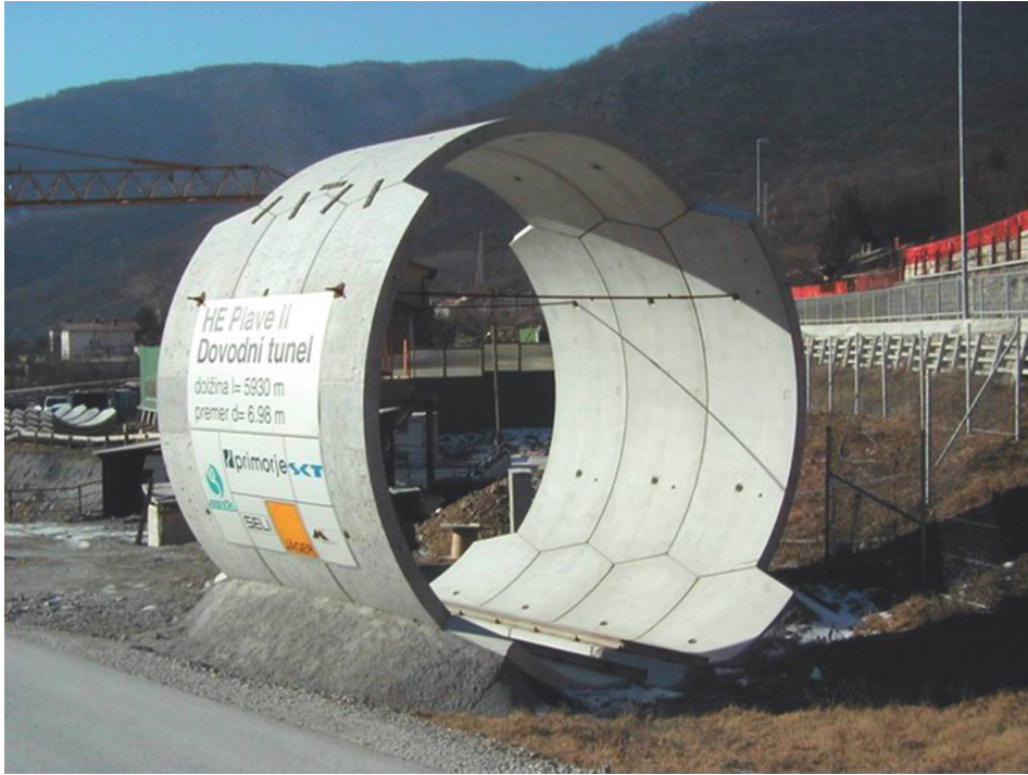
Figure 10.4 Pre-cast concrete segmental lining for final lining in a hydropower tunnel.
