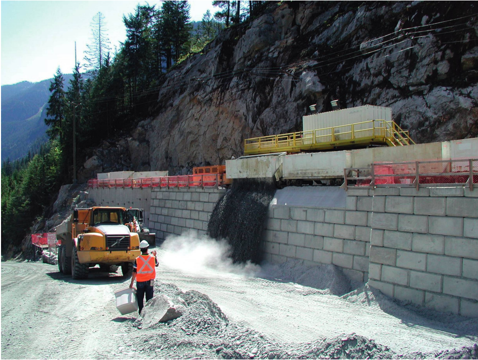
Figure 11.5 Tipping station for spoil disposal.
