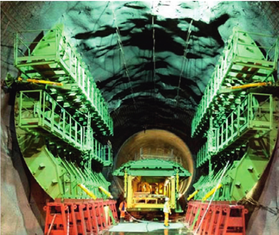
Figure 10.3 Large diameter traveling collapsible formwork.
