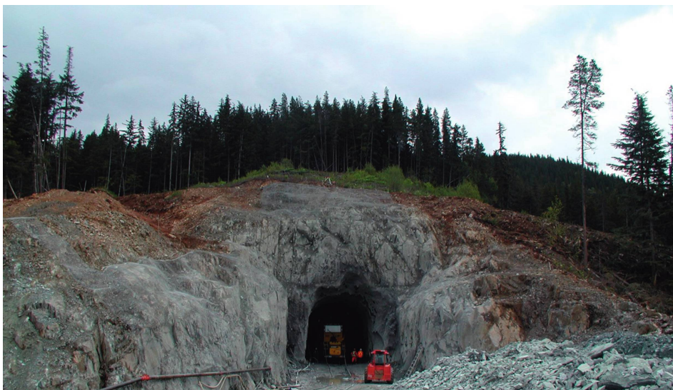
Figure 19.11 Tunnel portal location along small ridge versus gully location.
