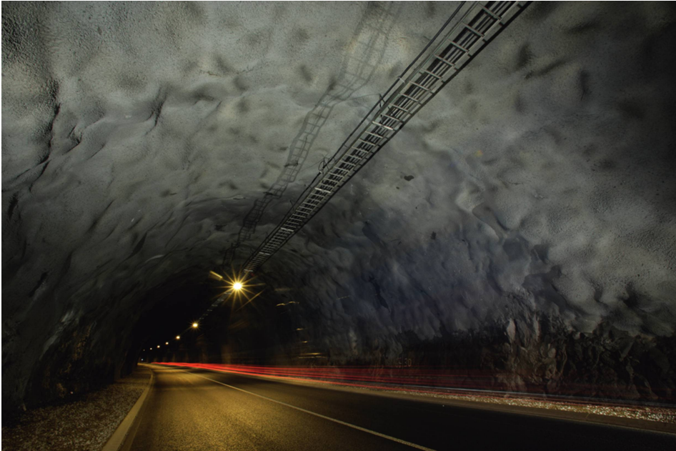
Figure 10.6 Spray-on membrane for waterproofing of road tunnel.
