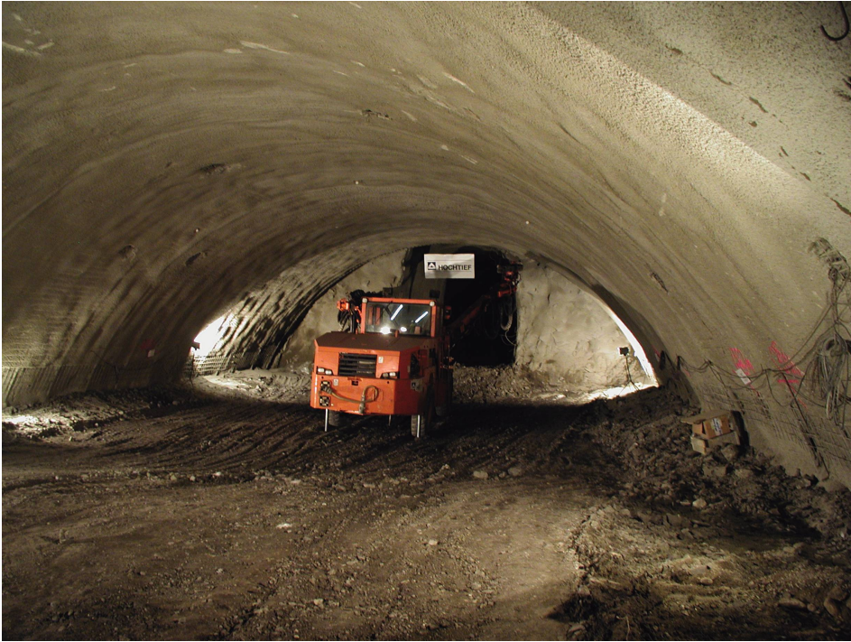
Figure 12.7 Pilot tunnel.
