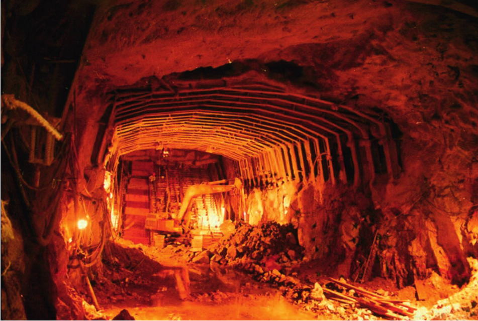
Figure 19.2 Steel sets for shallow pedestrian tunnel support.
