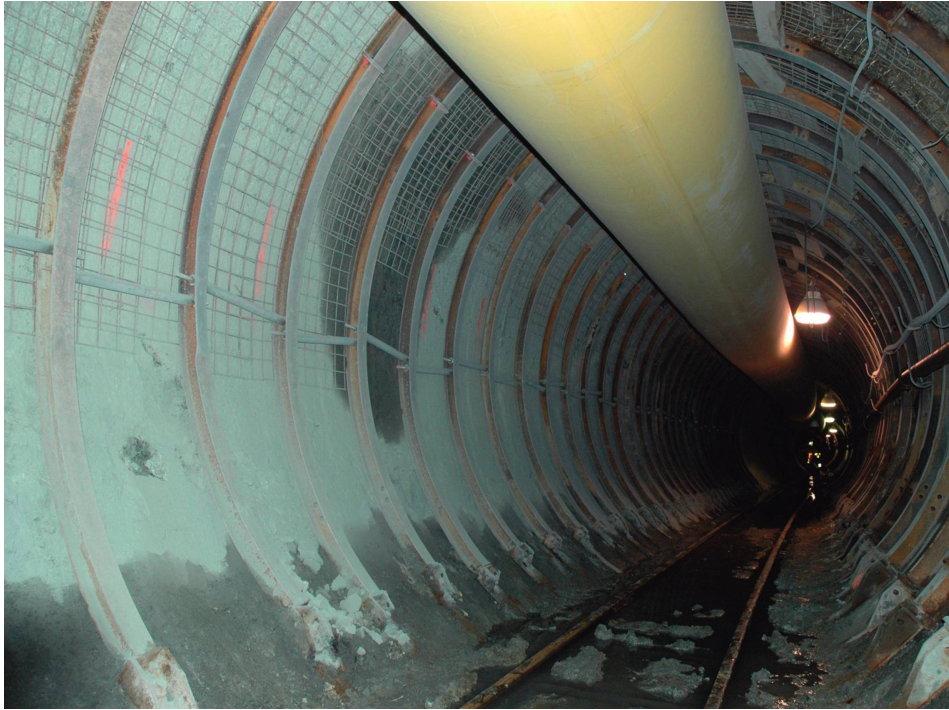
Figure 19.10 TBM tunnel support for long geological fault.
