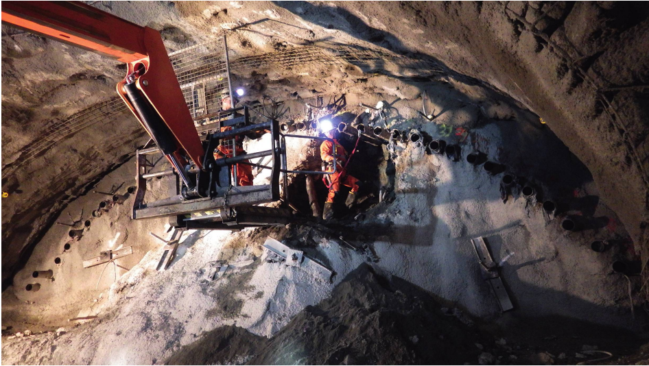
Figure 12.2 Canopy tube installation through paleochannel sediments.
