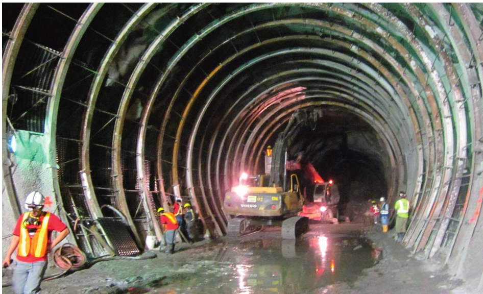
Figure 18.2 Repair of hydropower tunnel.
