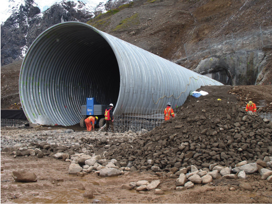
Figure 12.1 Structural portal canopy for avalanche risk.
