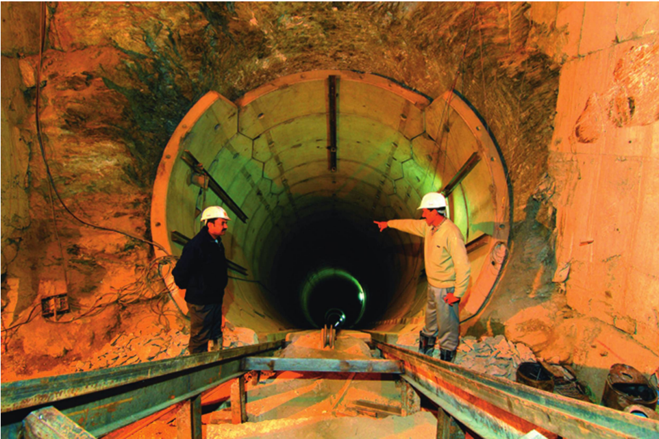
Figure 8.11 Inclined pressure shafts with pre-cast concrete linings at Parabati.
