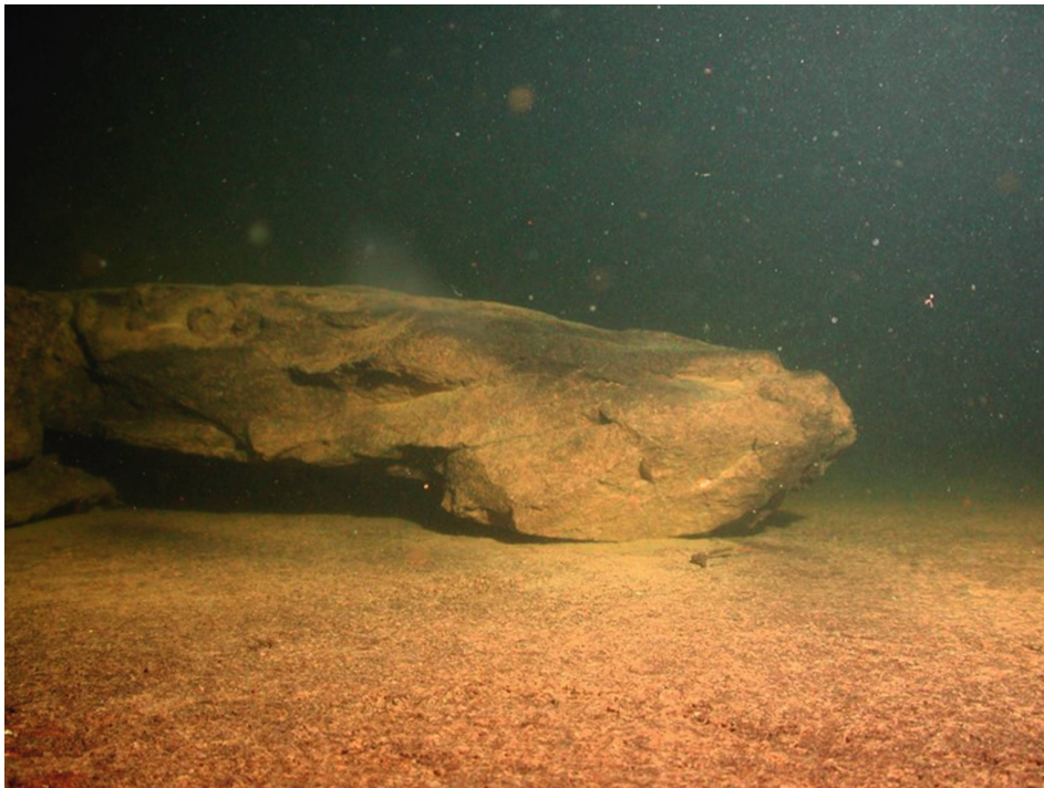
Figure 17.1 High resolution photograph from unwatered tunnel inspection.
