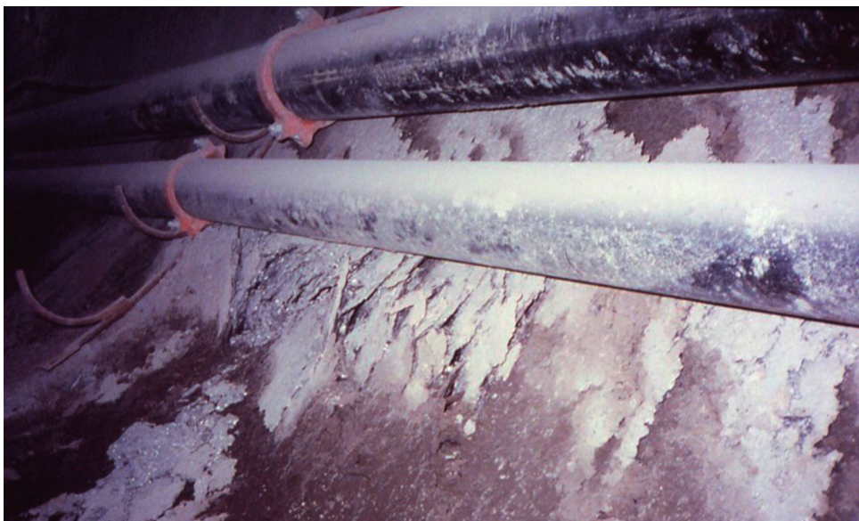
Figure 19.1 Deterioration of highly amygdaloidal basalts.
