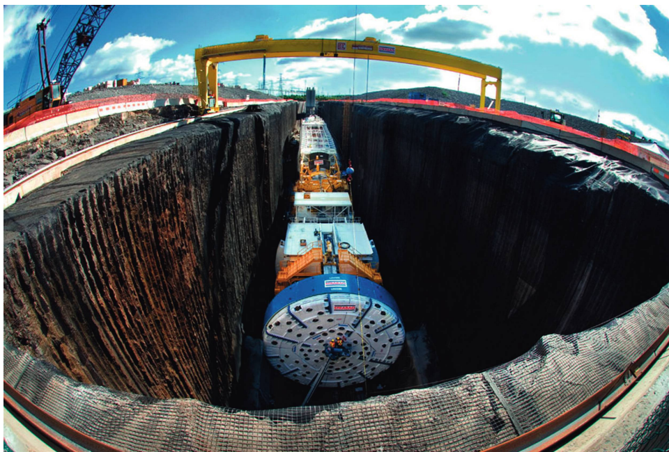
Figure 8.6 Open gripper TBM.
