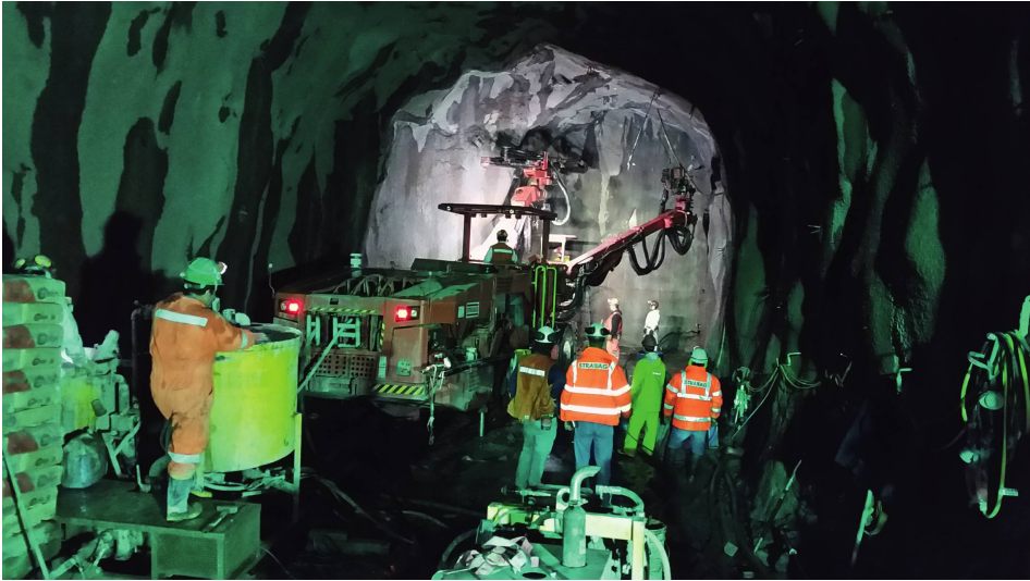
Figure 12.6 Pre-excitation grouting activities.
