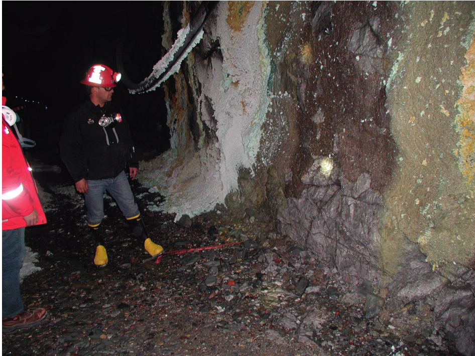
Figure 9.6 Softening of shotcrete from direct contact of acidic groundwater.
