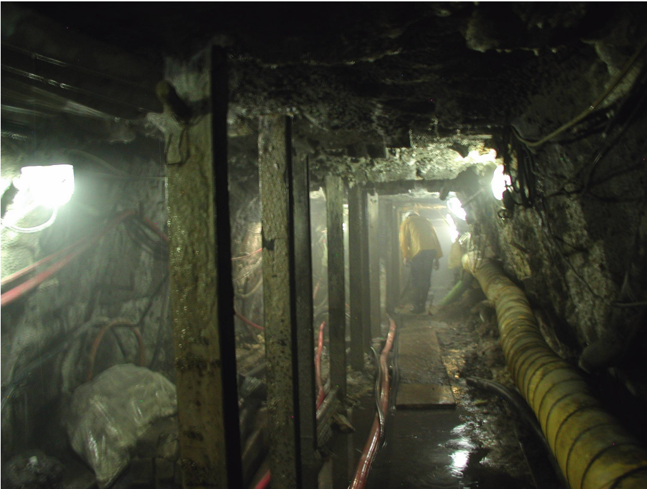
Figure 12.3 Bypass tunnel over TBM.
