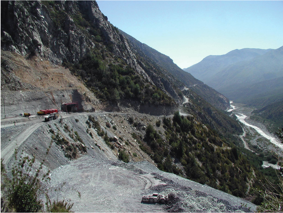
Figure 11.4 Tunnel spoil site.
