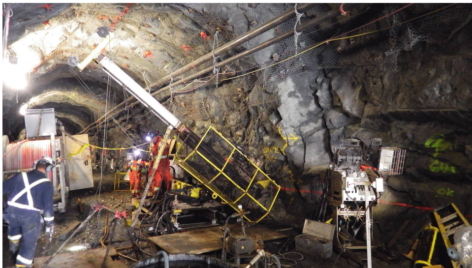
Figure 4.8 Hydraulic jacking testing.
