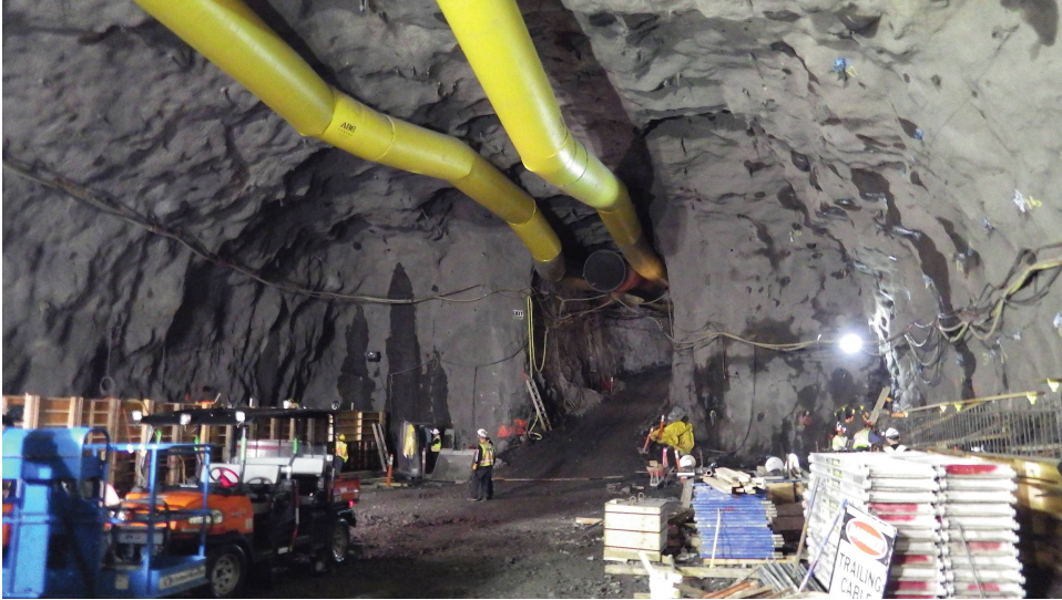
Figure 8.13 Cavern excavation for hydropower powerhouse.
