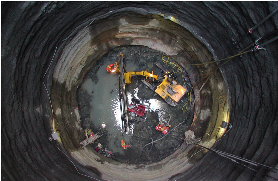
Figure 8.12 Shaft excavation.
