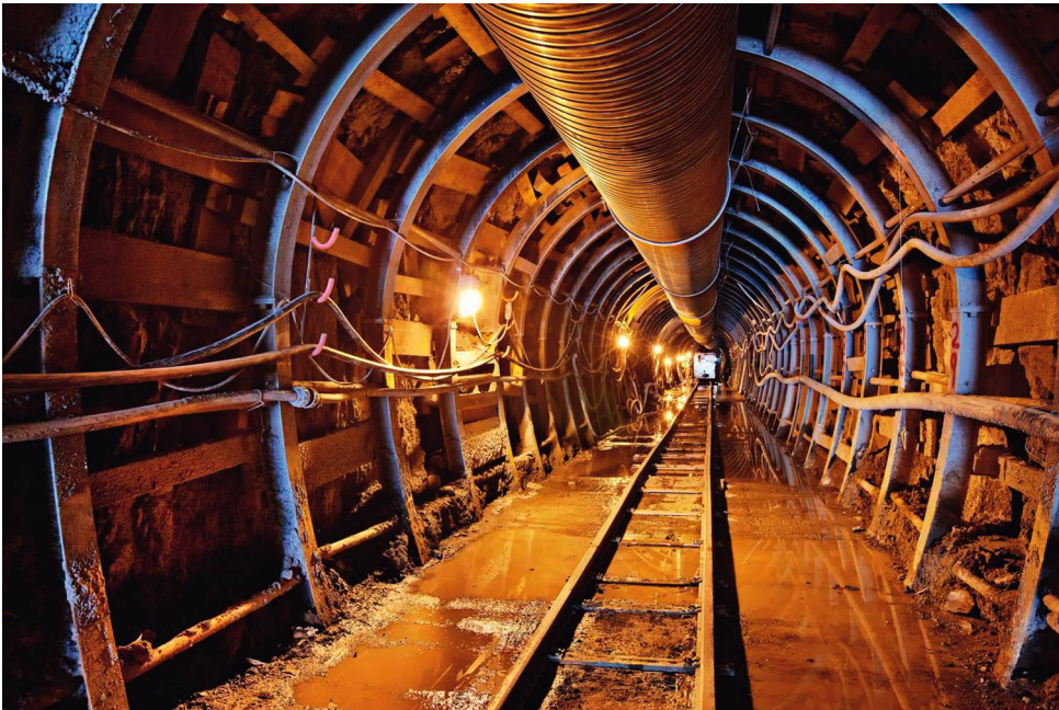
Figure 7.14 Steel ribs supports for continuous squeezing conditions.
