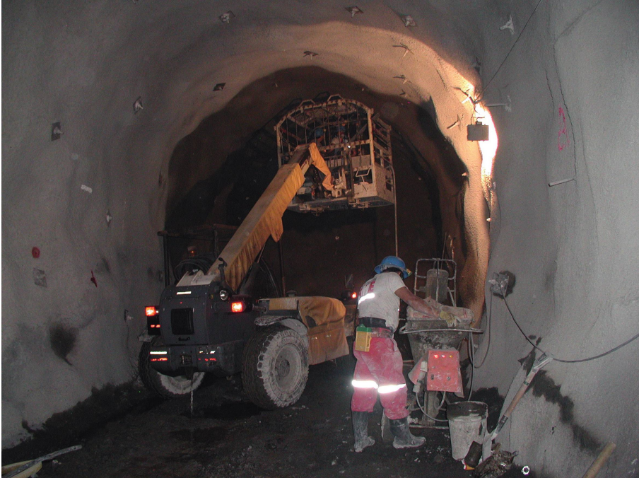
Figure 9.2 Protection canopy for rock bolt installation.
