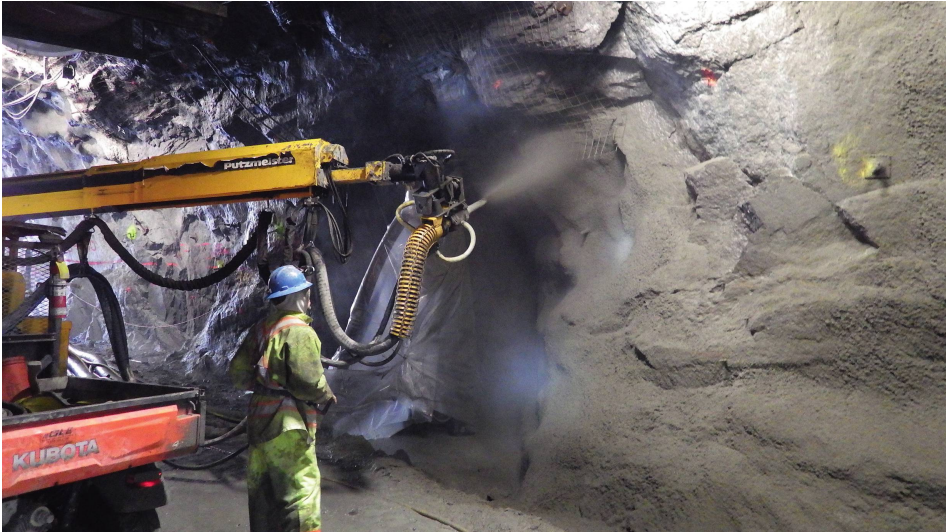
Figure 10.2 Shotcreting for final lining in a hydropower tunnel.
