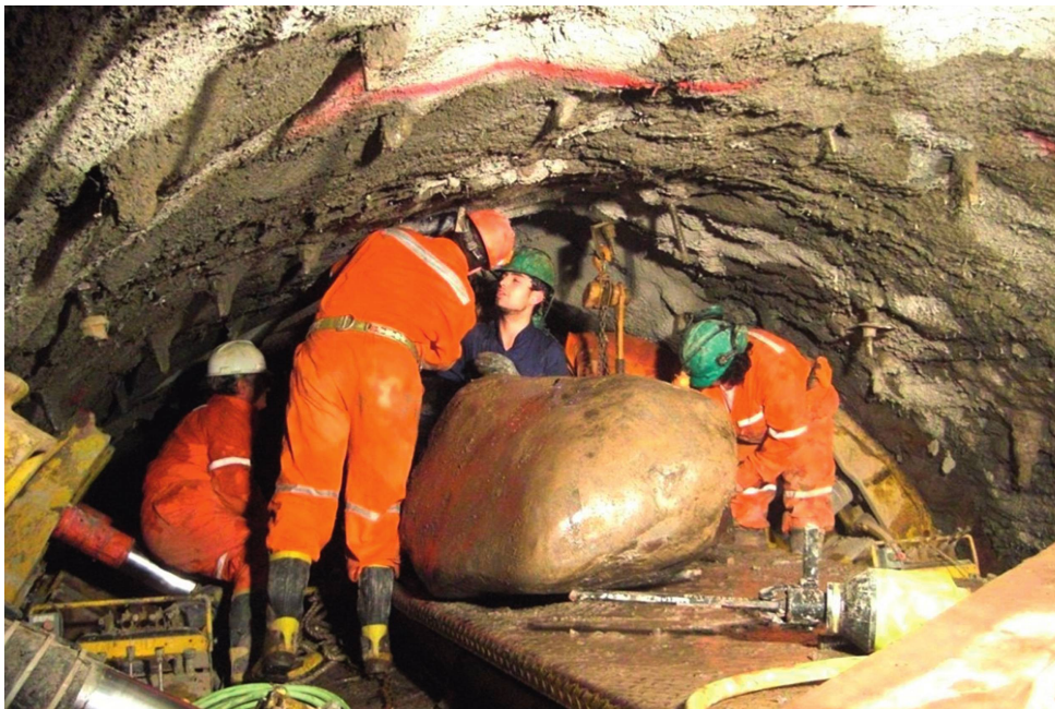
Figure 19.13 Open gripper TBM excavated tunnel with boulders.
