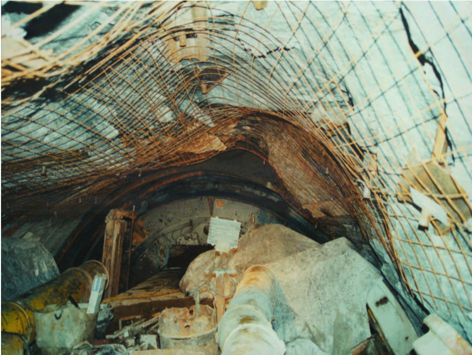
Figure 19.5 Extreme oversteering of rock at 1700 m depth.
