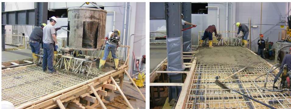
Deck Pour (08 February 2012) – GFRP reinforced deck (Truck C)
