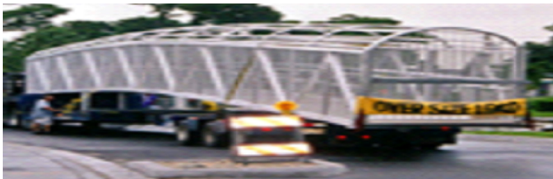
A Gator aluminum bridge being transported for erection
