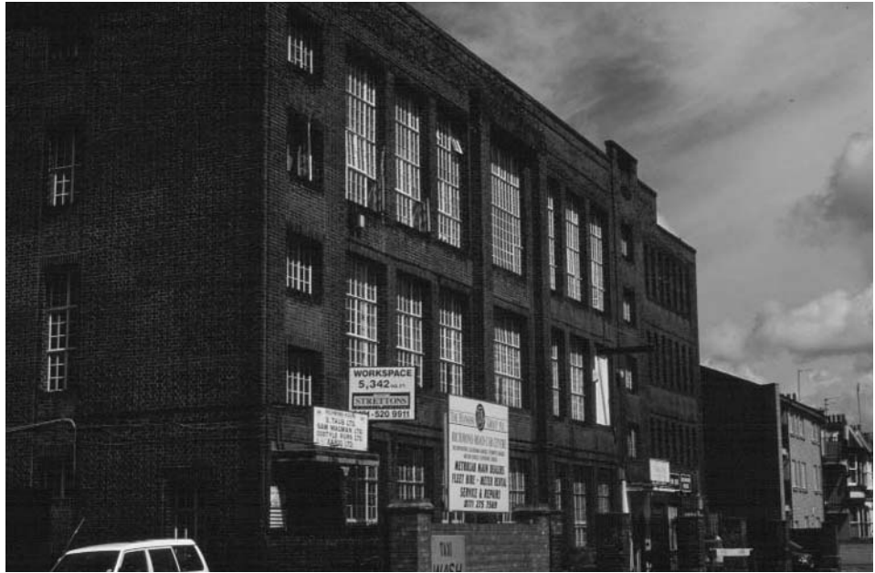
Richmond House in Hackney, London: a former garage now headquarters of MOMART and reused by the association SPACE for artists' studios – photo: Jesús Pedro Lorente
