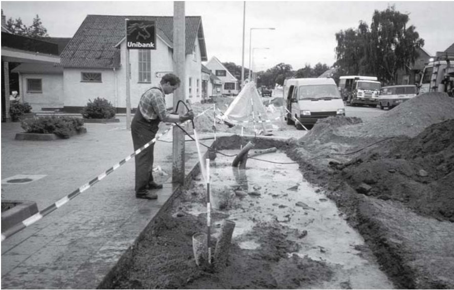
Fig. 11.8. Watermixing of the soil and stone during installation ( photo : P. Kristoffersen)
