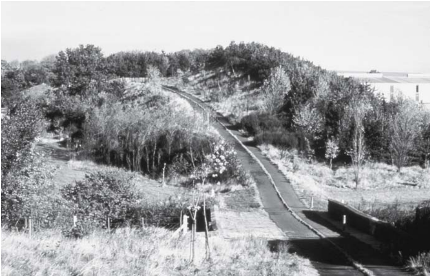
Fig. 18.5. A footpath/cycleway in Telford, threading its way along an urban forestry “green link” connecting areas of housing, recreation and employment ( photo: A. Simson )
