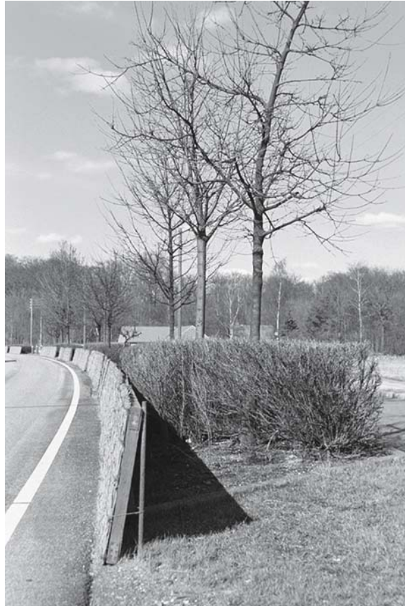
Fig. 11.6. Physical protection measures against de-icing agents in Copen- hagen (photo: T. B. Randrup)
