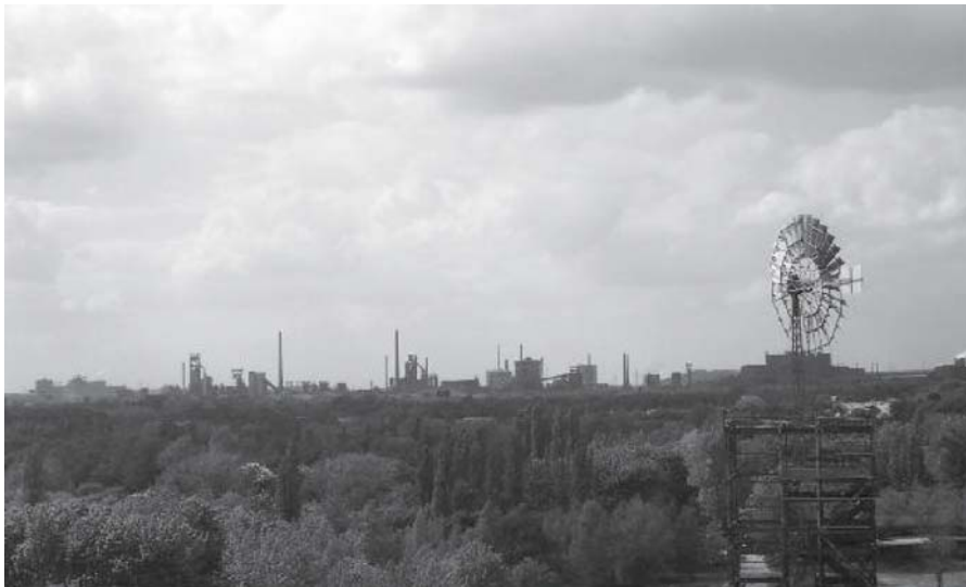
Fig. 18.7. An overview of the relationship between the regenerating urban forest and the relic industrial structures in the Emscher Park (photo: B. Schrader)
