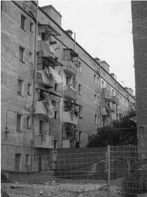
Plate 8.1 Run-down housing adjacent to new hotel developments, Cultural Forum 2004 site, Barcelona
