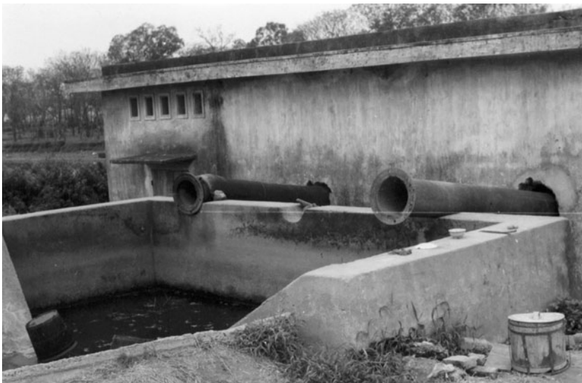
Fig. 7.2. A disused wastewater pumping station.
