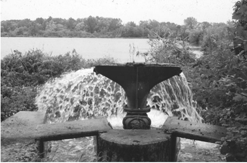
Fig. 4.3. A sprinkler introducing secondary treated wastewater diluted with river water into a wastewater-fed fishpond in Munich, Germany.
