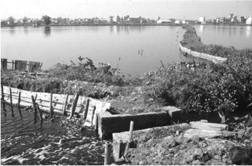
Fig. 4.1. Wastewater being pumped into a wastewater-fed fishpond in Hanoi.
