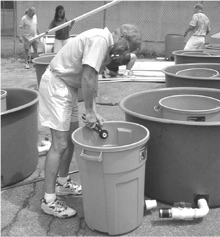
Fig. 16.2. A teacher works on fitting a bulkhead for the outflow of the sump during the Aquaculture in Action workshop.
