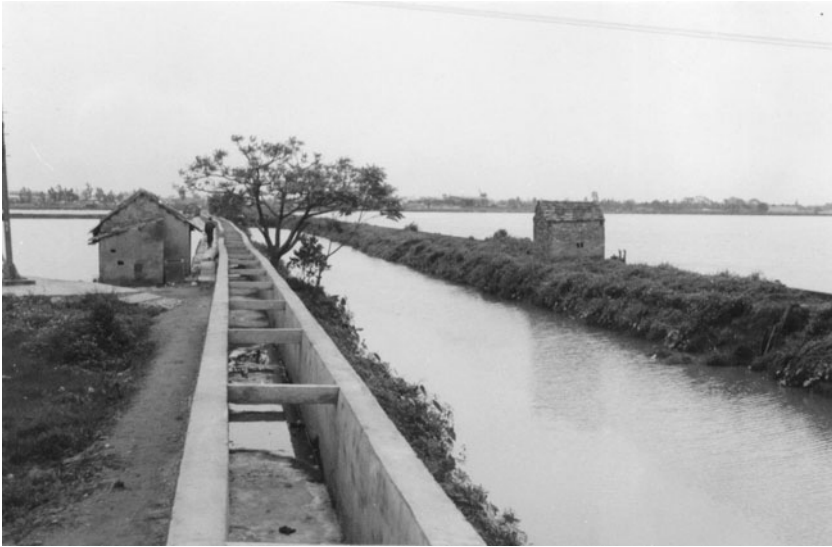
Fig. 7.3. A disused wastewater distribution channel with fish-only production system on each side.
