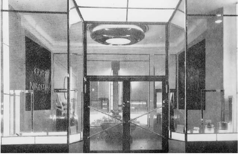
Figure 53. Stainless steel frames for display window of Krupp-Nirosta store, Düsseldorf, designed by Paul Mählberg (1928).
