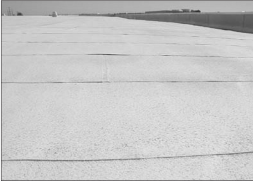
Figure 5.5 A cementitious cool roof coating
