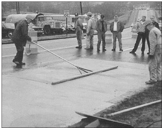
Figure 6.11 Ultra-thin white-topping being applied over an existing asphalt road
