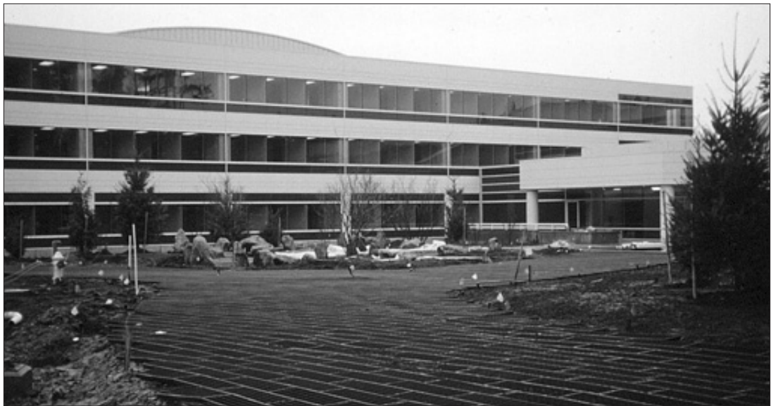
Figure 6.19 Porous pavers filled with soil and grass used as emergency fire lanes around buildings at the Microsoft campus in Washington state
