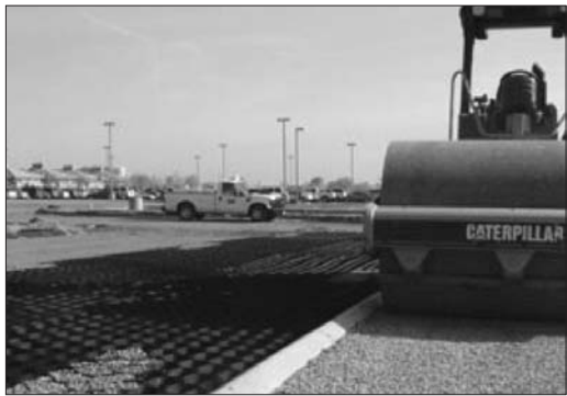
Figure 6.18 Porous pavers being filled with aggregate for use in a parking lot at the University of California Merced Campus
