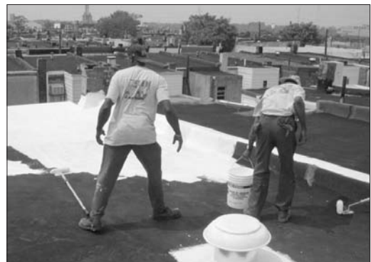
Figure 9.10 A cool coating being applied to the black roof of a rowhouse in Philadelphia
