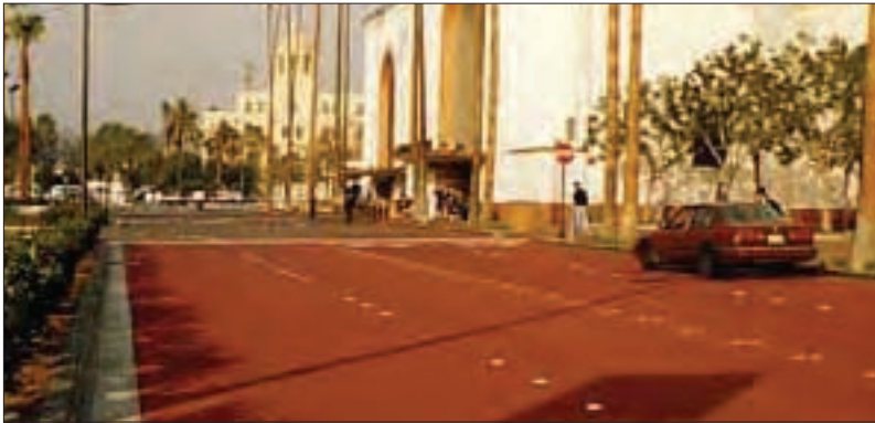
Plate 19 Roadway outside of Union Station in Los Angeles surfaced with a coloured asphalt emulsion sealcoat
