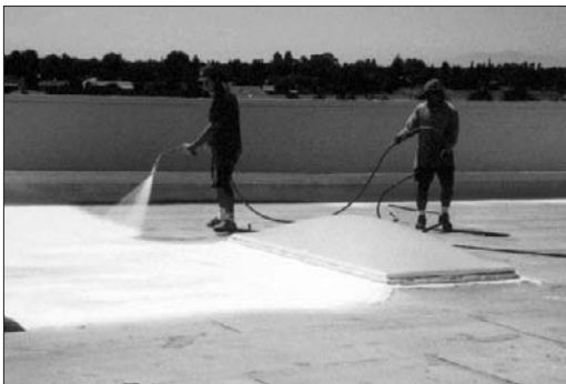
Figure 5.4 Application of an elastomeric cool roof coating
