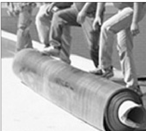
Figure 5.7 A roll of standard black EPDM single-ply roofing
