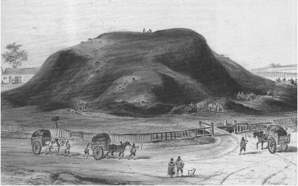
Smith's Dust Heap, end of Gray's Inn Road, King's Cross (courtesy of London Metropolitan Archives)
