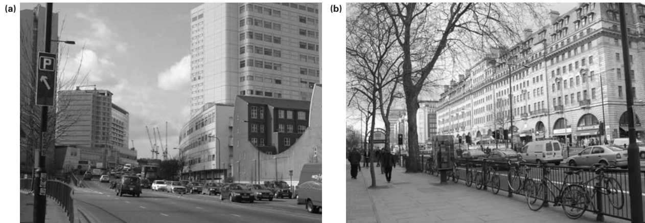
2.3 • Denial of the traditional arterial street. Under the current system, traditional arterial streets such as Marylebone Road (Figure 2.2) are not recognised as such; only the separate roles of (a) primary distributor or (b) access road (frontage street).
