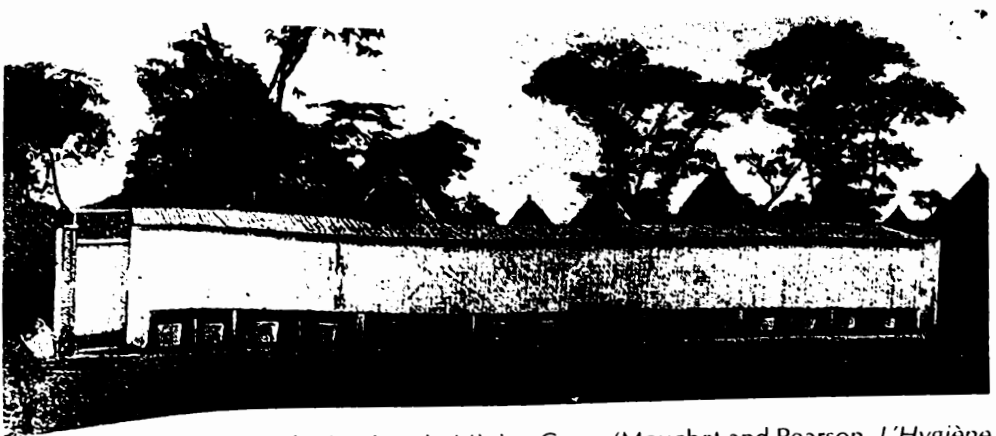
Photo 10.1. Building for Latrines in Mining Camp (Mouchet and Pearson, L'Hygiène pratique ).
