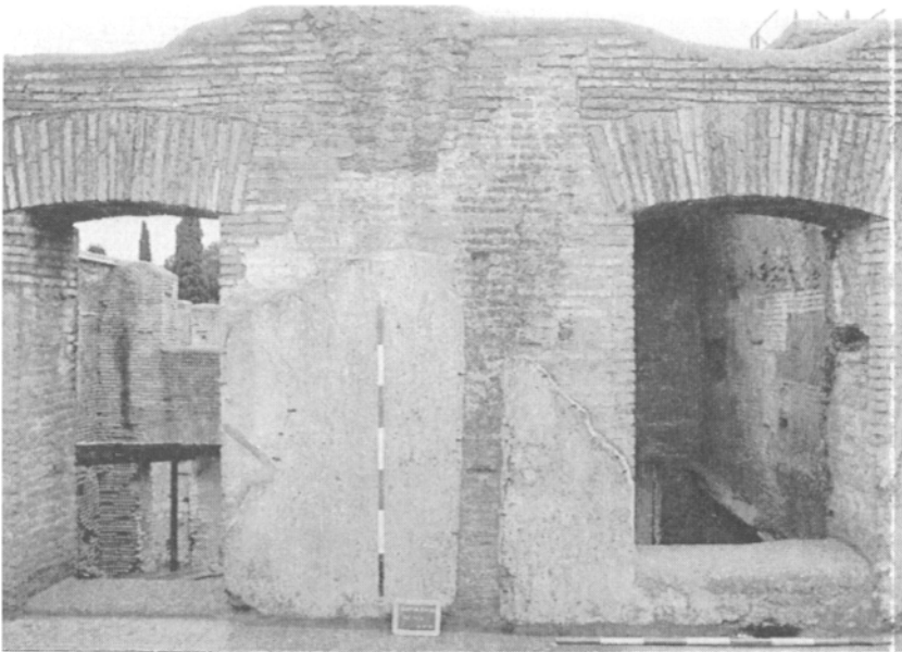
Figure 5.7 Marks of curtain wall in Rm 129.
