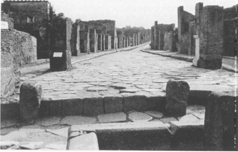
Figure 3.4 Via dell'Abbondanza, viewed from the junction with the Stabiana, looking towards the fo rum. Note the sharp drop in road level.
