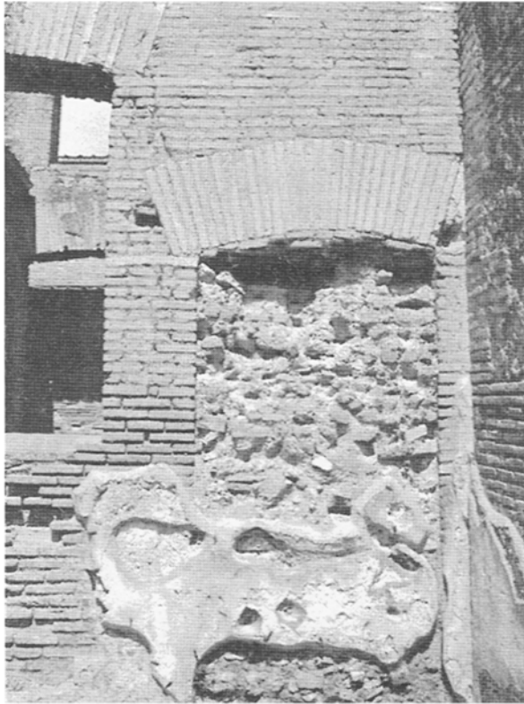
Figure 5.5 RMs 24/25, blocked doorway.
