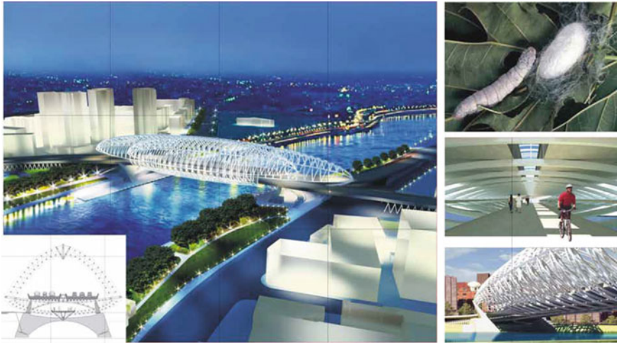
Fig. 6 Bridge over the river Hai He in the city of Tianjin, China. Bionic references taken from a silkworm (source Cervera et al. 2011)
