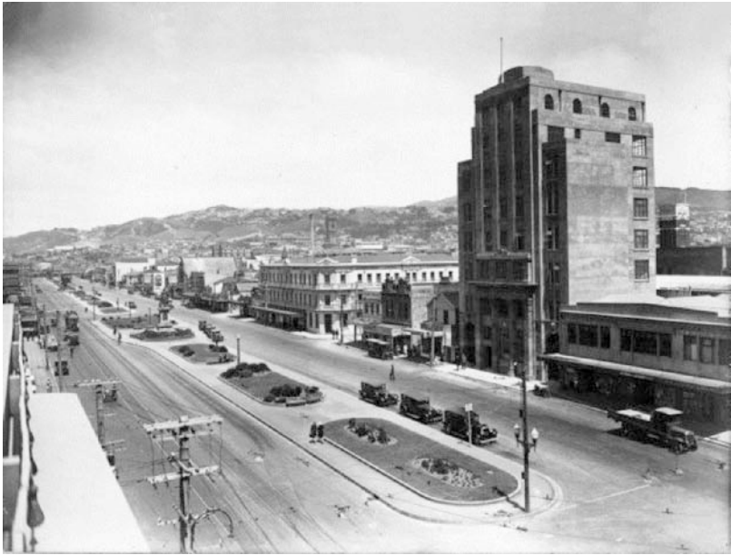
Figure 3.3 Cambridge and Kent Terraces, Wellington, 1931. The Wellington East Post Office Building is shown here completed – it tended to dwarf low-rise buildings around it, such as the Cambridge Hotel to the left of it
