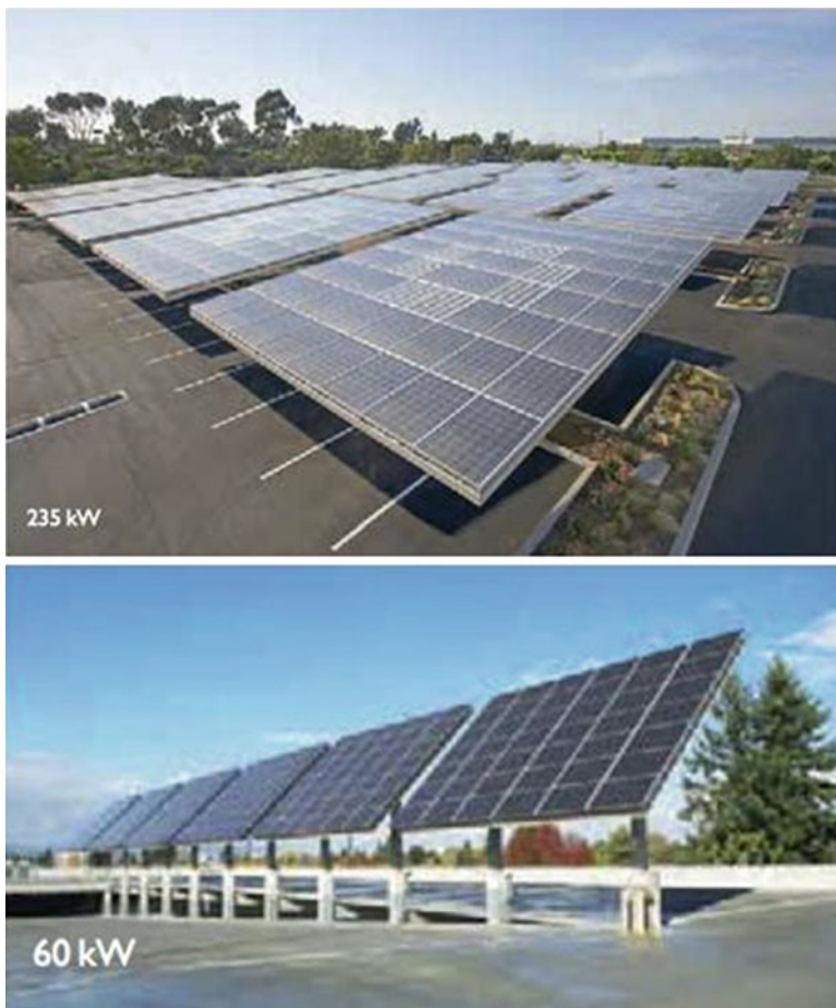
Fig. 12.5 Solar charging stations of different scales of electric vehicles (Created by the Waterloo Institute for Sustainable Energy [4])
