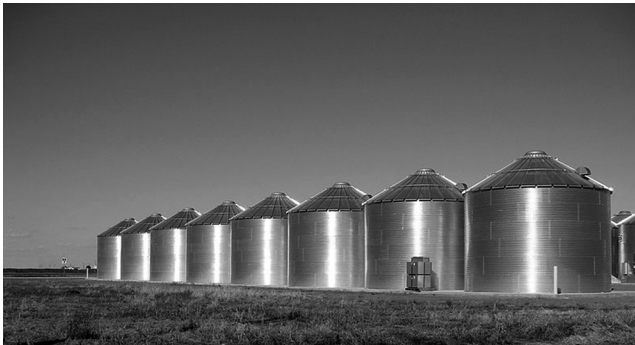
Figure 7.3 Sequential and independent operations within emergency management often create functional connection components that are ultimately disconnected such as commercial storage silos. (From Public Domain/Llano Estacado. With permission.)
