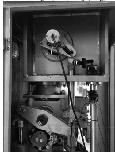
(b) Operating mechanism of LW30-252 model SF6 high-voltage CB.
