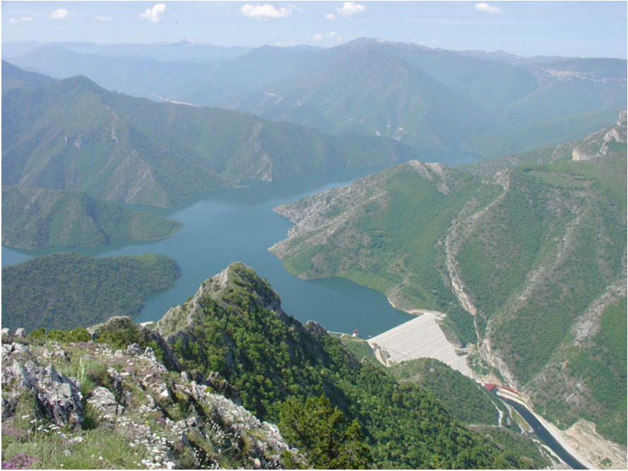
Fig. 15.10 The dam of the Kozjak reservoir
