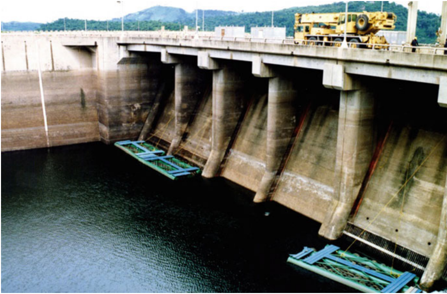
Fig. 2.2 Reduced water level at Akosombo (July 1998)
