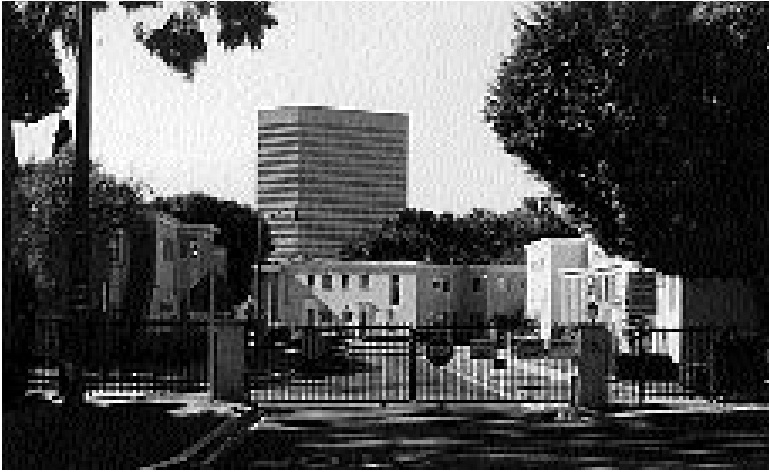
Gates added in 1990 to Park Labrea, Los Angeles. Originally designed by Leonard Schultze & Son and E. T. Heitschmidt for Metropolitan Life Housing Development, 1941–1948
