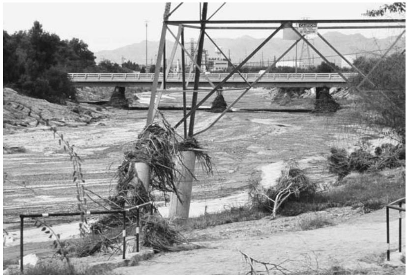
Heavy rains triggered by an El Niño event led to flooding in Rillito Creek, Tucson, Arizona, that caused substantial damage in October 1983. (USGS)
