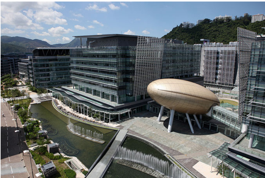
Fig. 2.11 Hong Kong Science and Technology Park
