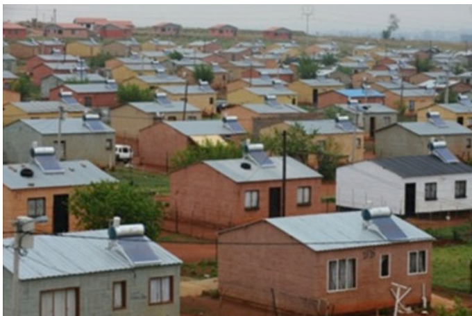
Fig. 16.22 Solar geysers installation project
