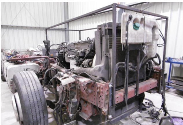
Fig. 6 Dismantling of the truck
