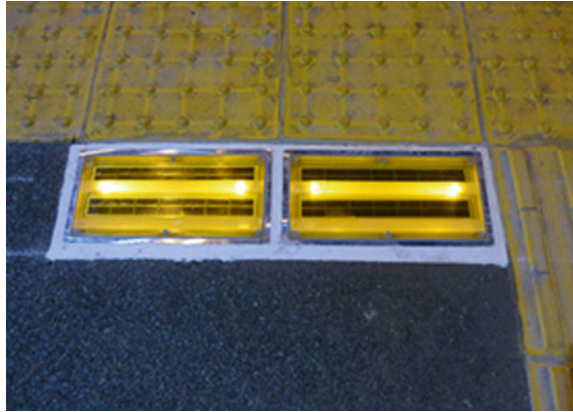
Fig. 2 LED block installed at crosswalk entrance
