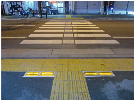
Fig. 3 The LED block was installed at an actual crosswalk entrance
