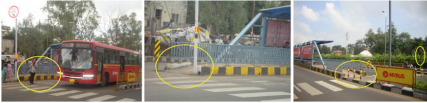
Fig. 1 Above photographs showing manually operated pedestrian movement on zebra crossing and condition of newly constructed curb and ramp showing poor quality (near Habibganj railway crossing, Bhopal). Images showing encircled issues like installed pedestrian crossing light (not working) at Misrod area. Source Author
