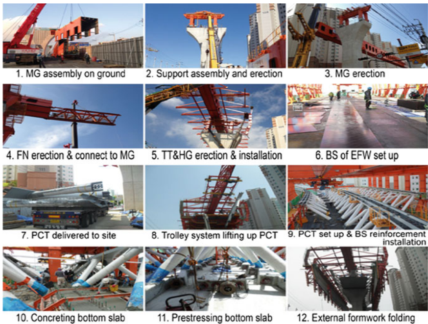
Fig. 4 Assembling and erecting sequence of the MSS and PCT
