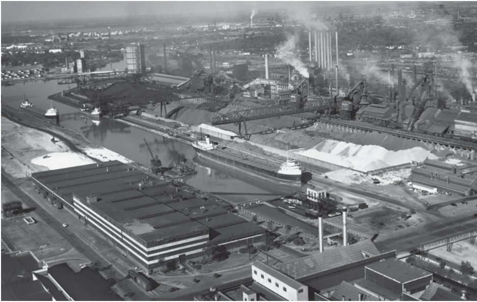
FIGURE 5.12 The classical principles of industrial location theory are evidenced in the river valley and railroad site of Bethlehem Steel Corporation's plant at Bethlehem, Pennsylvania. This huge plant, which extends for nearly 8 kilometers along the south bank of the Lehigh River, converts raw materials—Appalachian coking coal and Minnesota iron ore—into structural shapes, large open-die and closed-die forgings, forged steel rolls, cast steel and iron rolls, ingot molds, and steel, iron, and brass castings. The main market for the steel products is the American Manufacturing Belt with its abundance of metal-using industries.
