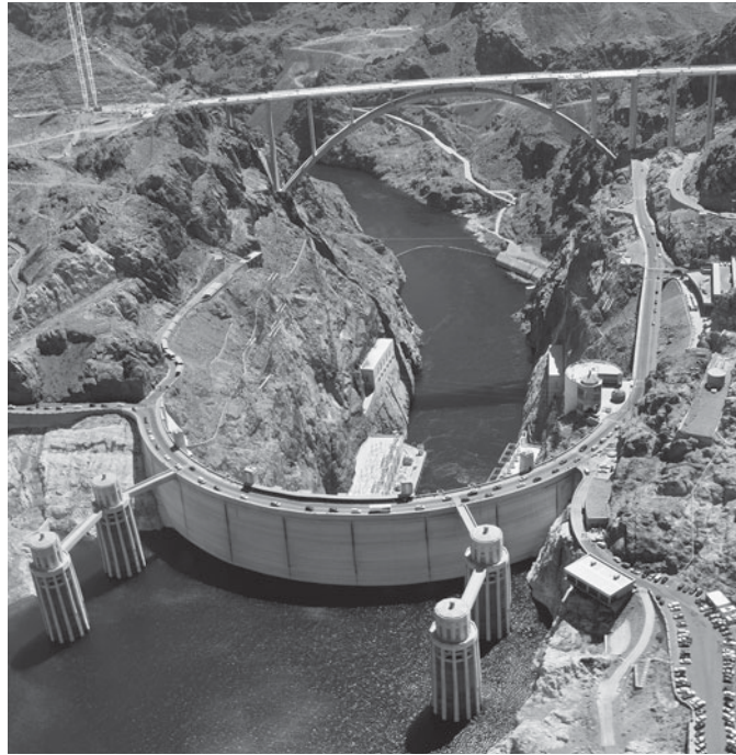
FIGURE 5.18 Hydroelectric dams, such as the Hoover Dam pictured here, are large, expensive projects that illustrate the state's role in the construction and maintenance of the infrastructure.
