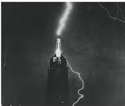
23.17 The metal mast at the top of the Empire State Building acts as a lightning rod. It is struck by lightning as many as 500 times each year.
